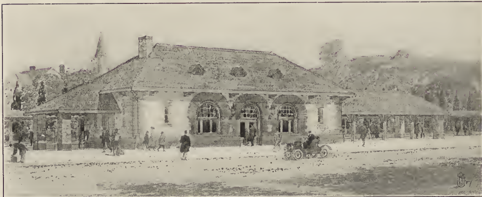
FIG. 4. STATION AT WEST FARMS.
