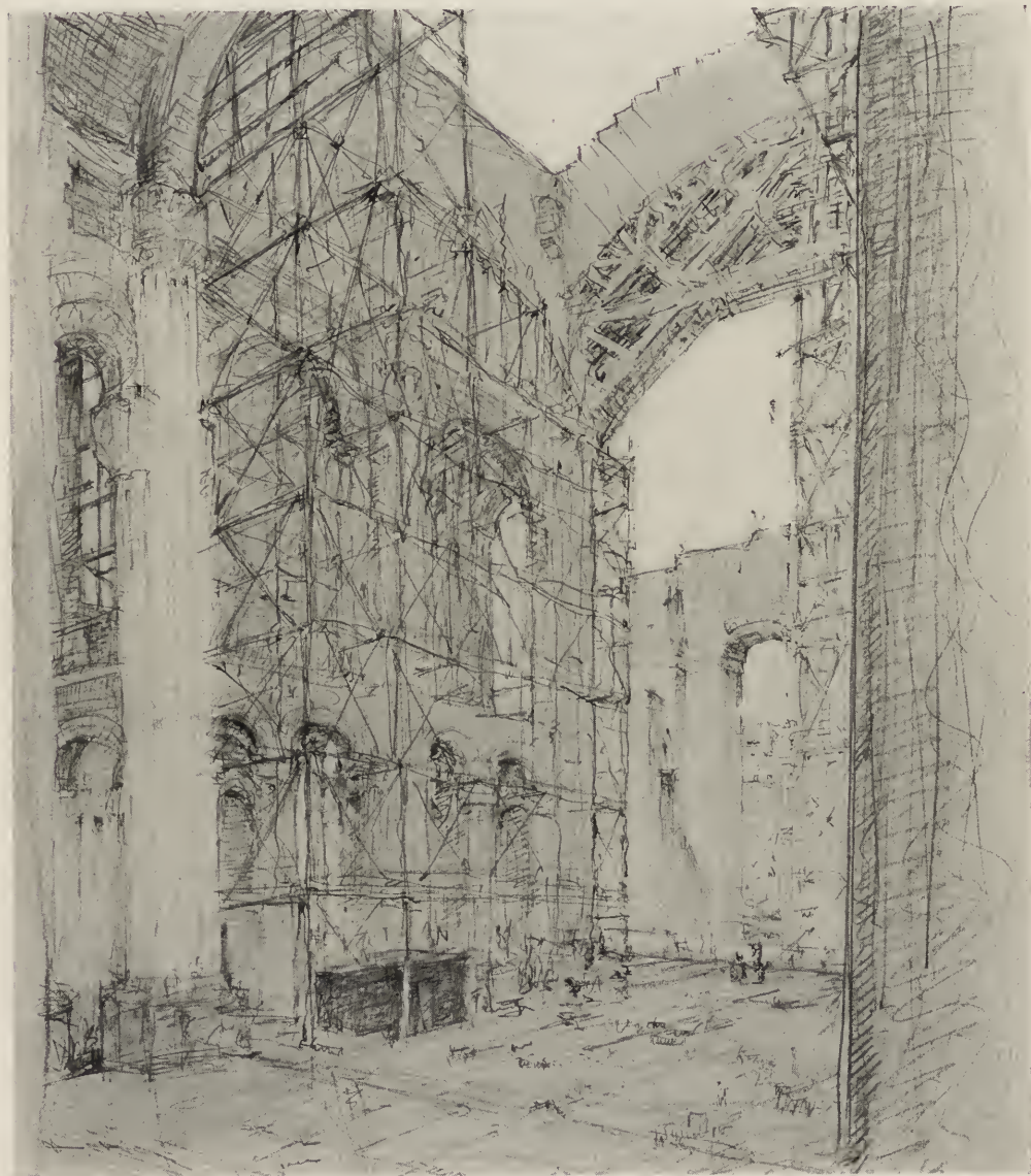
View westward from inside the Cathedral apse, in the opposite direction from that of opposite page. Here the completed arch is shown against the sky, and the southwest pier (one of the four on each corner of the square crossing) appears in the distance beneath the arch. Through the scaffolding may be seen the inside stone facing of the chancel. The crypt, in which service is now held, is directly beneath this chancel floor.
