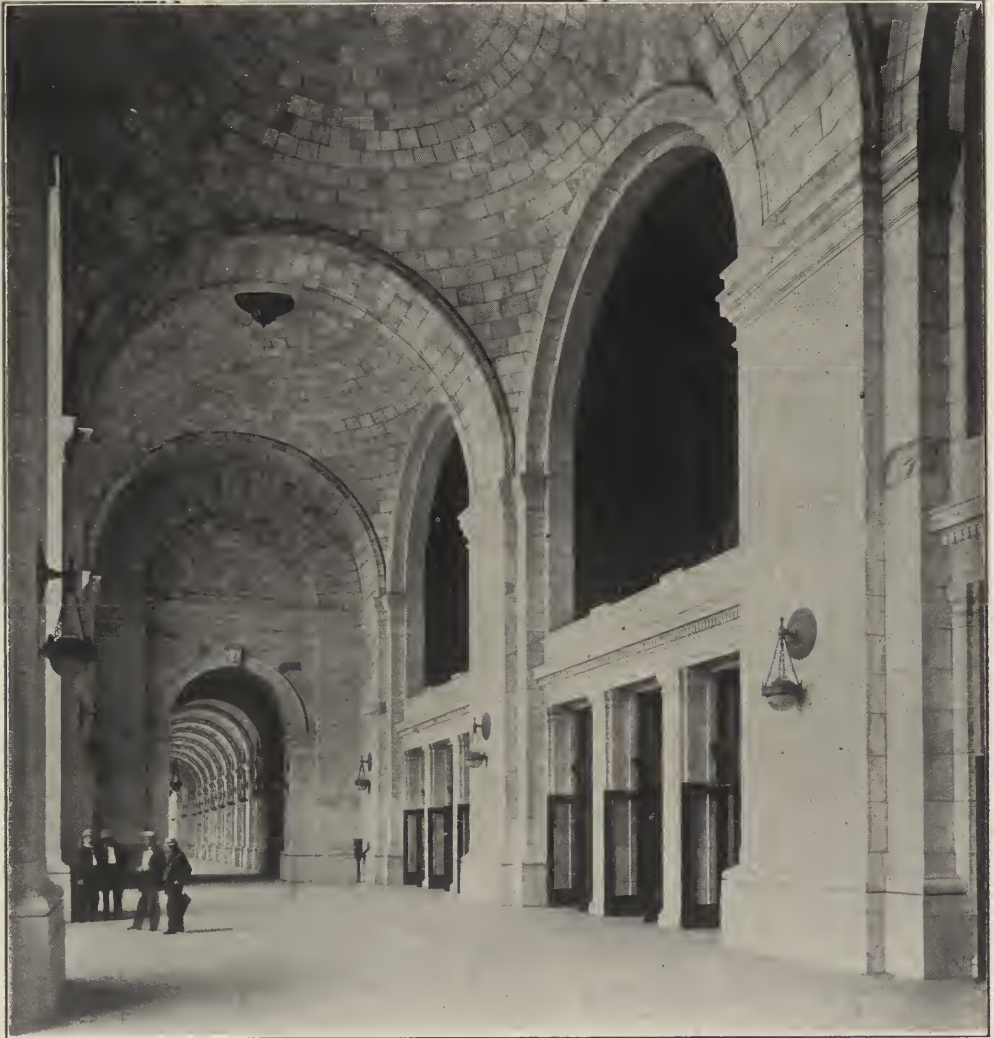
THE UNION STATION—PORTICO AND MAIN ENTRANCES.
