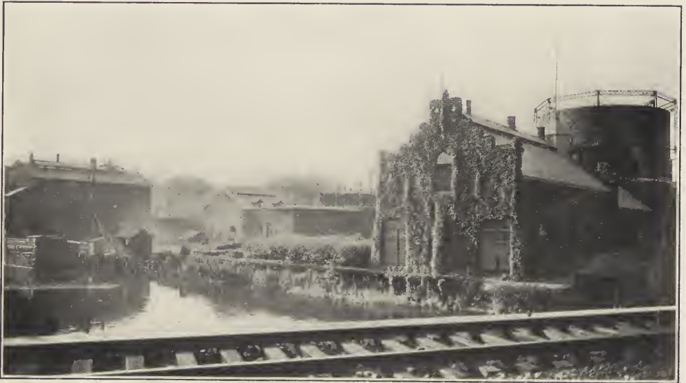
FIG. 17. GAS WORKS AT WEST FARMS.
