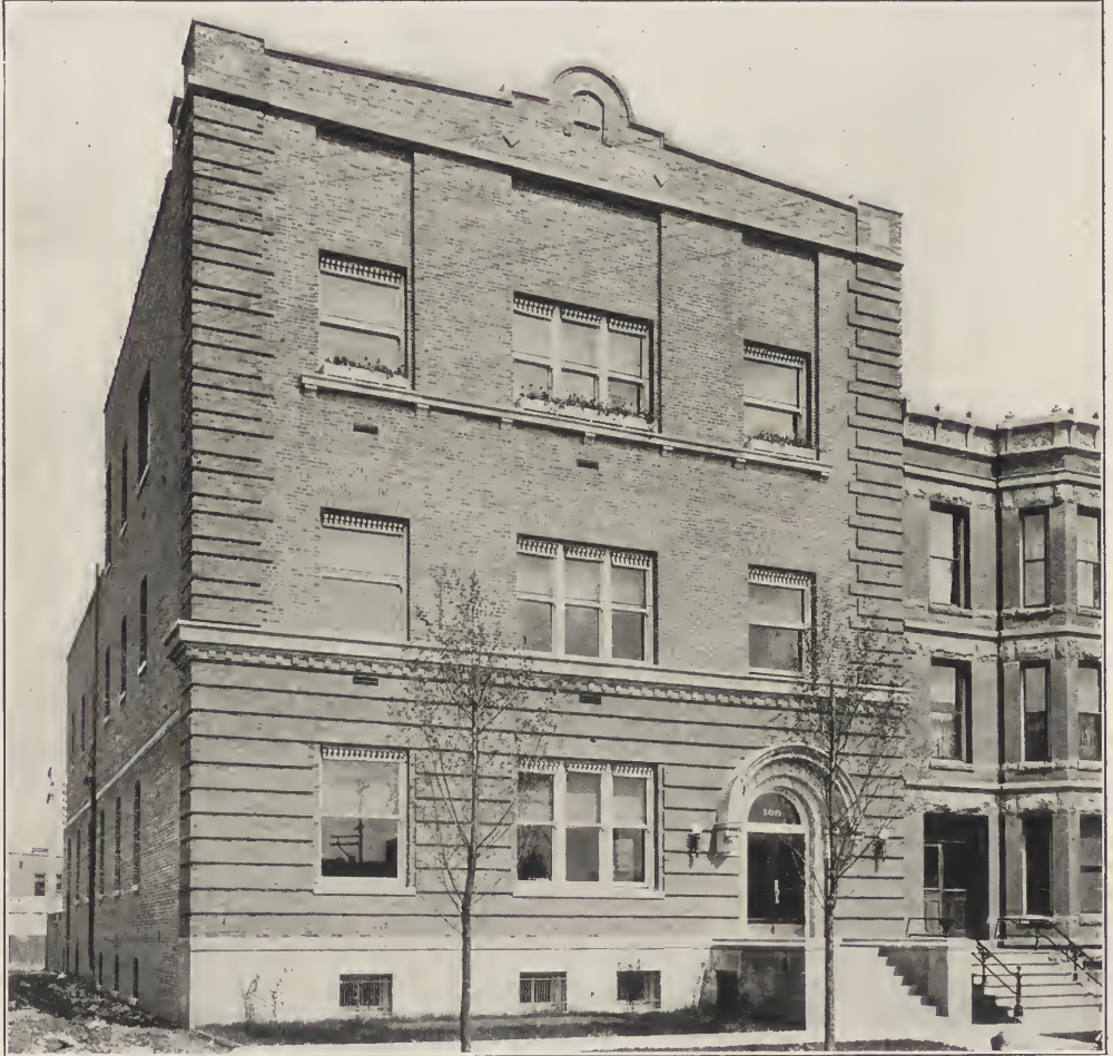
"KEDZIE" EXCHANGE, CHICAGO TELEPHONE COMPANY.
