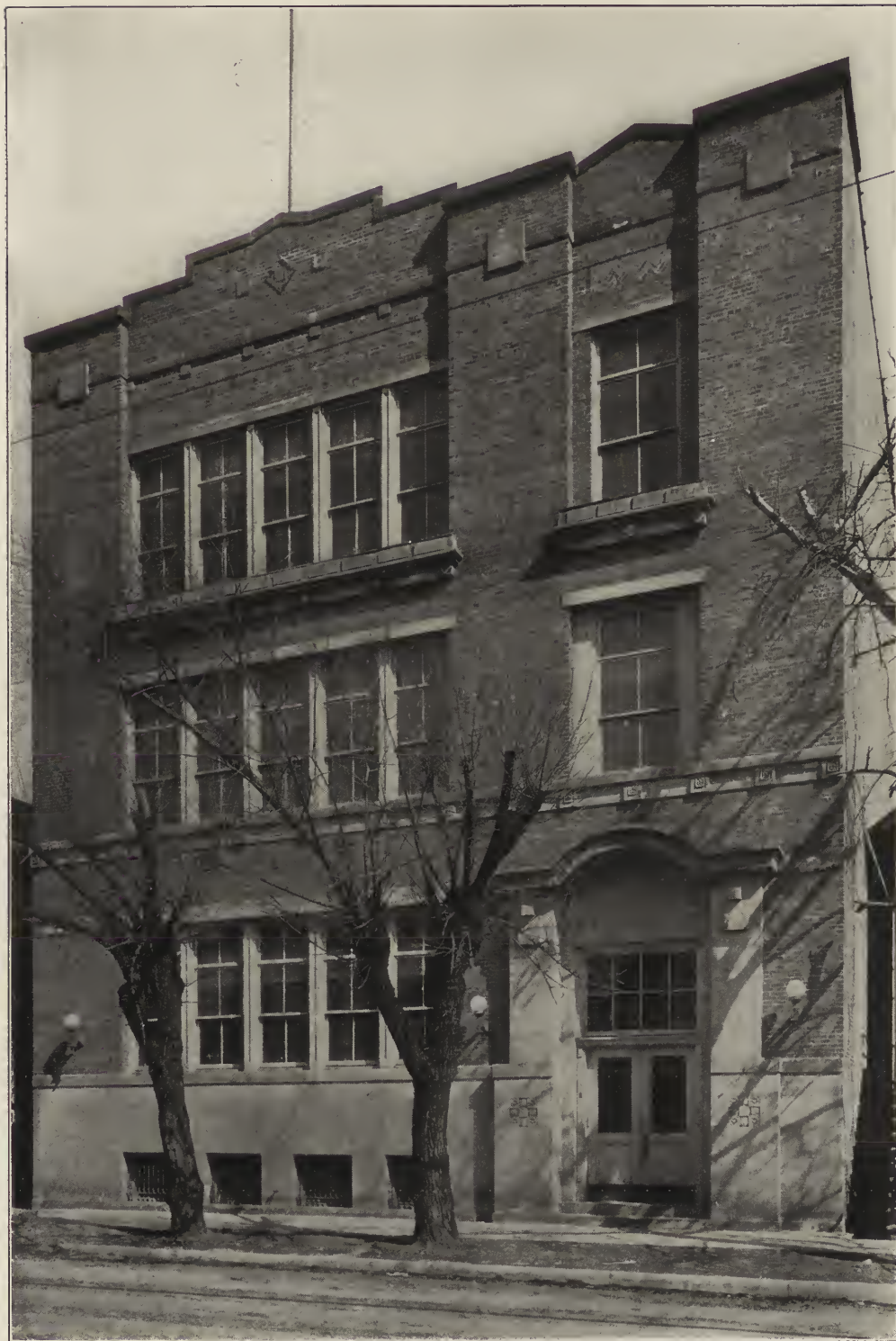
"LINCOLN" EXCHANGE, CHICAGO TELEPHONE COMPANY.
