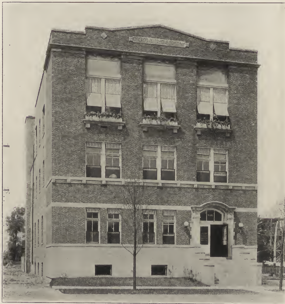
"EDGEWATER" EXCHANGE, CHICAGO TELEPHONE COMPANY.
