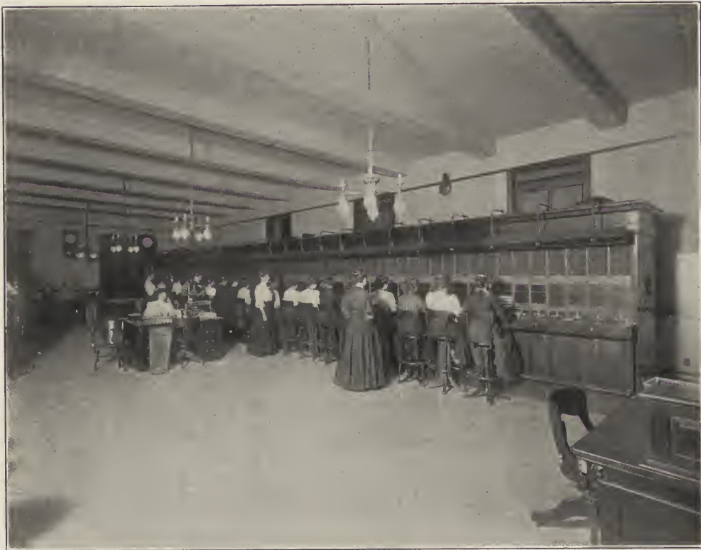
OPERATING ROOM AT "KEDZIE" EXCHANGE, CHICAGO TELEPHONE COMPANY.
