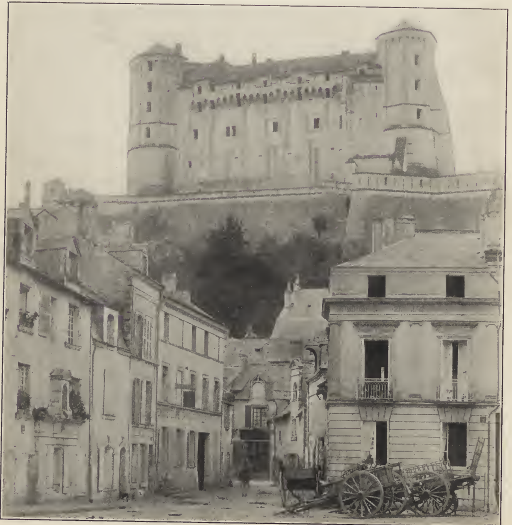
SAUMUR—THE CASTLE AS SEEN FROM THE STREET SKIRTING THE LOIRE.
