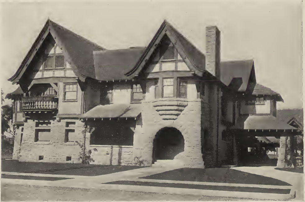
FIG. 11. DWELLING IN LOS ANGELES, CAL.
