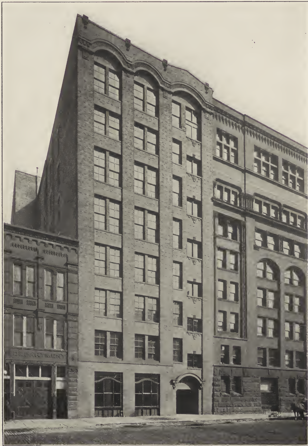
"TOLL AND LONG DISTANCE" EXCHANGE FOR THE CHICAGO TELEPHONE COMPANY. Pond & Pond, Architects.
