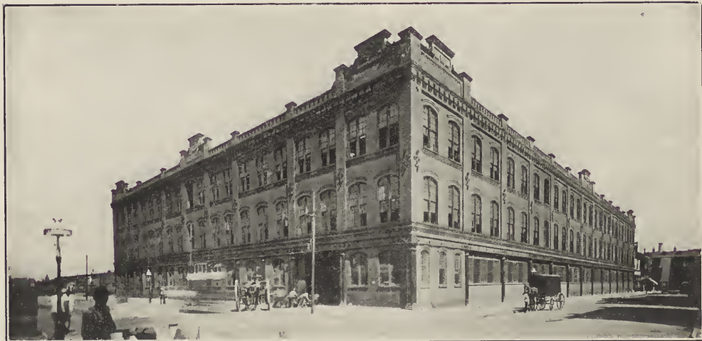
FIG. 12. CAR BARN OF THE NEW YORK CITY RAILWAY CO. Madison Avenue and 129th Street, New York.
