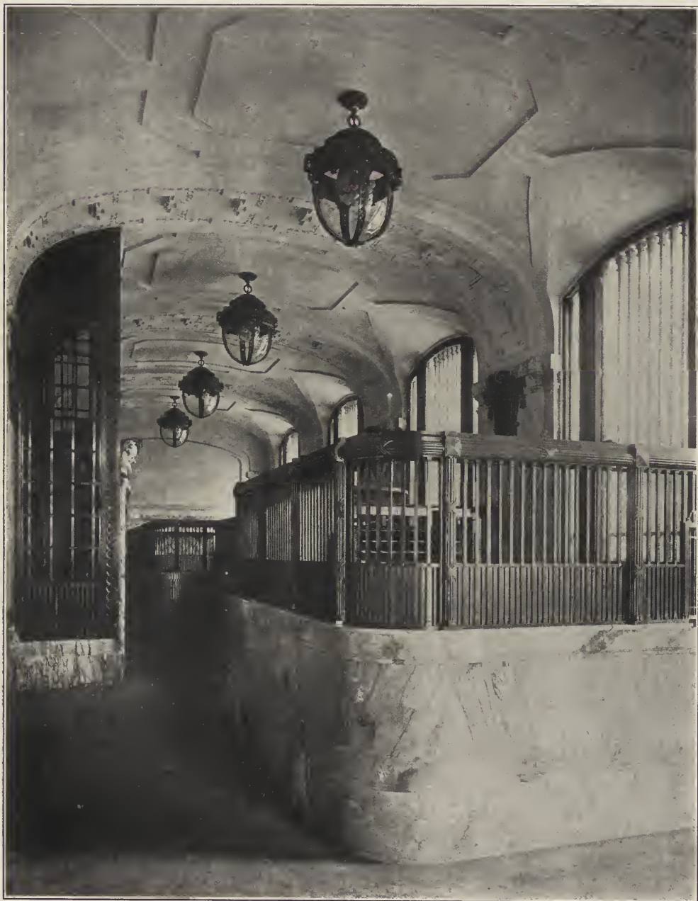
IMPORTERS' AND TRADERS' NATIONAL BANK—VIEW IN FIRST FLOOR BANKING ROOM. Murray Street and Broadway, New York. J. H. Freedlander, Architect. (Photo by A. Patzig.)
