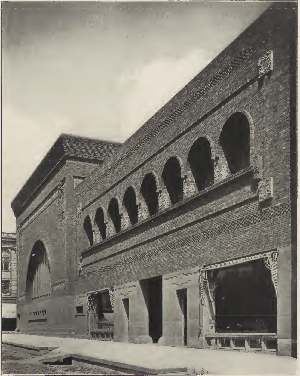
NATIONAL FARMERS' BANK OF OWATONNA, MINN.—VIEW OF SIDE.
