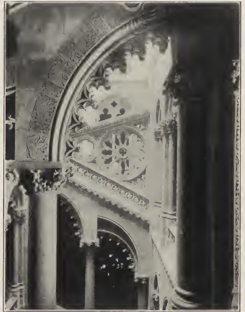
AT THE TOP OF THE SENATE STAIRCASE.
