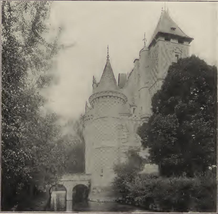
THE CHATEAU OF REAUX—VIEW OF HOUSE AND MOAT.
