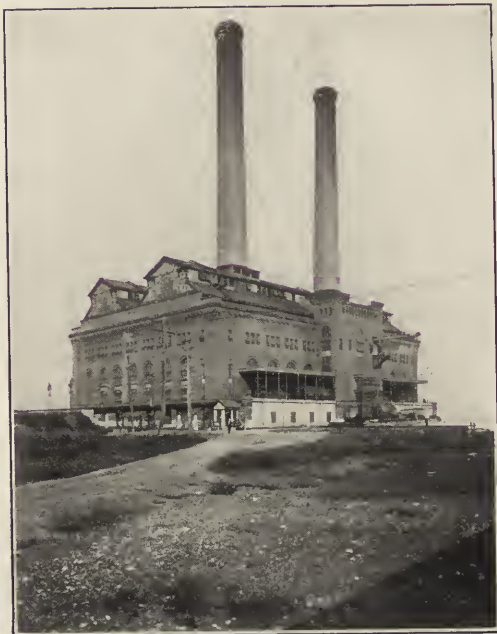
Fig. 15. Power House of the New York Central. Morris Dock, New York City. Reed & Stem, Architects.
