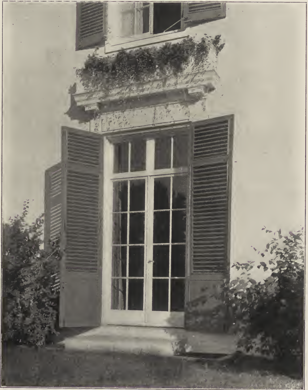
HOUSE OF MR. JOHN J. CHAPMAN—DETAIL OF A WINDOW. Barrytown, N. Y.
