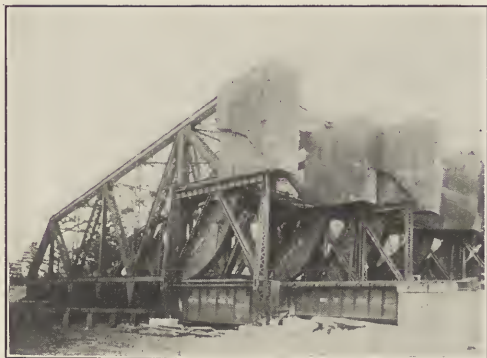
FIG. 2. THE "ROLLER LIFT" BRIDGE. Bronx River, New York City. Bridge Dept., N. Y., N. H. & H. R. R. Engrs.
