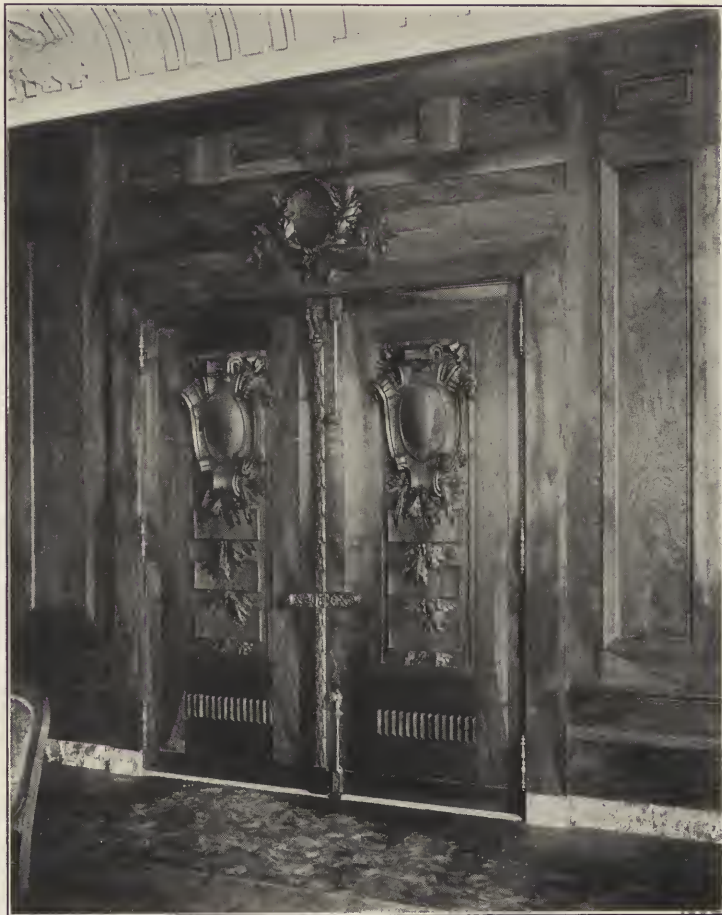
IMPORTERS' AND TRADERS' NATIONAL BANK—ENTRANCE DOORS IN DIRECTORS' ROOM.
