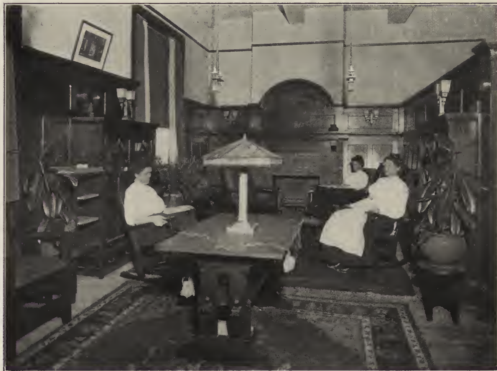
REST ROOM, "KEDZIE" EXCHANGE, CHICAGO TELEPHONE COMPANY.
