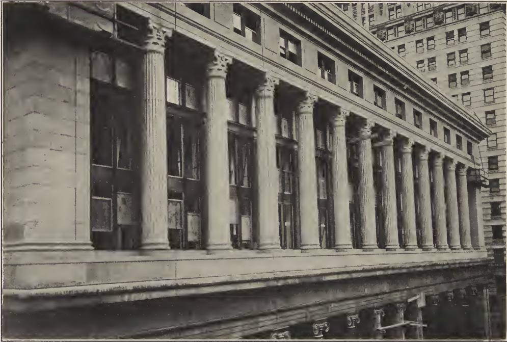
NATIONAL CITY BANK—DETAIL OF NEW UPPER STORIES.
