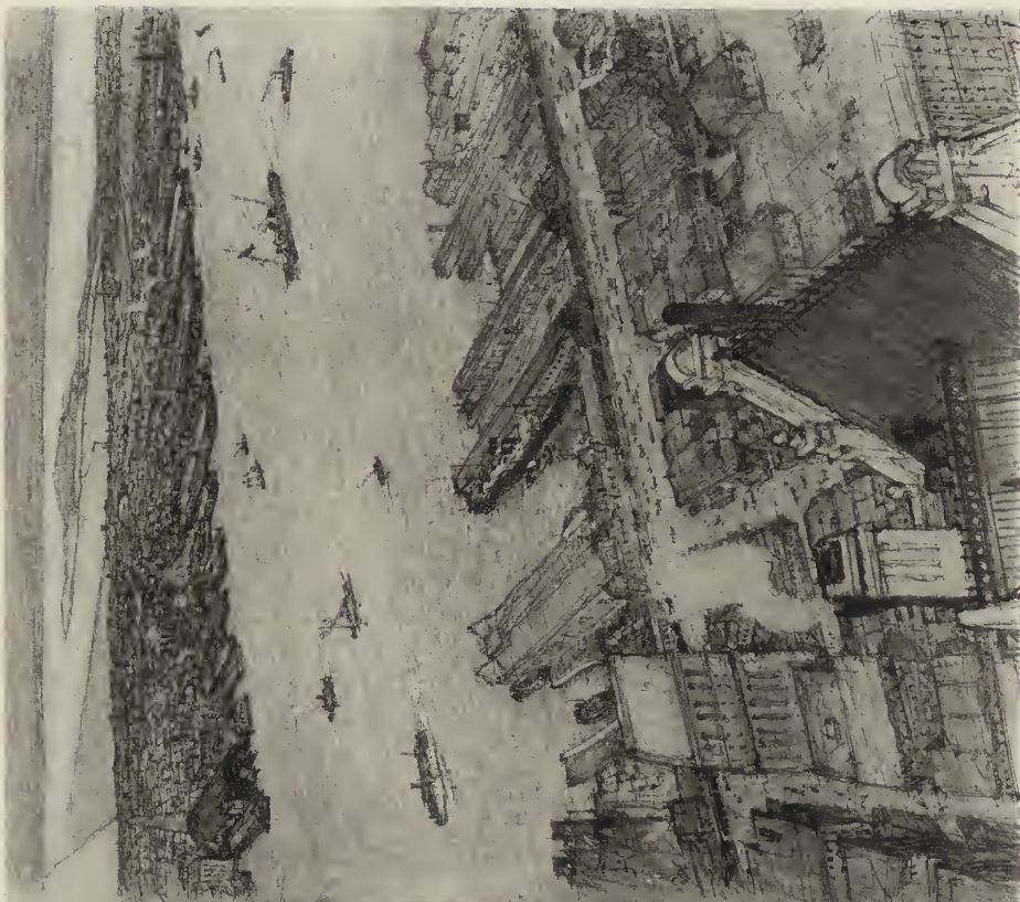
View from the Singer Building, looking west over the North River and Jersey City, with the City Investing Building in the immediate foreground. The Jersey river front is shown from the long, dark Pennsylvania train shed on the left to the station tower of the D., L. & W. Railroad on the right.
