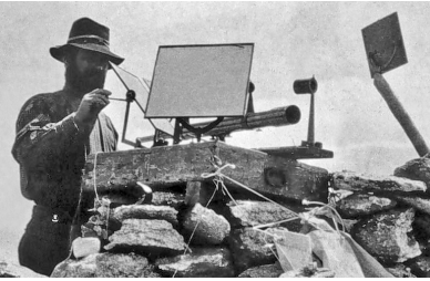
b / A surveyor on a mountaintop uses a heliotrope.
