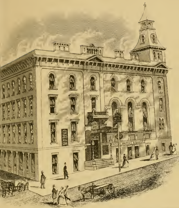
W. H. Wood BOARD OF TRADE BUILDING COR. MADISON & WATER STS.
