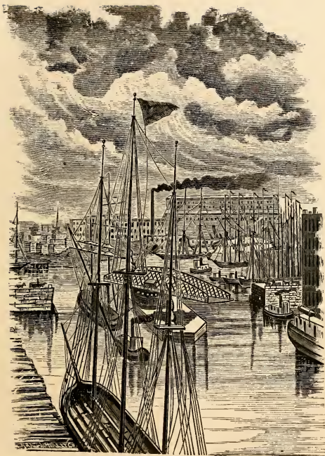
CHICAGO RIVER, LAKE STREET BRIDGE.
