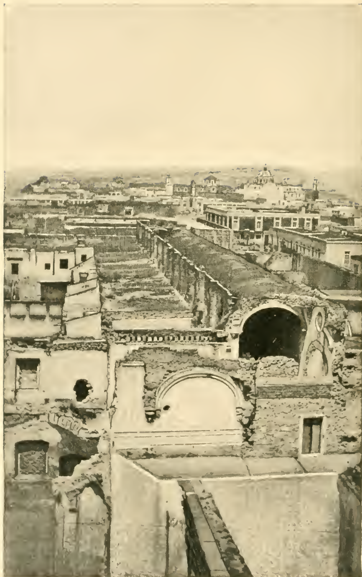
COVERED WAY OF THE INQUISITION, Connecting with the Examining Chapel.
