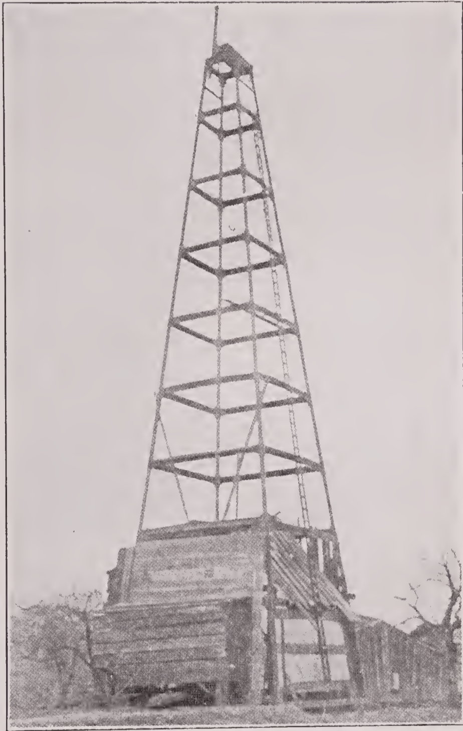
Fig. 15. A steel framed derrick. (Photo by Ill. Survey).
