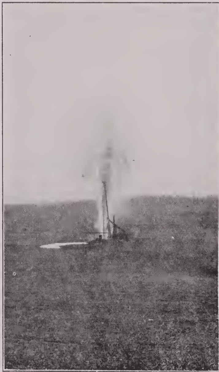
Fig. 22. Broad Ripple oil well after shooting.
