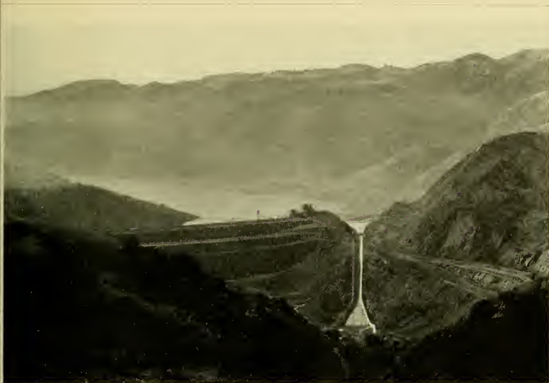
Calaveras Reservoir dominates the trans-Bay (or Alameda) Division of Spring Valley's catchment system. It is replenished by the streams of a very productive watershed in the Mt. Hamilton spur of the Coast Range. Water is released into Alameda Creek, percolates through the Sunol gravels, and enters the Sunol Aqueduct.
