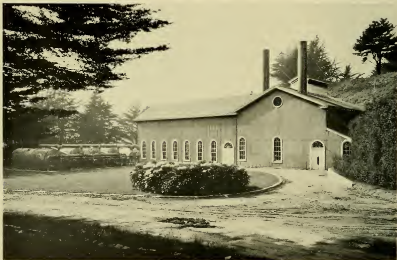
The Lake Merced (or "City") pumping station, situated on the east shore of the lake, takes water from Lake Merced and also "boosts" water flowing to the city from San Andres Reservoir. The Lake Merced sand-screens adjoin the pumping station. These pumps were installed in 1891.
