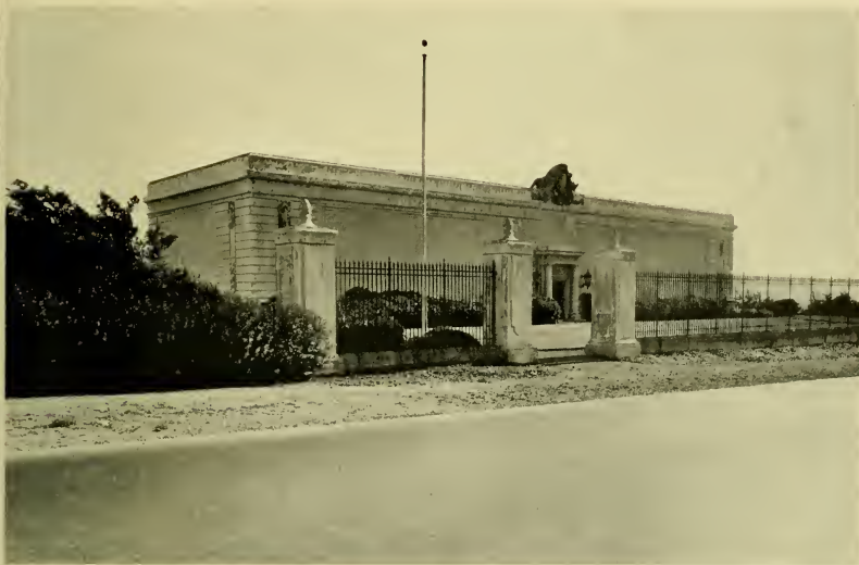
On Sloat Boulevard at Twenty-second Avenue, against the background of Lake Merced, stands Central Pumps, the largest pumping station in Spring Valley's distributing system. The water coming into the city reaches these pumps through a concrete reservoir near by, and is pumped to Laguna Honda at the rate of eight million gallons per day.
