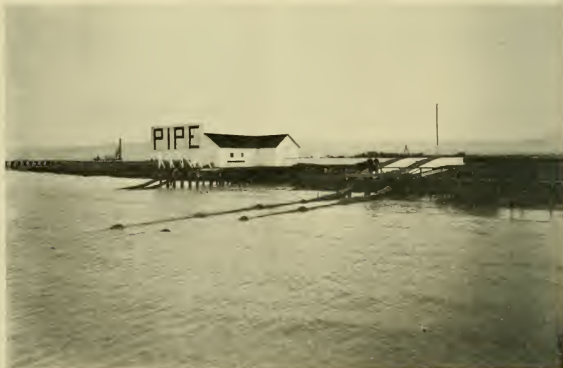
At Ravenswood, on the Bay shore of San Mateo County, the submarine pipes emerge, carrying water from the Alameda Division of Spring Valley. There are four of these submarine pipes; they were constructed with flexible joints to rest on the bottom of the Bay. Their construction in 1888 by Hermann Schussler, set an engineering precedent.
