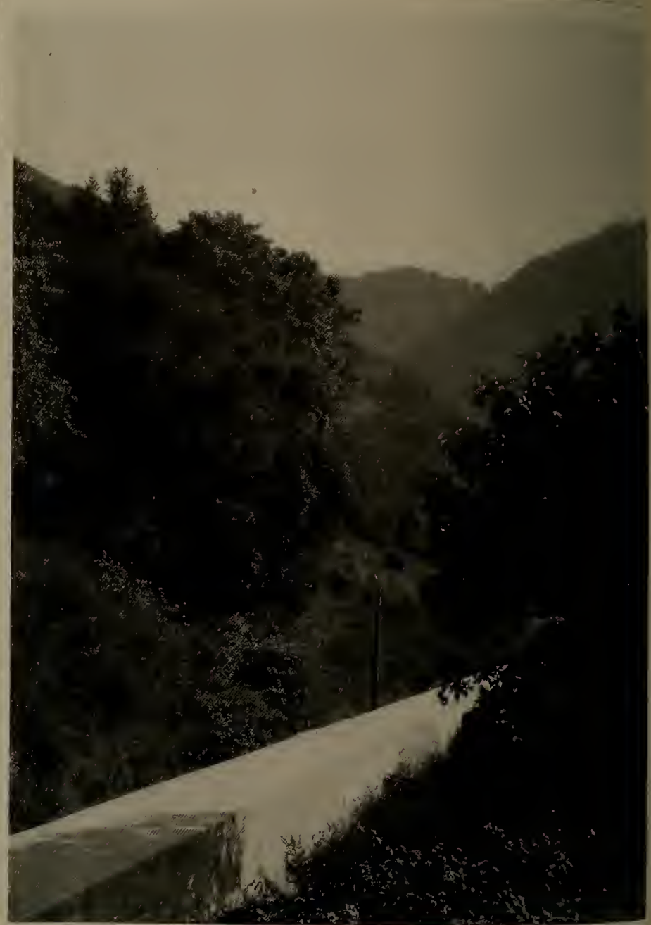
Emerging and disappearing as it threads the winding gorge of Niles Canyon, a great white aqueduct that can carry seventy million gallons of water a day reminds us that, while utility is paramount, structural beauty is not necessarily ignored by those who build for the public weal
