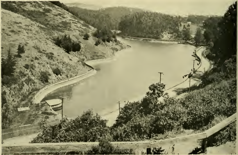
The first built of Spring Valley's three major distributing reservoirs in San Francisco is Laguna Honda, at Seventh Avenue opposite Ortega Street. When Pilarcitos water was first brought to the city in 1862, it was delivered here, and this "deep lake" has been part of the city system ever since. At elevation 370 feet, it supplies high city areas.
