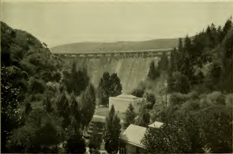
A down-stream view of Crystal Springs, the huge concrete dam that dominates the Peninsula Division of Spring Valley. In the foreground, the Crystal Springs auxiliary pumping station. Along the curving crest of this dam runs the Skyline Boulevard, immediately above the waters of Crystal Springs, largest of the peninsular reservoirs.
