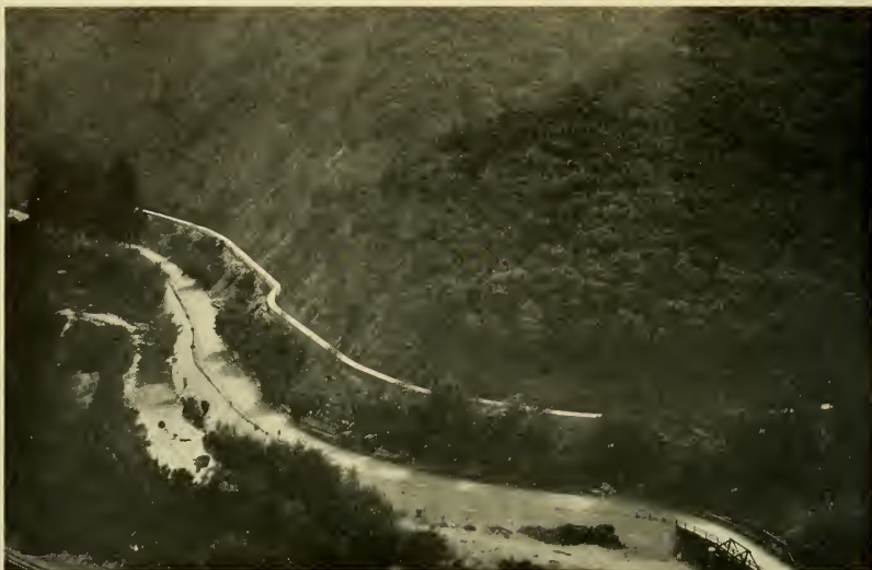
This picture, with that adjoining on page eleven, presents a panoramic view of Niles Canyon. Above the railroad, on a bench of the steep hillside, is the great concrete Sunol Aqueduct which carries Calaveras, Sunol, and Pleasanton water as far as Niles. There the water passes through Niles Reservoir to pipe-lines that convey it across the Bay.
