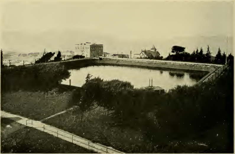
When Spring Valley absorbed the old San Francisco City Water Works, it took over two distributing reservoirs on Russian Hill, Lombard-street reservoir (pictured here), and that at Francisco and Hyde. These historic reservoirs, which originally stored water from Lobos Creek in the Presidio, have been continuously in use for sixty-five years.
