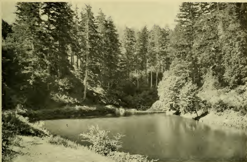
Two miles below Pilarcitos, near the dividing-line between the oceanside and the interior watershed of the San Mateo hills, the Stone Dam was built to intercept the productive flow of streams that would otherwise waste to the Pacific. This is perhaps the most charming spot to be found on all the Spring Valley properties.
