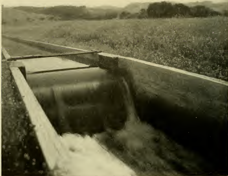
The Hetch Hetchy line to Crystal Springs Reservoir tunnels the hills west of Redwood City, and the water, hidden from the light of day during all its long journey from Sunol, finally comes out of the Pulgas Tunnel to flow thus for a brief space before plunging into Crystal Springs Lake
