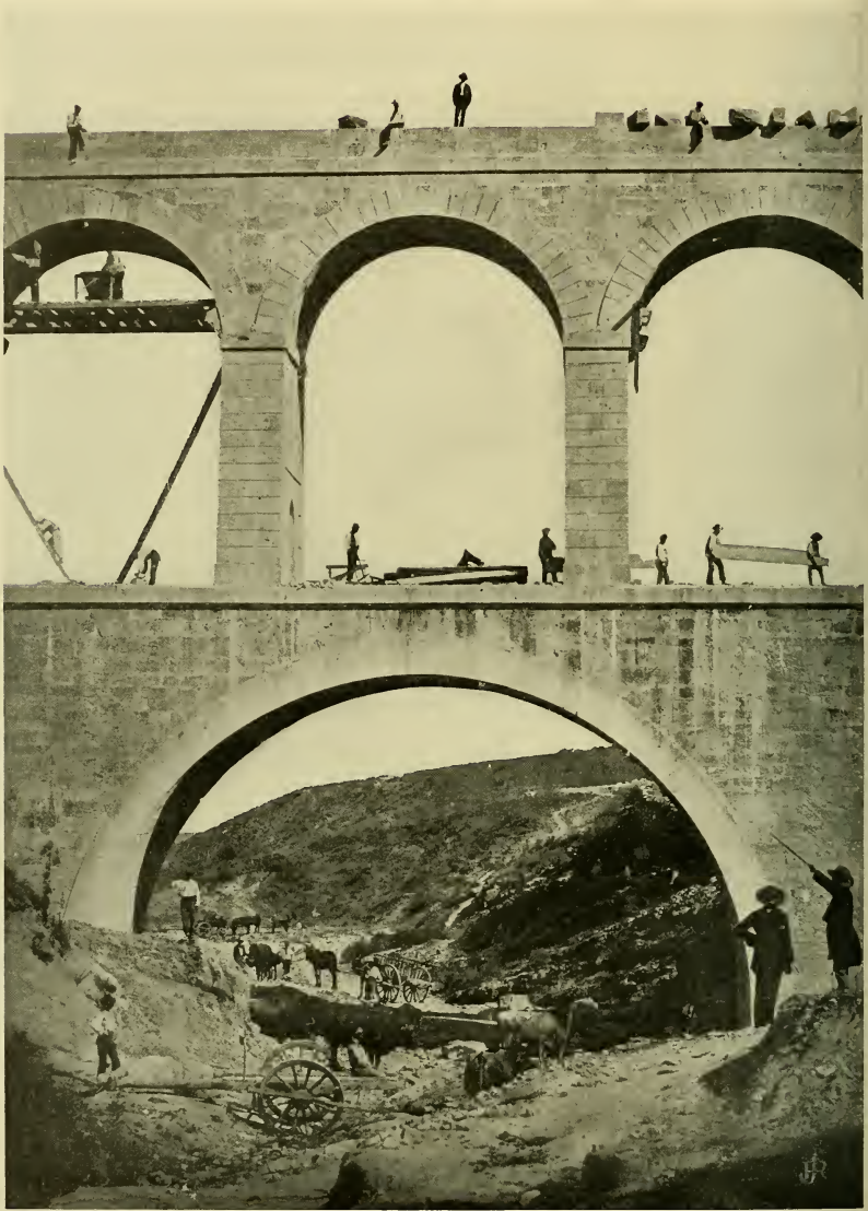
Lozoya water on its way to Madrid, a city about the same size as San Francisco. The Madrid Water Conduit—so the works are called—dates from the late fifties of the last century, like our water supply. This photograph was taken during construction, and records a time when hydraulic engineers wore frock coats and canes.
