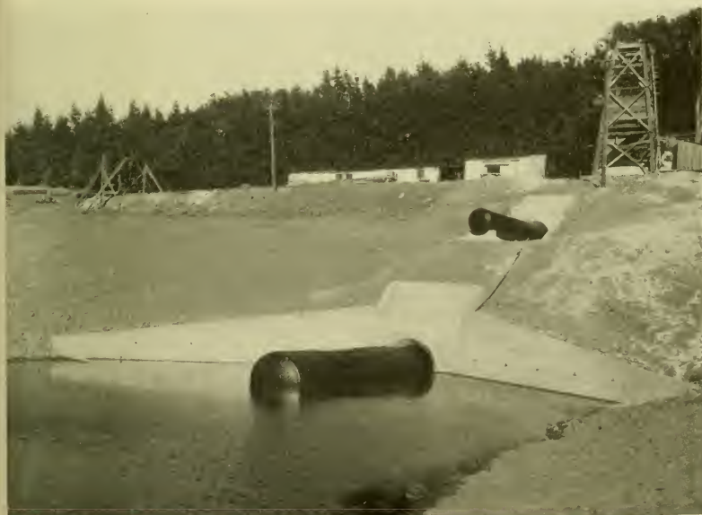
Large screens protect the lakeside tunnels against intrusion of foreign substances
