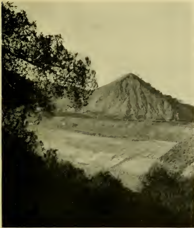
Up-stream slope of Calaveras Dam, with Observation Hill beyond. Out of the borrow pit on this hill over two million yards of material have been taken
