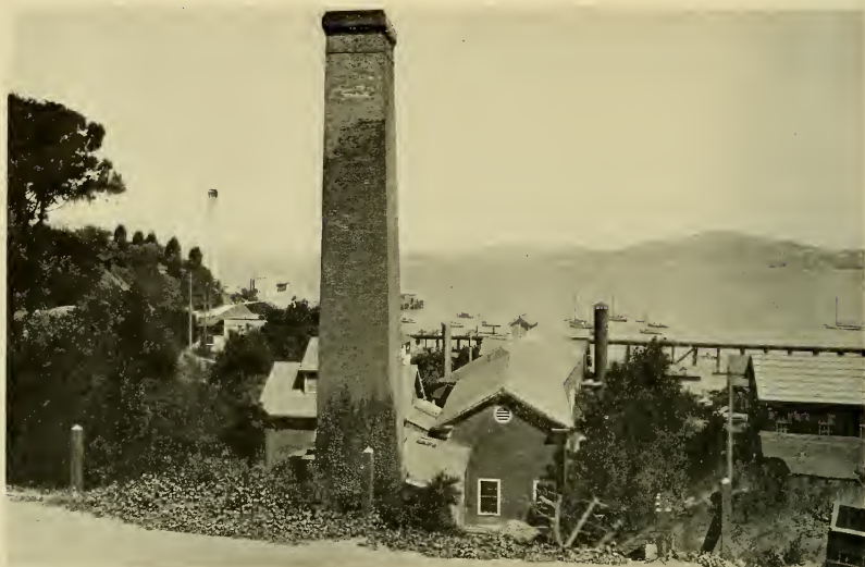
The brick stack of Black Point Pumps is a landmark of San Francisco; it has towered above the inner reaches of the Golden Gate, at Van Ness Avenue and Beach Street, ever since 1858. This pumping station used to serve the pioneer Russian Hill reservoirs. It now receives water from University Mount and lifts it to Presidio Heights.
