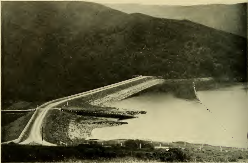
Second in size of the three San Mateo County storage reservoirs is San Andres, which takes its name from a valley famous in the annals of the Spanish explorers. In 1868 an earthen dam was thrown across San Andres Creek, forming this artificial lake. Though San Andres earthquake fault runs through the dam, it suffered no damage in 1906.
