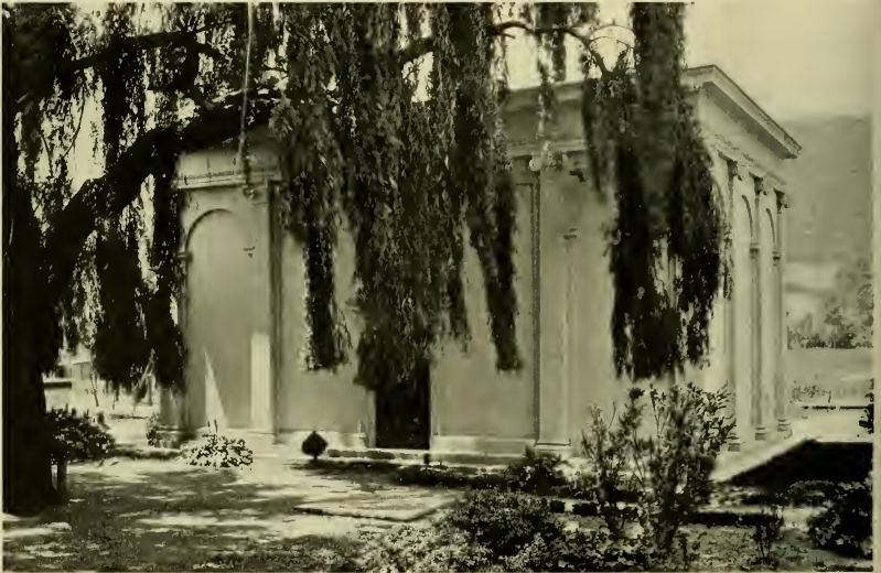
The Pleasanton pumping station is situated at the outlet of Livermore Valley. Hereabouts Spring Valley has in operation some seventy-five wells to draw water from the underground gravels which are fed from a drainage area of 400 square miles. The pipe-line to the Water Temple at Sunol has a capacity of twenty million gallons per day.
