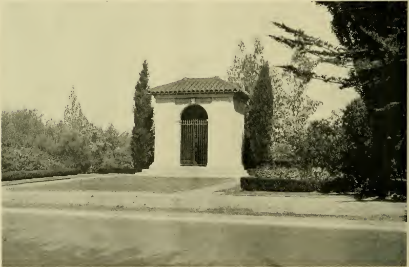
The Venturi meters at this station on the Highway twelve miles south of San Francisco are master-meters, measuring all the water that enters the City from Spring Valley sources. This station stands at the entrance to the Millbrae pumping station, the headquarters for the Peninsula Division, as Sunol is for the Alameda Division, of the Company.
