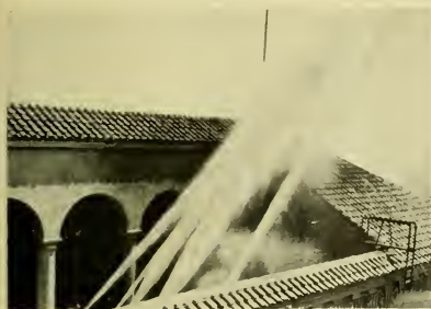
Testing the "throw" from the stand-pipes of the Standard Oil Building. The streams are topping the roof of the al-fresco garden, which is twenty-two stories—more than three hundred feet—above the sidewalk
