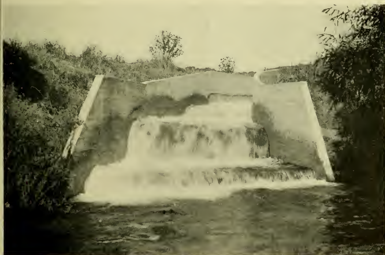
Spring Valley water from Calaveras Reservoir pouring through the City's Pulgas Tunnel into Crystal Springs Reservoir. Pulgas Tunnel is the western terminus of the Hetch Hetchy Conduit, and is used to deliver Calaveras water into the largest of Spring Valley's peninsular reservoirs. Eventually it will also deliver Hetch Hetchy water.
