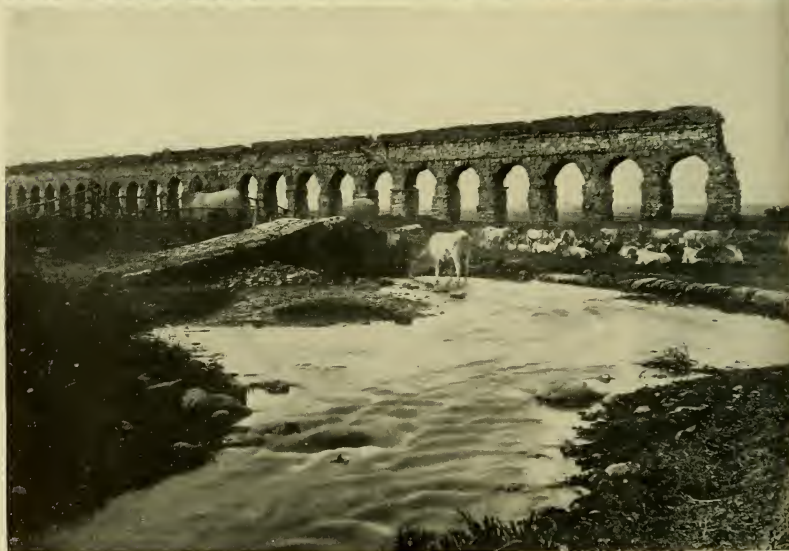
Aqua Claudia, one of the most famous of ancient Rome's eleven aqueducts, was begun by the Emperor Caligula in A. D. 38, and completed by the Emperor Claudius in A. D. 52. Its farthest spring, the Fons Albulinus, was about forty-five miles from Rome. It crossed ravines and tunneled hills until within seven miles of the city, entering upon a magnificent line of arches.
