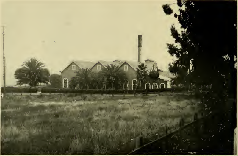
Twenty-one million gallons of water flowing daily to San Francisco from the Alameda Division of Spring Valley passes through Belmont Pumps, twenty miles south of San Francisco. This is a strategic point on the line, for by the time water from across the Bay reaches Belmont it has exhausted its gravity momentum and needs "boosting."
