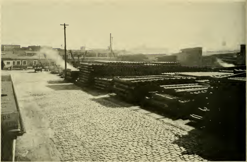
On Bryant Street, between Fourth and Fifth, is the Spring Valley Yard, where all water-meters are tested before installation. The Yard is headquarters for 120 pipe men, service and meter men, and machinists. Here are kept in stock the thousand and one items that must be instantly available in the water service of a large city.
