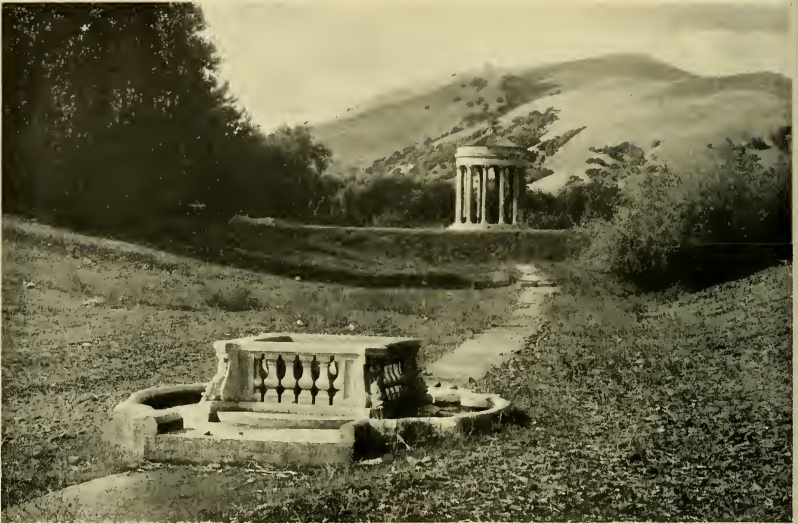
The famous Water Temple at Sunol draws innumerable sightseers. Here may be seen "the meeting of the waters"—from Calaveras Reservoir, the Sunol infiltration galleries, and the Livermore Valley wells. Here these waters mingle and start on the long flow down Niles Canyon, across the Bay, and up the San Mateo peninsula to San Francisco.
