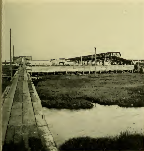
The Bay Division of Hetch Hetchy Conduit begins at Irvington, crosses the Bay near Spring Valley's pipe-line, from Dumbarton to Ravenswood, and terminates in Crystal Springs. Left: Spring Valley line enclosed in flume, with connection to City line where this leaves Ravenswood bridge. Right: The Nilcs-Irvington line.
