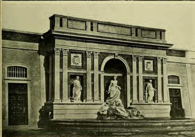
Madrid derives its water supply from the Valley of the Lozoya. There, at an elevation of 8,040 feet above the sea, a granite-walled stream is diverted and carried forty-three miles to the capital. Above, a reservoir on this great system. It is shown incomplete; after roofing, it was covered with earth. Below, the Old Reservoir in Madrid, where art does honor to water.
