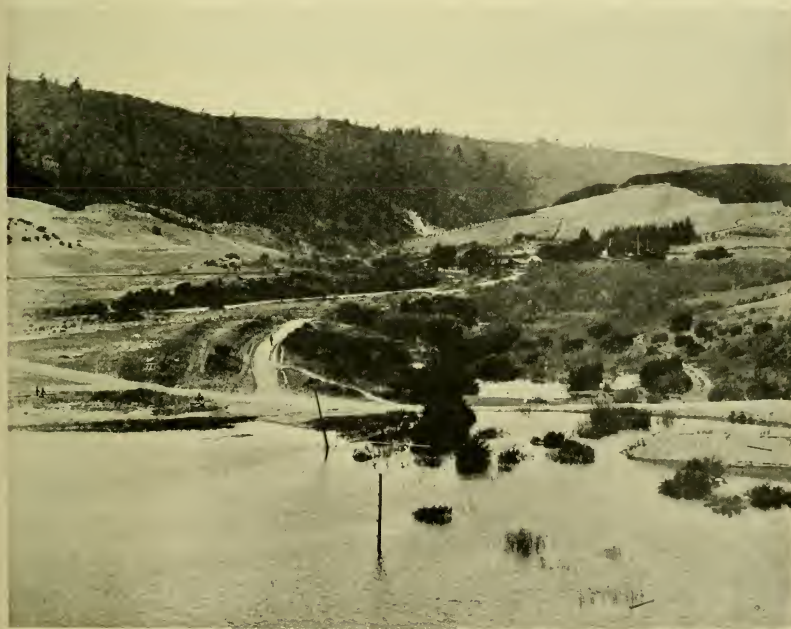
Site of Crystal Springs Reservoir as it appeared in 1887, when work started on the huge concrete dam
