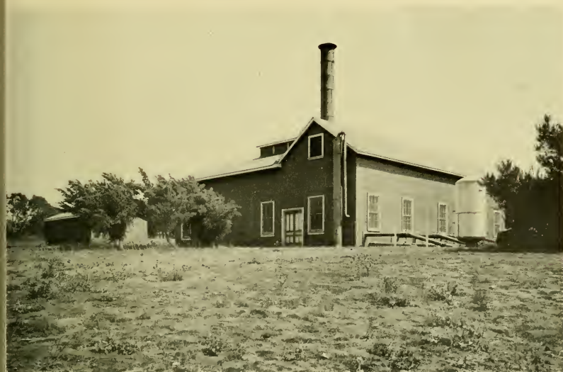
Less than a mile southeast of Lake Merced Pumps is the Ocean View pumping station, which pumps San Andres and Pilarcitos water to Laguna Honda. It was built in 1907 at the time that Pilarcitos Reservoir became a feeder to San Andres, to lift the increased supply coming into the city through the new Merced branch of the San Andres line.
