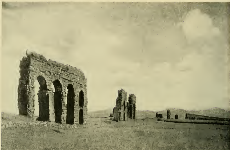
Claudia and Anio Novus of the great Roman water system, with the Alban Hills in the background. Claudia was built of dimension stone; Anio Novus, on top of it, of small stone and concrete
