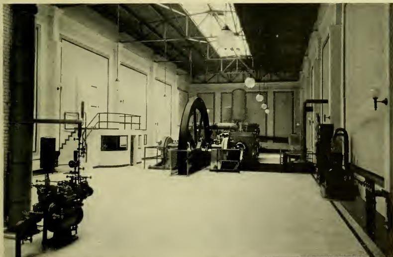
Interior view of Central Pumps. Simplicity of architectural design gives this utilitarian structure unusual beauty. A gallery has been provided for the convenience of visitors. The station was constructed in 1911 on a plan which will permit its extension when additional units are necessary.
