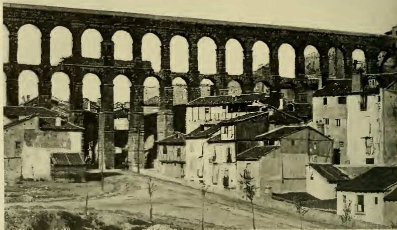
This section of the Roman aqueduct of Segovia, called El Puente, traverses a deep valley, the suburbs, and part of the city. For part of the distance it has two stages. It is built entirely of blocks of granite, without either mortar or clamps. The main storage reservoir for Segovia's supply of mountain water is outside the city, beyond El Puente.
