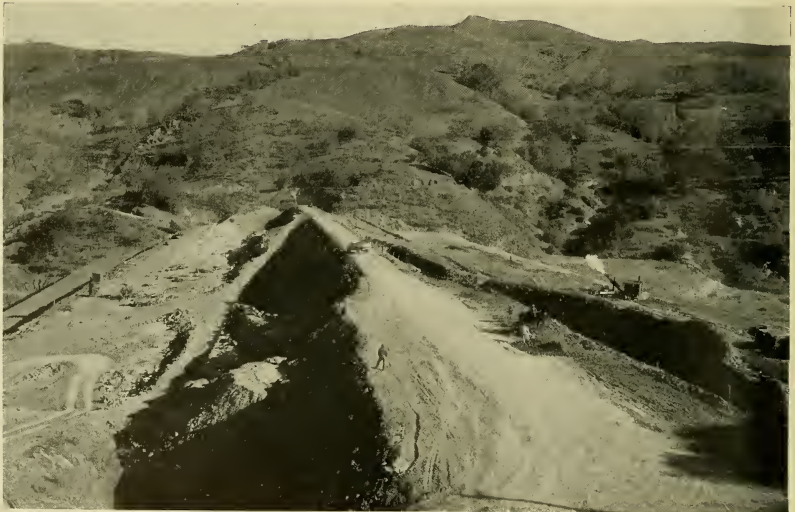
Present work at Spring Valley's Calaveras Dam approaches completion. When this picture was taken, at the beginning of December, 1924, there were 2,677,000 cubic yards of material in place
