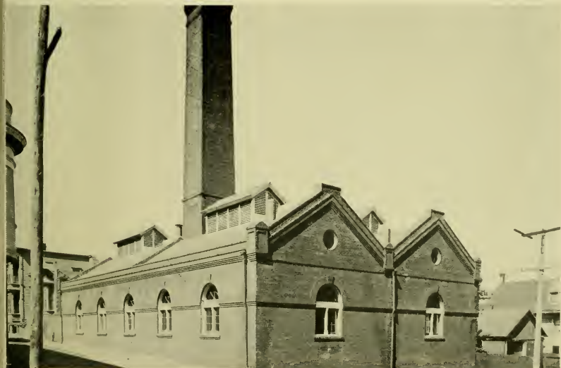
On Seventeenth Street, between Sanchez and Noe, is the Clarendon Heights pumping station. It is typical of the smaller pumps serving numerous regions into which the city has been districted for supply and fire-protection purposes. It lifts water to Stanford Heights, filling a five-million-gallon reservoir at an elevation of 620 feet.
