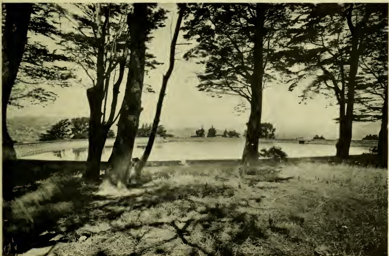
On a spur of Bernal Heights, at Appleton Avenue and Elsie Street, College Hill distributing reservoir was constructed in 1870 at an elevation of 255 feet to meet the growth of San Francisco and to supply sections of our hilly city on levels lower than those necessarily served by Laguna Honda Reservoir.
