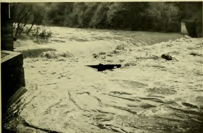
Alameda Creek is a "flashy" stream that has torrential flows in the height of the winter rainy season. The water here seen wasting over Sunol Dam is now conserved, and its release controlled, by Calaveras Reservoir. The conduit from the Water Temple to the Sunol Aqueduct pierces the dam transversely.
