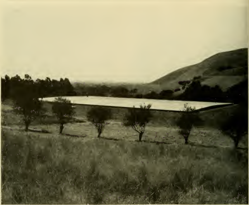
Cuddled in a fold of the hills near the town of Niles, this reservoir, dug deep in the cool clay, receives water from the Sunol-Niles Aqueduct and releases it for the journey to Irvington, where it enters the Bay Division of the Hetch Hetchy Conduit and crosses the Bay to Crystal Springs
