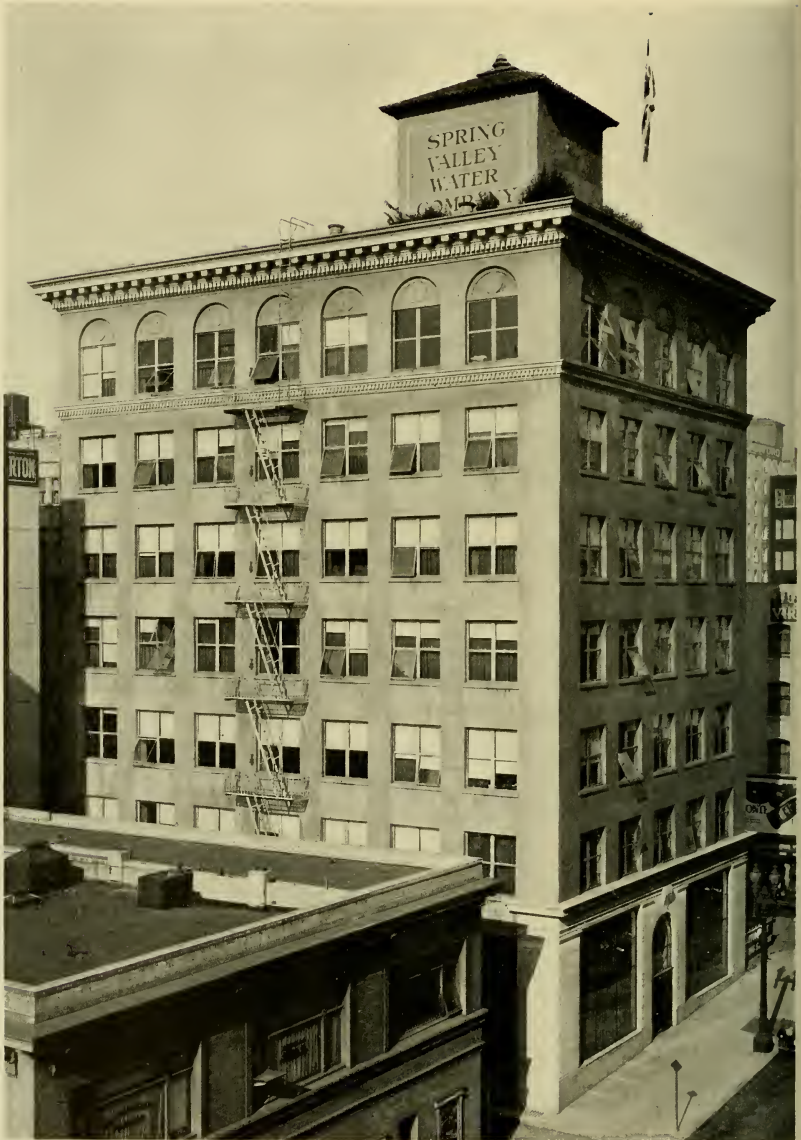
The Directors' rooms, the executive offices, the engineering, water sales, agricultural, real estate, and other departments of Spring Valley are housed in this reinforced concrete structure designed for the Company by the late Willis Polk. It stands on the west side of Mason Street between Geary and Post. Occupancy dates from October of 1923.
