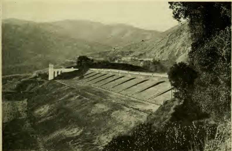
Calaveras Dam is one of the big earth-fill dams of the world. It closes the outlet of the long narrow valley that has been converted into Calaveras Reservoir. The white tower houses the gate-valves that control the release of water through a tunnel to the creek channel below the dam.
