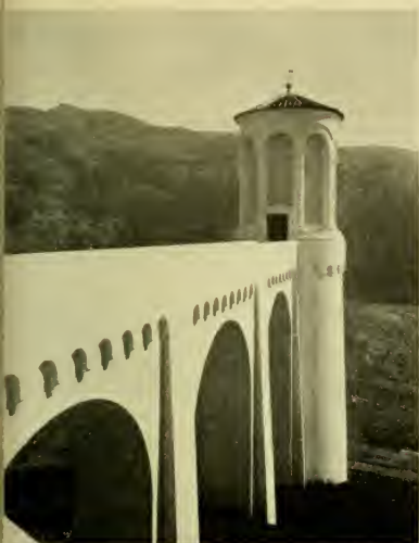
From this gate-house the release of Calaveras water is controlled. The entrance is pictured on the cover of this issue. The Latin inscription "Lympha Optima" proclaims that "Water Is Best"
