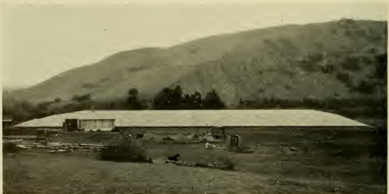
Spring Valley's Niles Reservoir, completed and roofed over, will receive Calaveras water at the outlet of the Sunol Aqueduct
