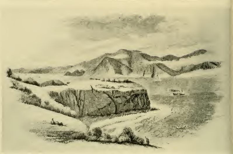
Fort Point used to be Punta del Cantil Blanco, and the old Spanish fort was called Castillo de San Joaquin. This was built of adobe, with embrasures lined with brick. The parapet was ten feet thick. It mounted eight nine-pounders. Finished in 1794, it cost about sixty-four hundred dollars
