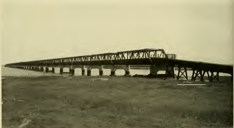
On this steel bridge constructed by the City of San Francisco the Bay Division of the Hetch Hetchy Conduit emerges from the Bay at Ravenswood in San Mateo County, paralleling the emergence of Spring Valley's own conduit. Through this Hetch Hetchy line Spring Valley water flows to Crystal Springs
