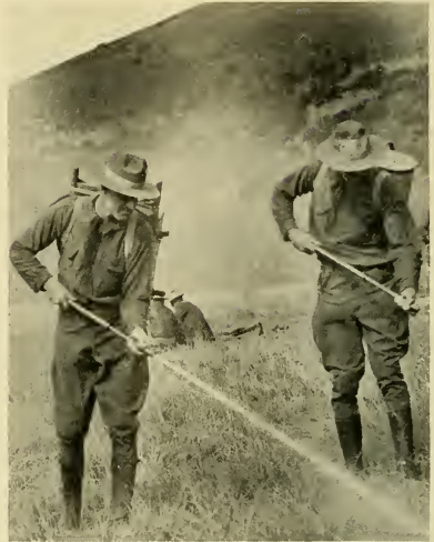
To put out flames in burning logs and dead trees, the forest rangers use a hand force-pump attached to a metal water-container strapped on the back "Alaska pack" fashion
