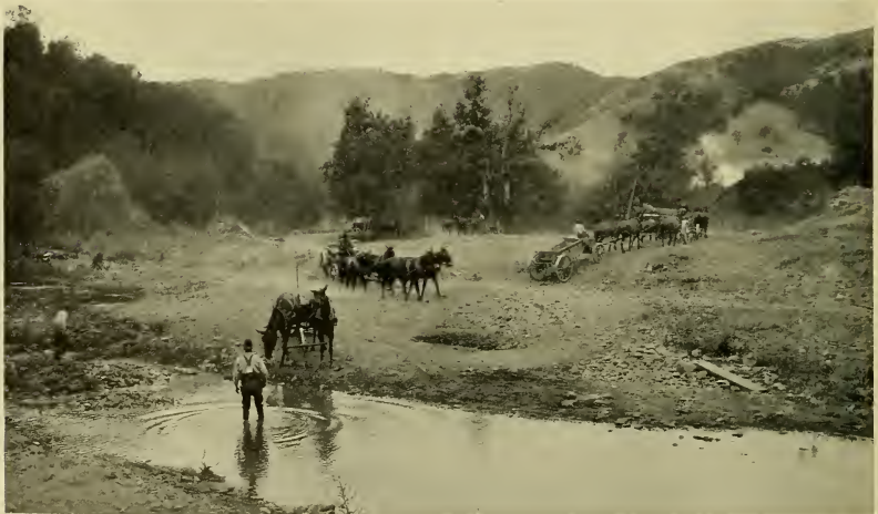
Before Calaveras Reservoir existed. The huge Spring Valley dam now spans this outlet of beautiful Calaveras Valley. This picture was taken as workmen began clearing the valley floor
