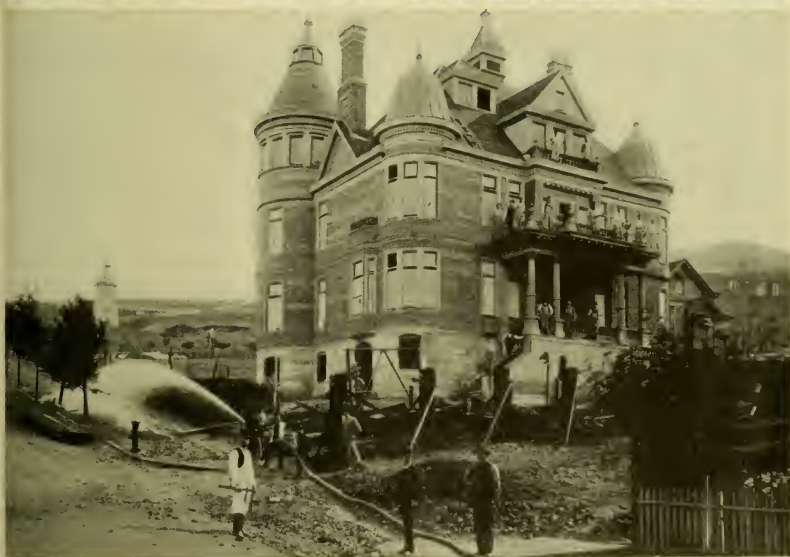
The circular structure in the upper picture Mr. Clarke described as "the large brick reservoir." Below is the Clarke home, at Douglass Street and Caselli Avenue. The hose is being played to demonstrate water pressure
