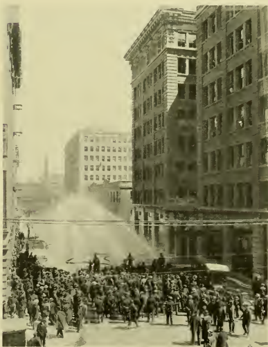
A concentration of high-pressure lines demonstrated on New Montgomery Street
