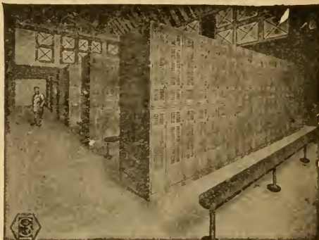
Some of the 6,000 Durand-Steel Lockers installed in the Public Gymnasium of Chicago. 12'x 15'x 42", Double Tier.
