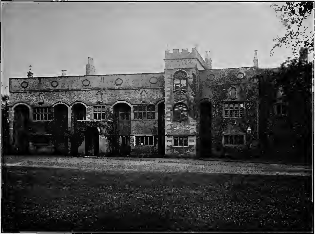
HALE HALL : THE NORTH FRONT
