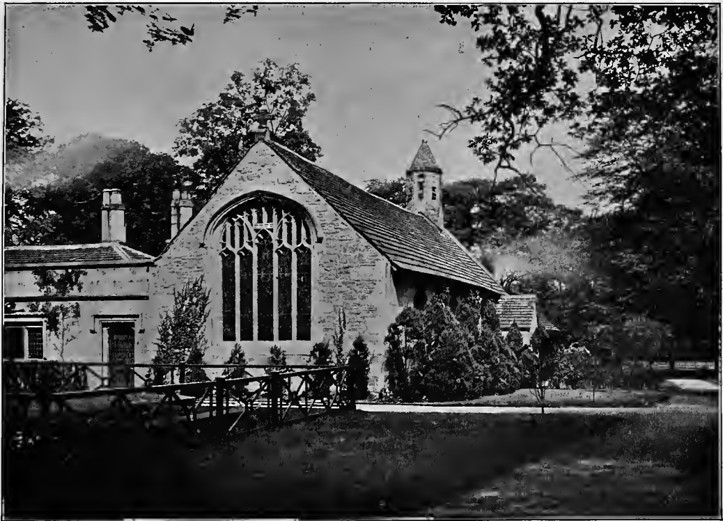
LATHOM CHAPEL : THE EAST END
