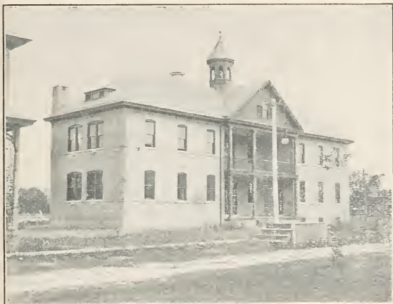
THE ASSEMBLY HALL
