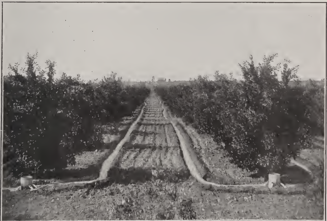
FIG. 2.—ORCHARD IRRIGATION WITH CONCRETE STANDS.
