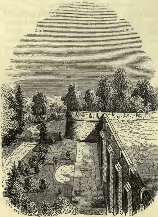
SLOPES, FROM THE NORTH-EAST ANGLE OF THE TERRACE.
