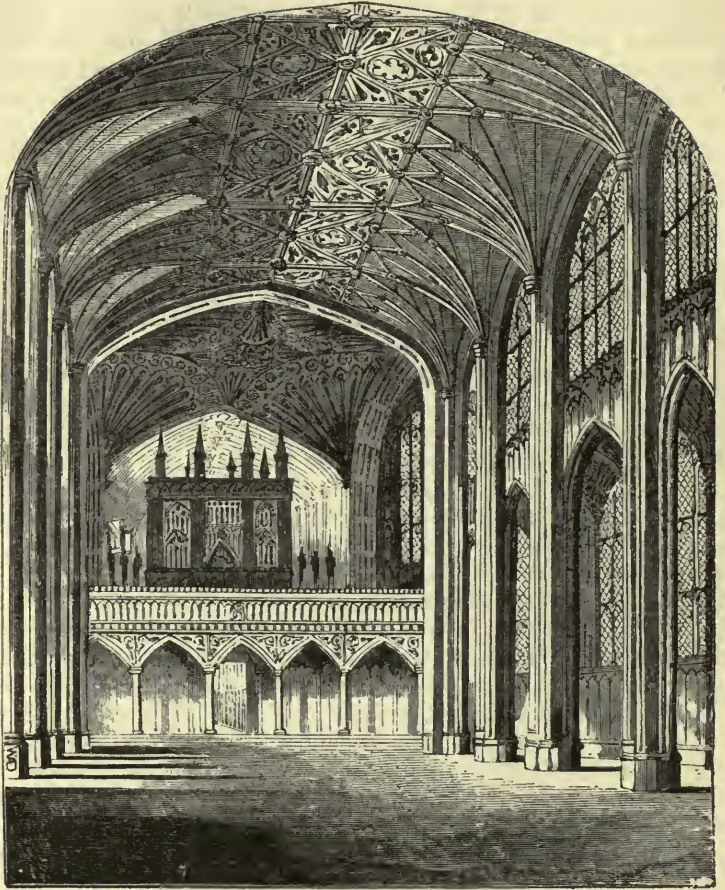
INTERIOR OF SAINT GEORGE'S CHAPEL, LOOKING TOWARDS THE CHOIR
