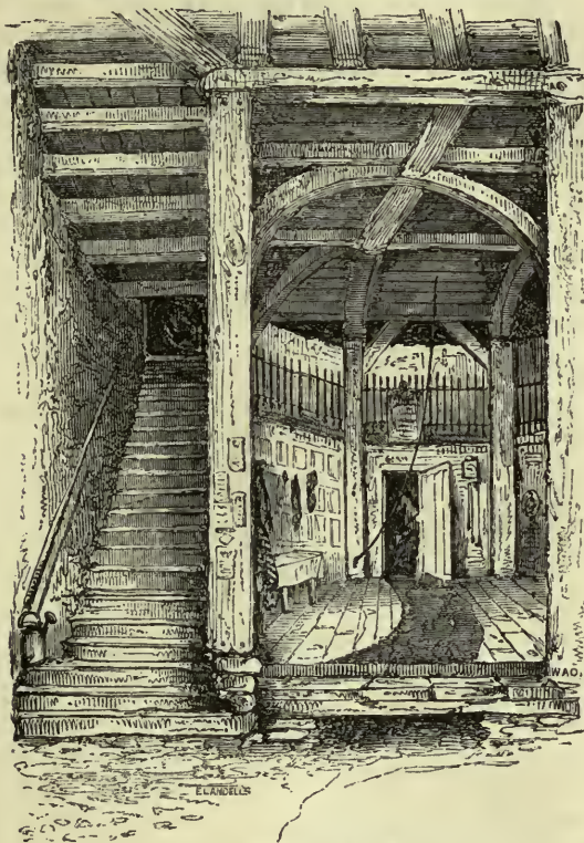
INTERIOR OF THE CURFEW TOWER.
