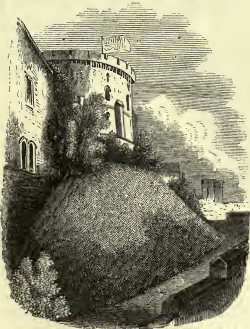
ROUND TOWER FROM THE SOUTH-EAST, WITH COVERED WAY FROM SAINT GEORGE'S GATE
