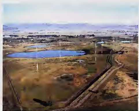
Figure 5. An aerial view of the WWVB antenna systems.
