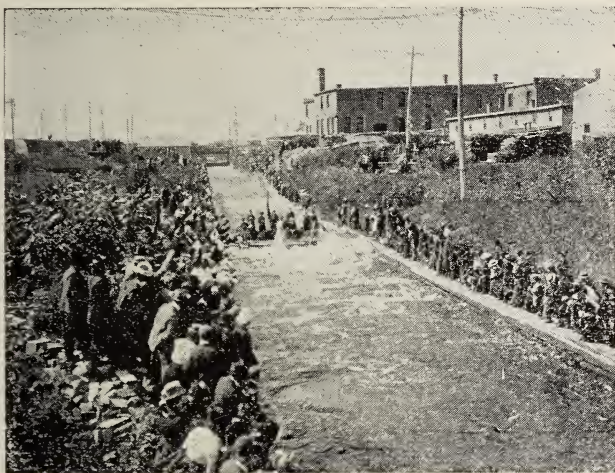
KING GEORGE (Duke of York) Running Timber Slides.
