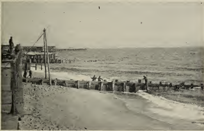
Building a Jetty
