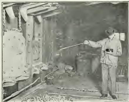
Method of Using Thwing Radiation Pyrometer
