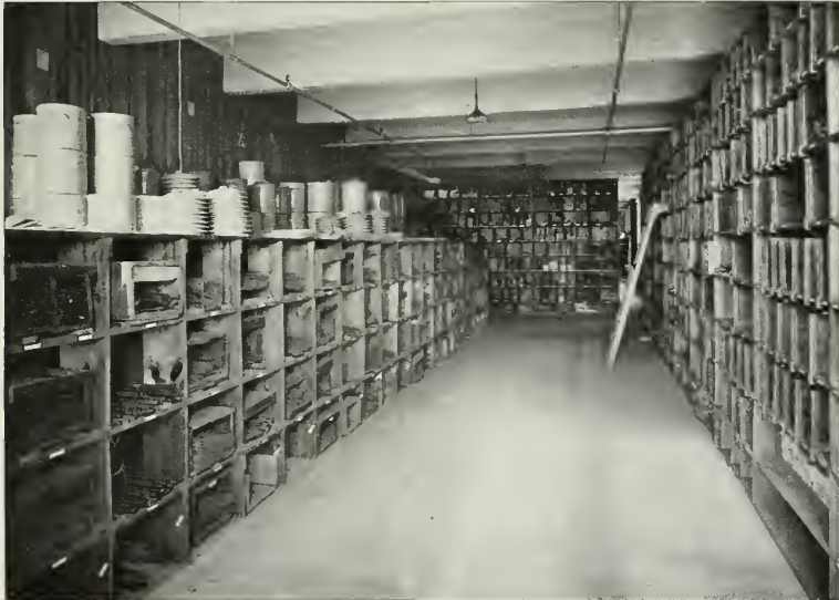
View in Stock Room Showing Adjustable Partitions on Right and Glass Tubing on Left
