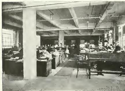
View in Office
