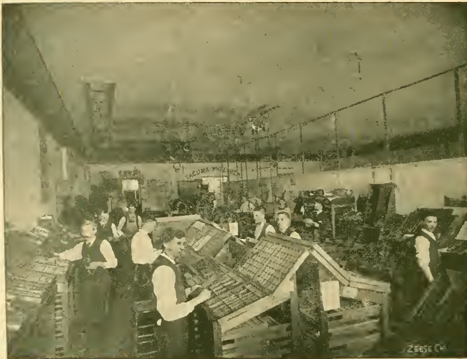
PUGET SOUND PRINTING COMPANY'S OFFICE.
