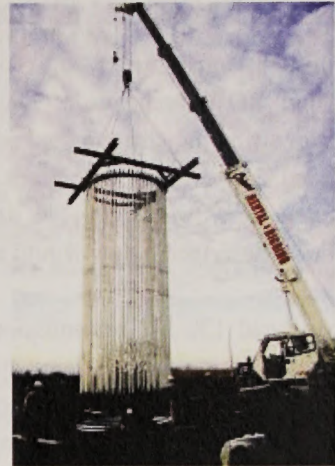
Figure 2.3-10. Bolt Structure for Tower Foundation.
