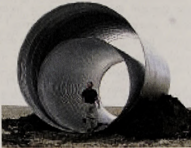
Figure 2.3-9. Two Steel Conduit Foundation Forms.
