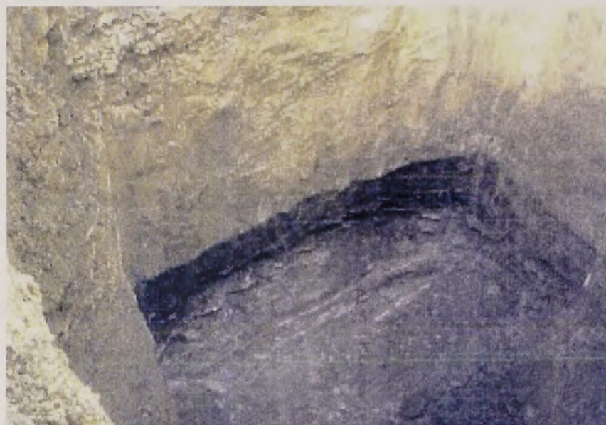
Figure 2.3-8. Excavation of Tower Foundation Hole Following Blasting.
