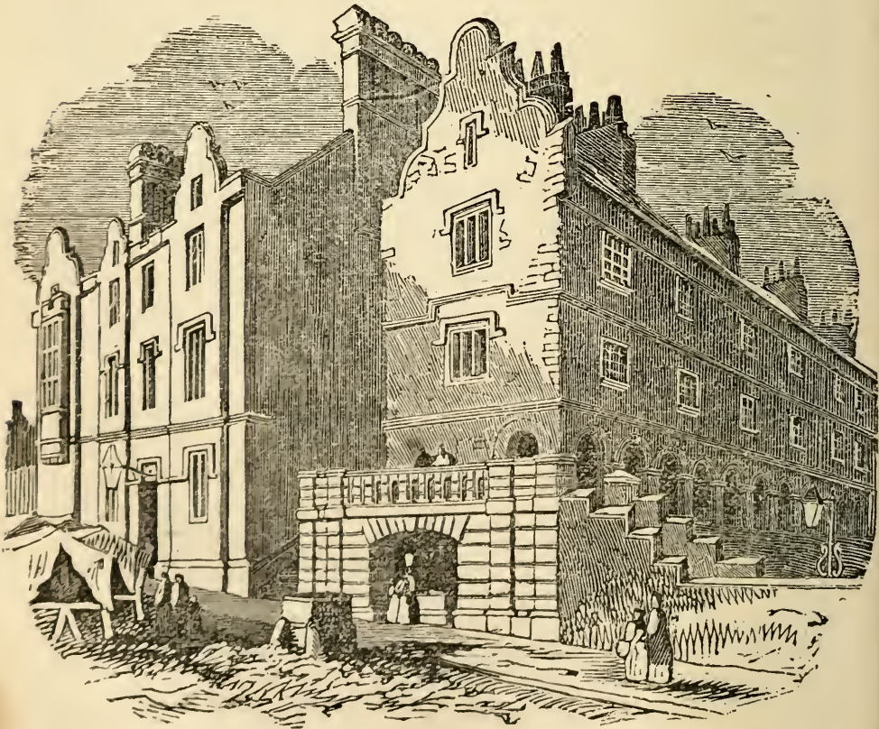
POLICE STATION, MANORS, AND FREEMEN'S HOSPITAL.
