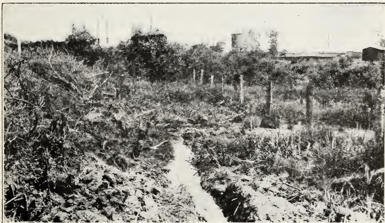
FIG. 22.—SEEPAGE INTERCEPTION, TOE AT FISH POND EMBANKMENT, CROSSETT.
