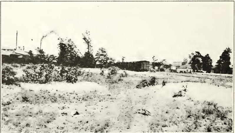
FIG. 20.—SAME BORROW PIT SHOWN IN FIG. 19, AFTER TREATMENT BY FILLING.
