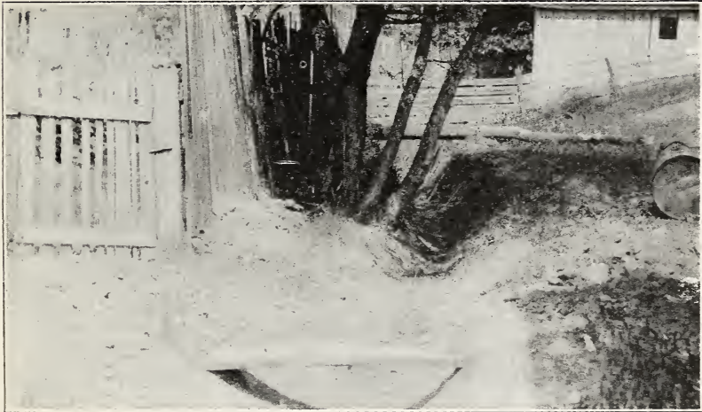
FIG. 14.—SAME DITCH AS SHOWN IN FIG. 13, AFTER CLEARING.
