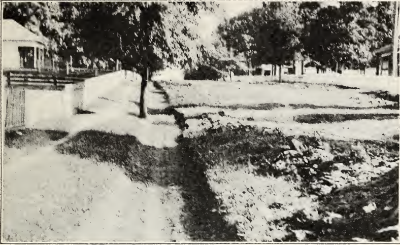
FIG. 9.—STREET DITCHING, CROSSETT.
