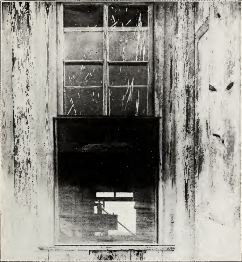
FIG. 28.—TYPE OF WINDOW SCREENING INSTALLED, HOUSES OF GROUPS "A" AND "C."
