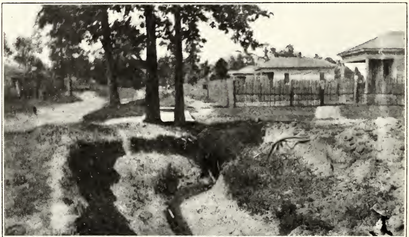
FIG. 12.—SAME STREAM AS IN FIG. 11, SHOWING RECHANNELING.
