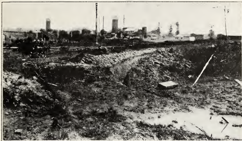
FIG. 21.—DRAINING A BORROW PIT.
