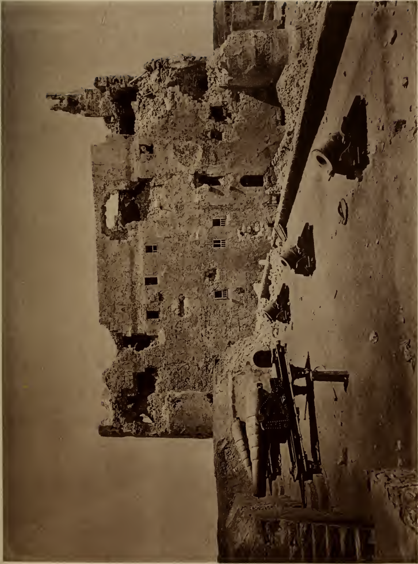
FORT PHAROS. 8 IN. GUN BATTERY. CONDITION OF WEST FACE OF KEEP AFTER BOMBARDMENT.
