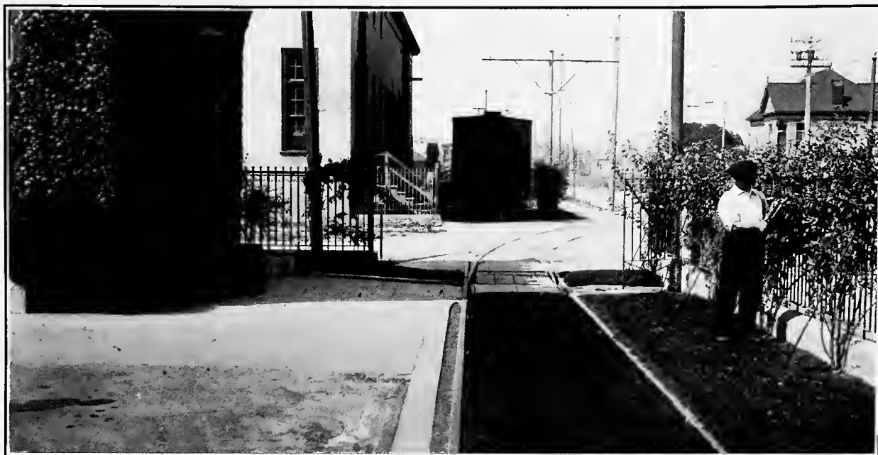
ELECTRIC SPUR TRACK OF OAKLAND FACTORY
