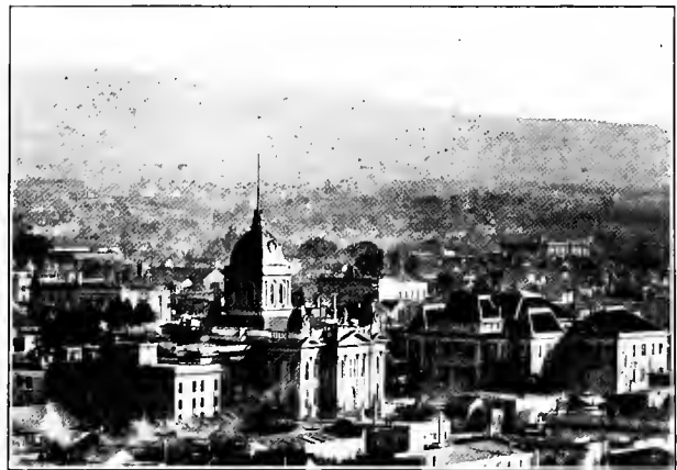
EARLY ATTEMPT IN OAKLAND AT GROUPING PUBLIC BUILDINGS
