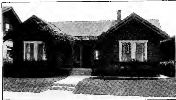
INEXPENSIVE EAST BAY RUNGALOWS. COST ABOUT $2500 EACH. MATERIAL (UPPER PICTURE), PLASTER; (LOWER PICTURE), WOOD
