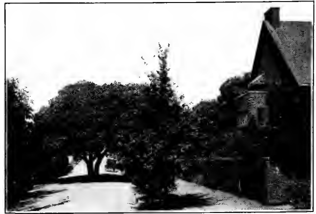
LEROY AVENUE NEAR RIDGE ROAD, BERKELEY EXAMPLE OF "GOOD OUTGOINGS"
