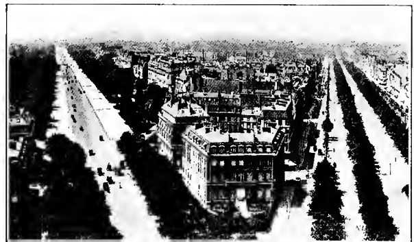
SUCCESSFUL TREATMENT OF A CORNER
