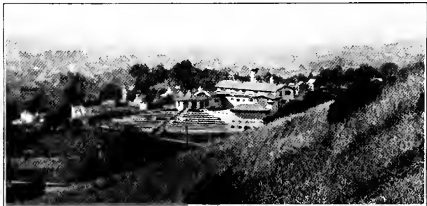
VIEWS OF THE TERRACES AND NEIGHBORHOOD OF THE SAME HOUSE
