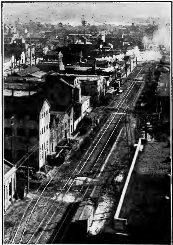
UNDEVELOPED TRACKAGE OF SOUTHERN PACIFIC RAILROAD, FIRST STREET, OAKLAND
