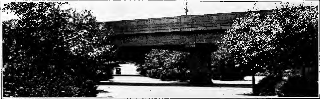
ELEVATED RAPID TRANSIT LINE OVER PARKWAY AT FOREST HILLS, BOSTON
