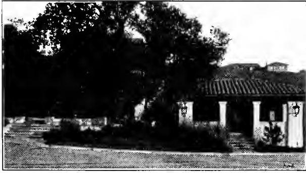
PLEASANT APPROACHES AND "GOOD OUTGOINGS," NORTHBRAE STATION, BERKELEY
