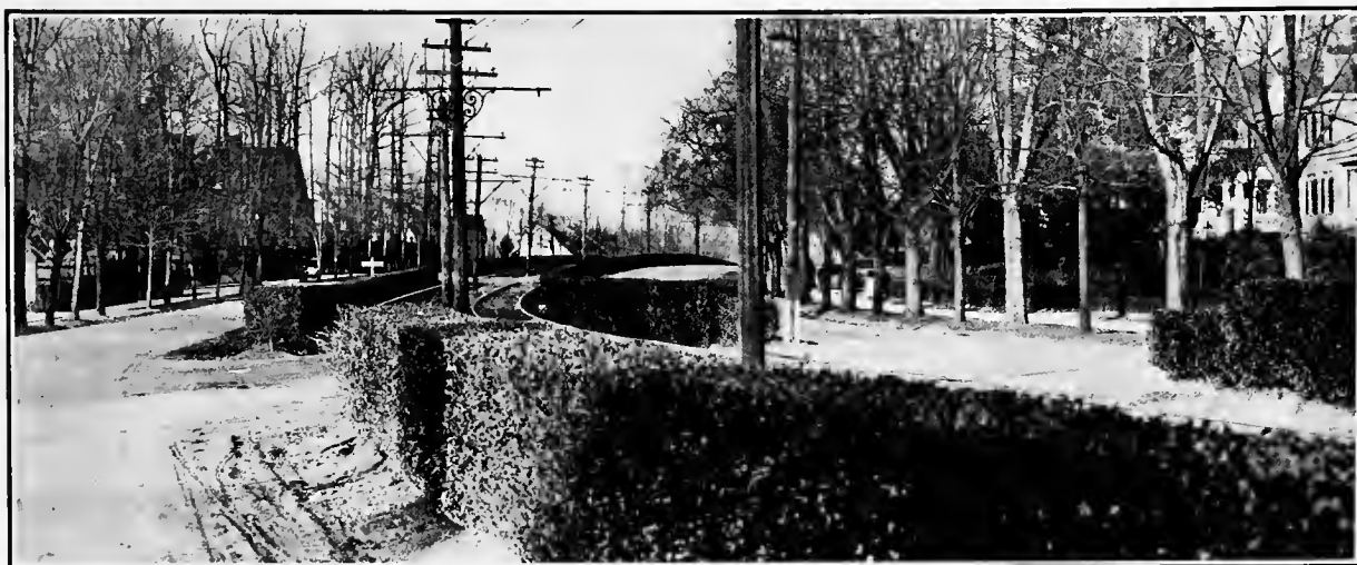
PROPER PLANTING ACHIEVED
