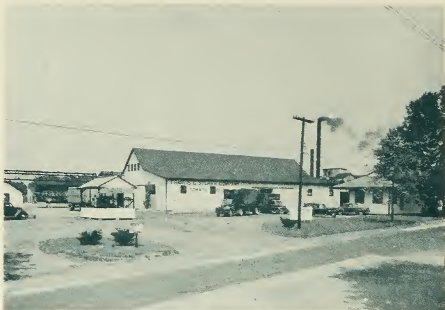
The Stokes establishment at Vincentown, New Jersey.
