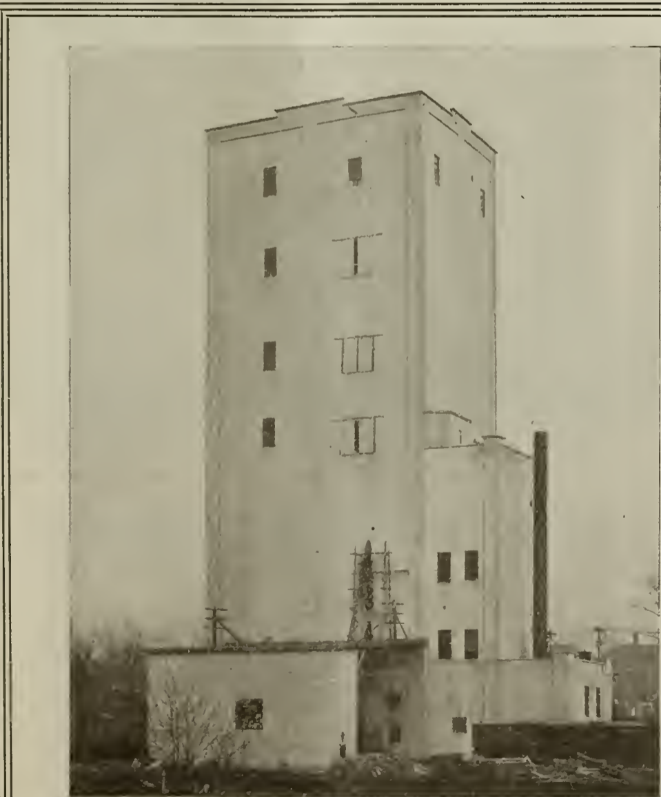
Constructed by us for Dewein-Hamman Co., Decatur, Ill. For full description see page 621 of this assue.
