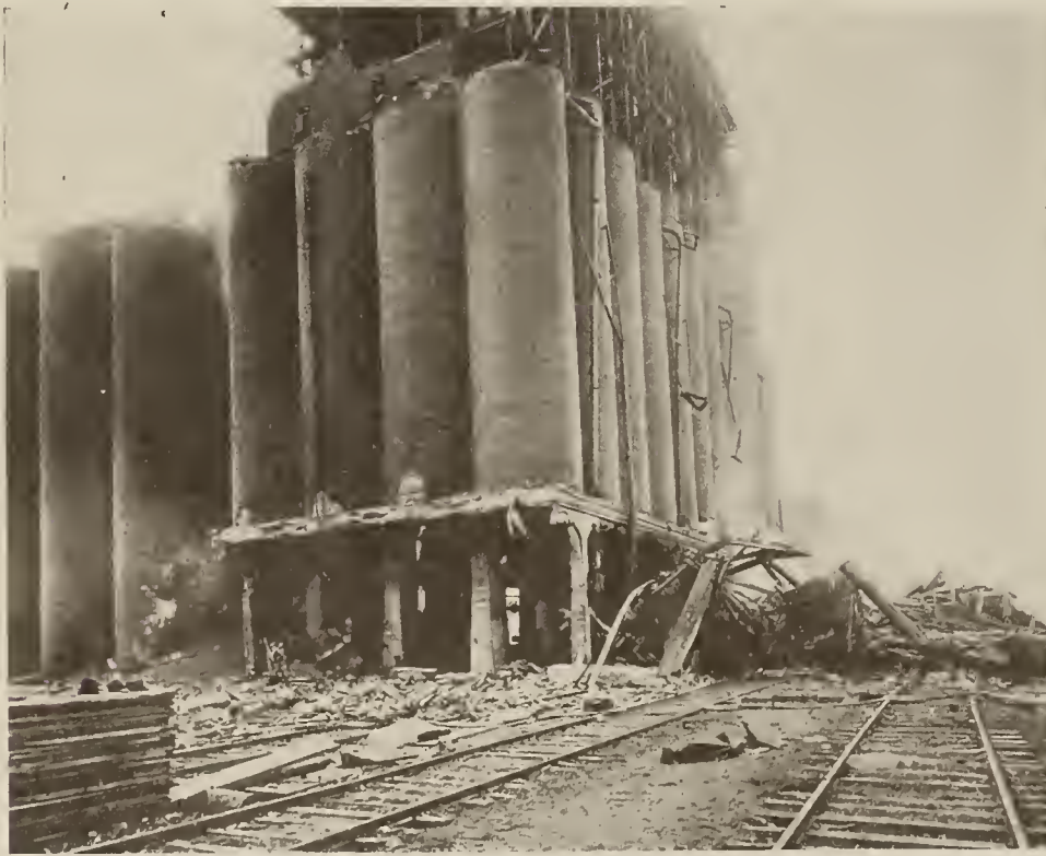
VIEW OF NORTHWESTERN PORTION OF THE PLANT Destruction of working shed and railroad cars is shown at the right
