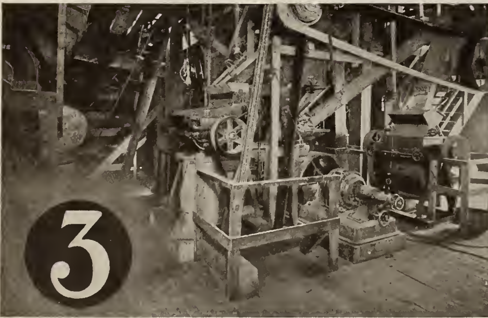
Separating and Grinding Room
