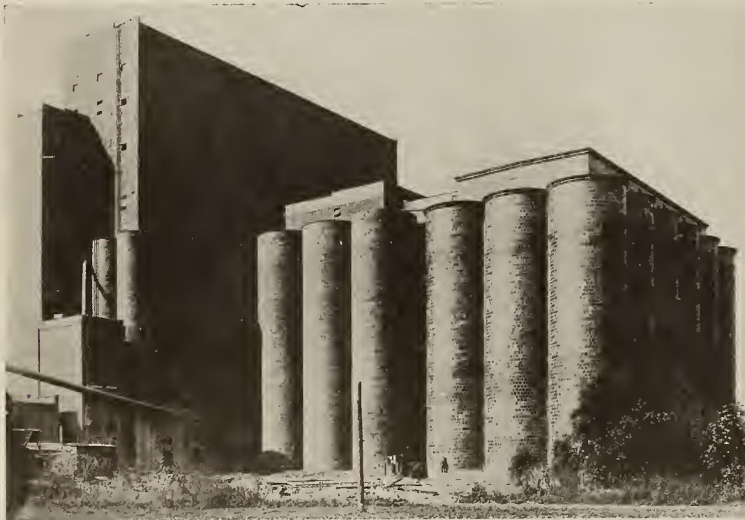
VIEW OF THE ELEVATOR BEFORE THE EXPLOSION
