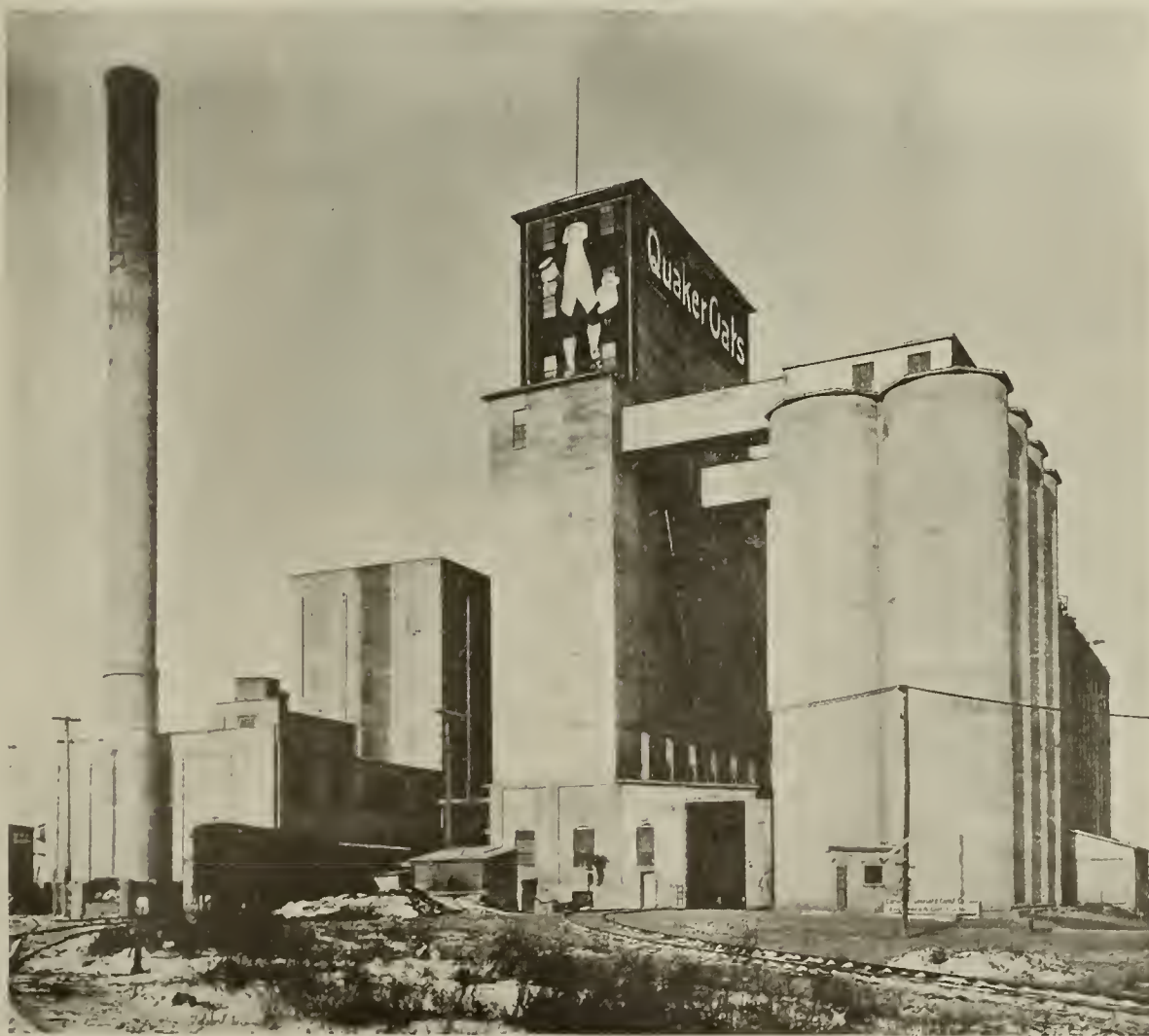
NEW QUAKER OATS ELEVATOR AT SASKATOON, SASK.
