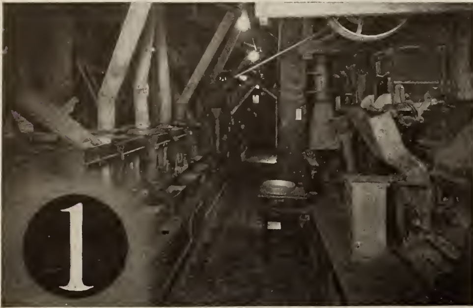
A Few of the 76 Feeders in the Mixing Room
