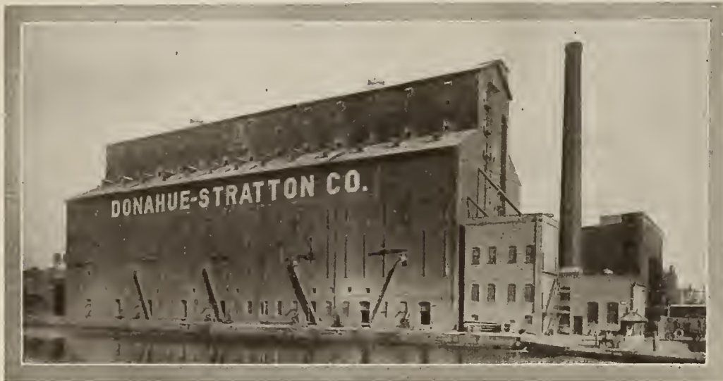
THE DONAHUE-STRATTON ELEVATOR, MILWAUKEE Destroyed by fire on January 25
