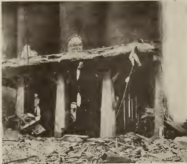
NORTH END OF WORKING FLOOR
