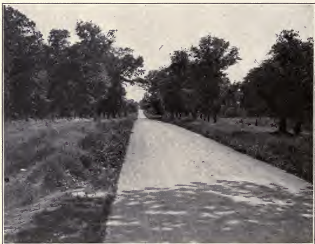
CONCRETE ROAD LEADING TO PRESERVE.
