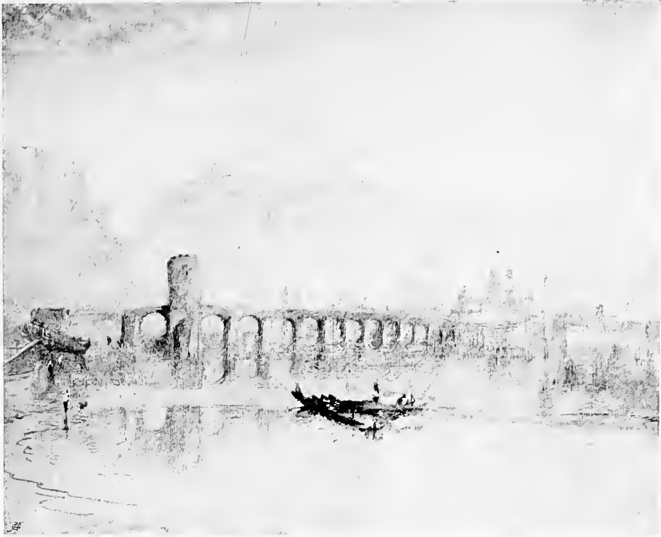
COBLENTZ: BRIDGE ON THE MOSELLE
