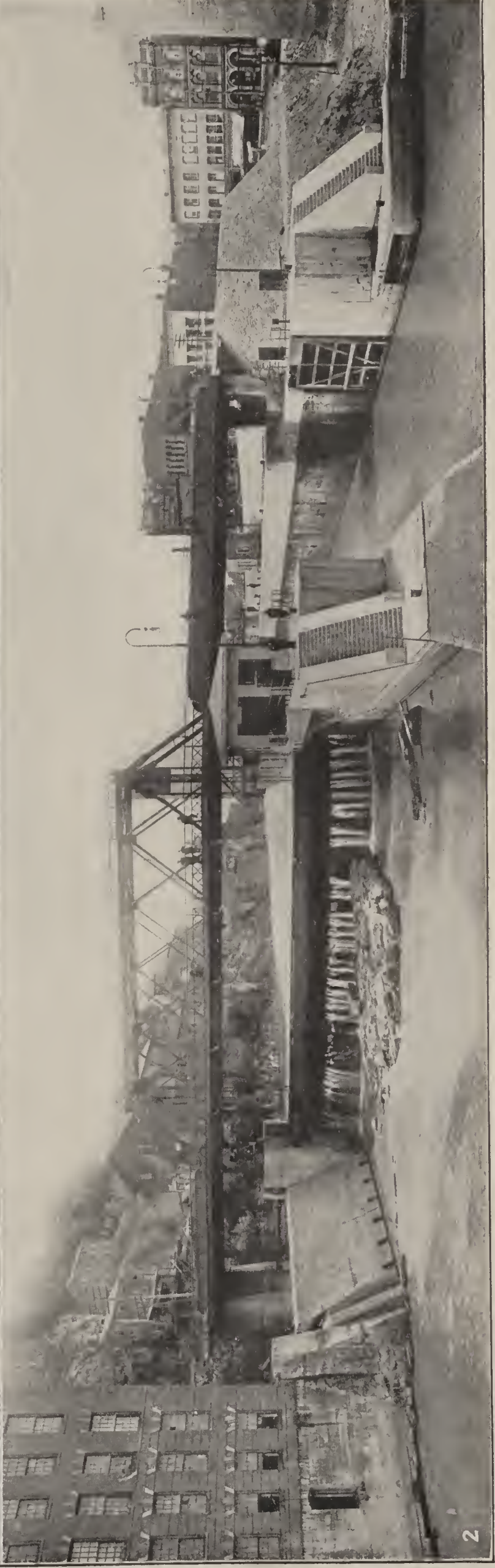
1. DAM AT MECHANICSVILLE Here the Hudson River has been canalized by using an existing dam. A portion has been cut away and the lock seen on the right built. 2. ENTRANCE OF CHAMPLAIN CANAL INTO LAKE CHAMPLAIN. View at Whitehall, showing a siphon spillway on the left, dam in the centre with movable crest of Taintor gate type operated from highway bridge, and regulating Wood Creek and lock No. 12 with its power house on the right.
