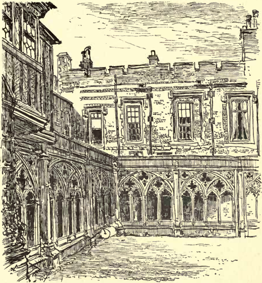
THE CLOISTERS AND THE DEANERY.
