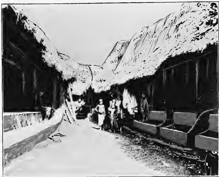
The part of a Bini house called ODERIE, marked No. 15 on Plan. See page 189
