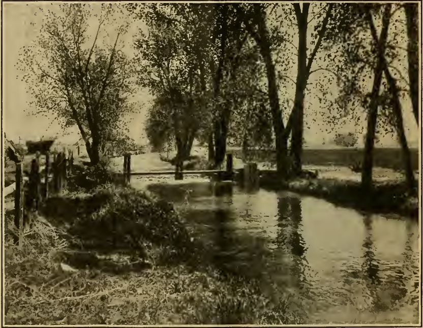
FIG. 3.—Irrigation canal No. 2 in the Greeley district.
