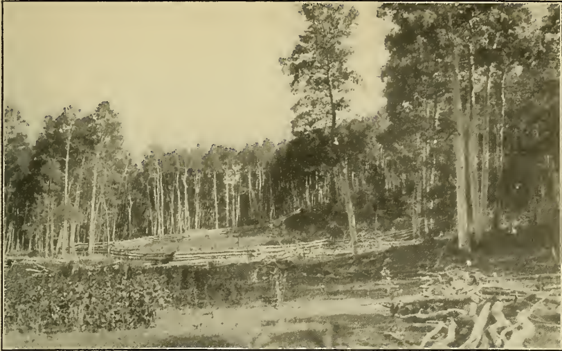
FIG. 1.—CLEAR-CUT PROTECTED ASPEN AREA ON SHEEP RANGE AS IT APPEARED AFTER FENCING IN THE SPRING, 1913.
