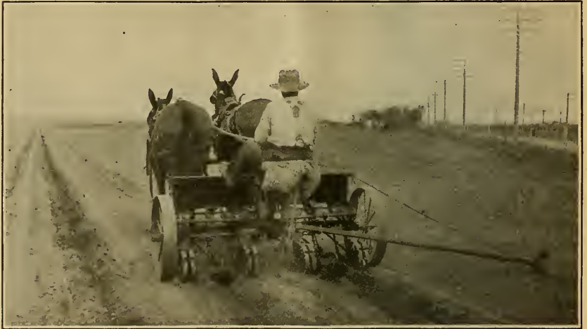
FIG. 11.—Planting beet seed with a four-row beet drill. The marker to the right makes a line that serves as a guide for the driver. Furrowing-out shovels are also attached to this beet drill.
