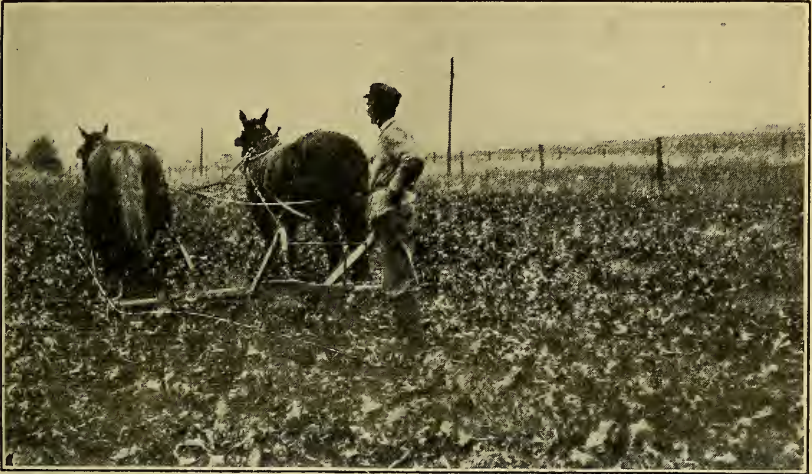
FIG. 19.—Harvesting beets with a lifter. The points of the crotch lifter run on either side of the row.
