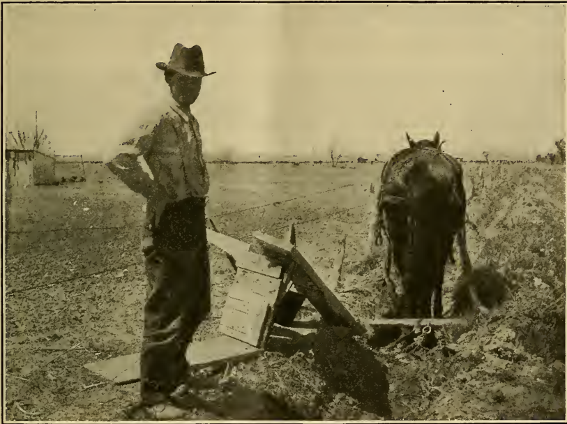
FIG. 10.—Removing silt and other débris with a homemade V ditcher. It will be seen that the deposit of silt was first loosened with a plow.
