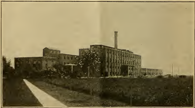
FIG. 2.—One of the beet-sugar factories in northeastern Colorado. This plant, constructed in 1905, has a rated capacity of practically 1,000 tons daily.
