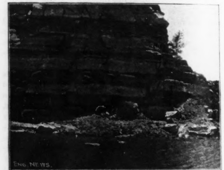
Fig. 3.—Quarry from which Limestone for Center of Austin Dam was Taken.
