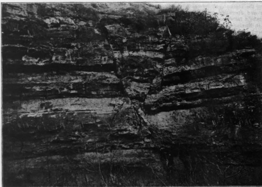
FIG. 2.—VIEW SHOWING FAULTY NATURE OF LIMESTONE ROCK AT THE SITE OF THE AUSTIN DAM.
