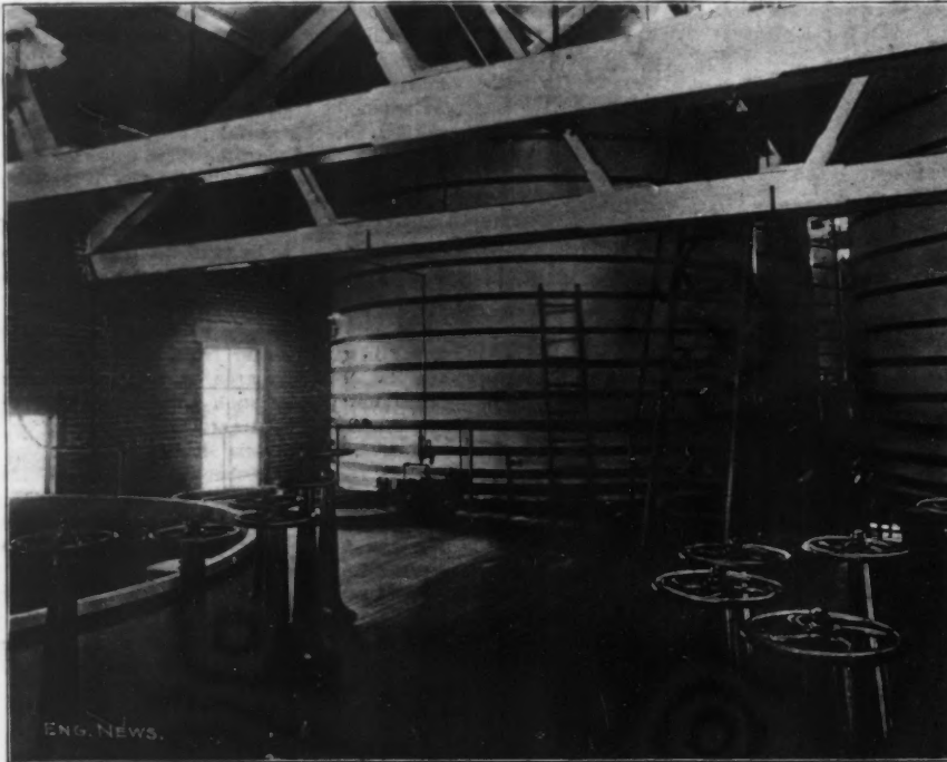
FIG. 2.—VIEW OF FILTERS, SETTLING TANKS AND ACCESSORIES.
