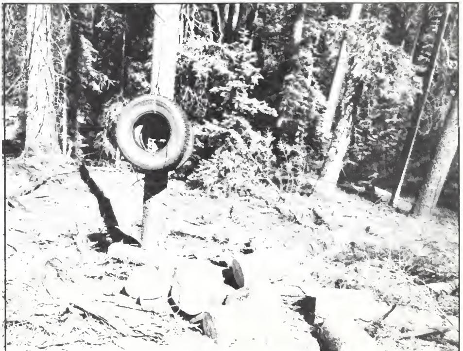
A staple puller (top) or tires (bottom) can be used to keep firewood blocks from hitting the lower spar tree.
