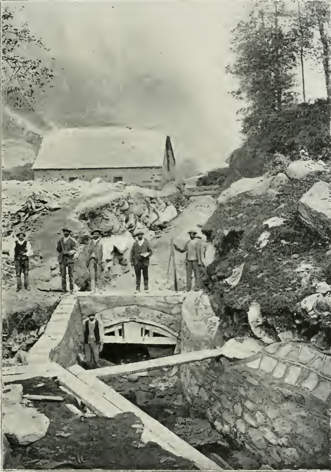
Fig. 314.—Pierrefitte Electric Power Station : Construction of Intake Canal.
