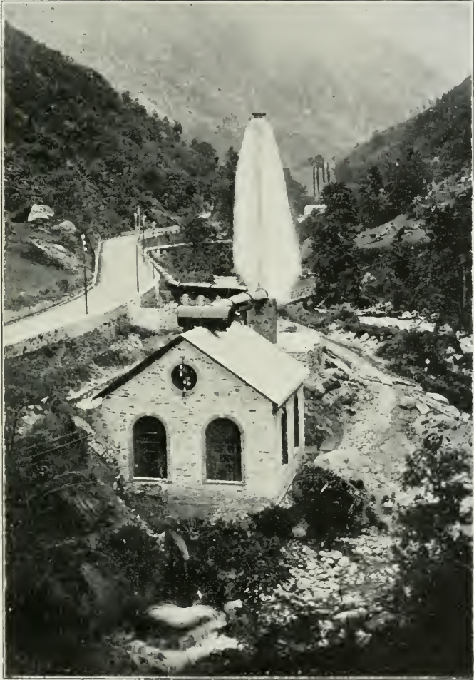
Fig. 317.—Pierrefitte Electric Power Station: Safety-valve in Operation.
