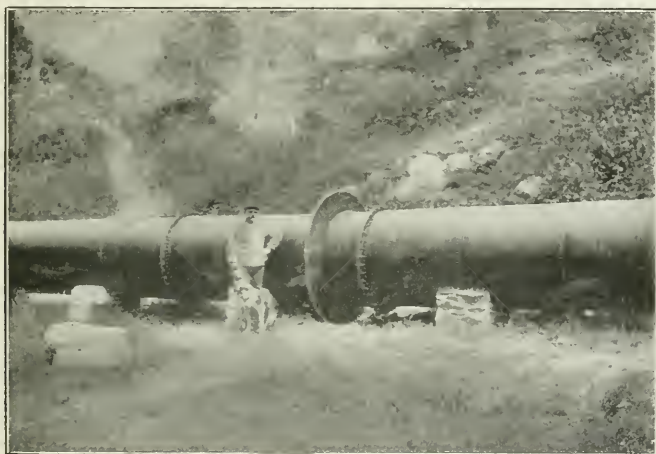
FIG. 315.—EXPANSION JOINT ON PIPE LINE.
