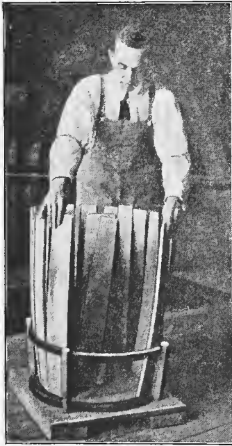
Fig. 38.—FORM FOR SETTING UP A BARREL
