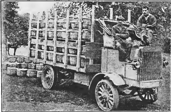
Fig. 107.—EFFICIENT TRANSPORTATION ON GOOD ROADS FOR 15 OR 20 MILES
