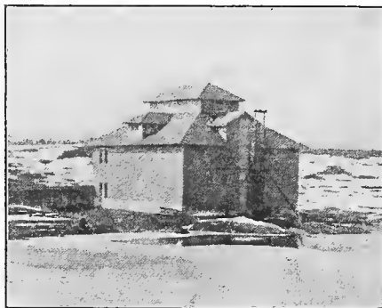
Fig. 79.—LOCAL COLD STORAGE
