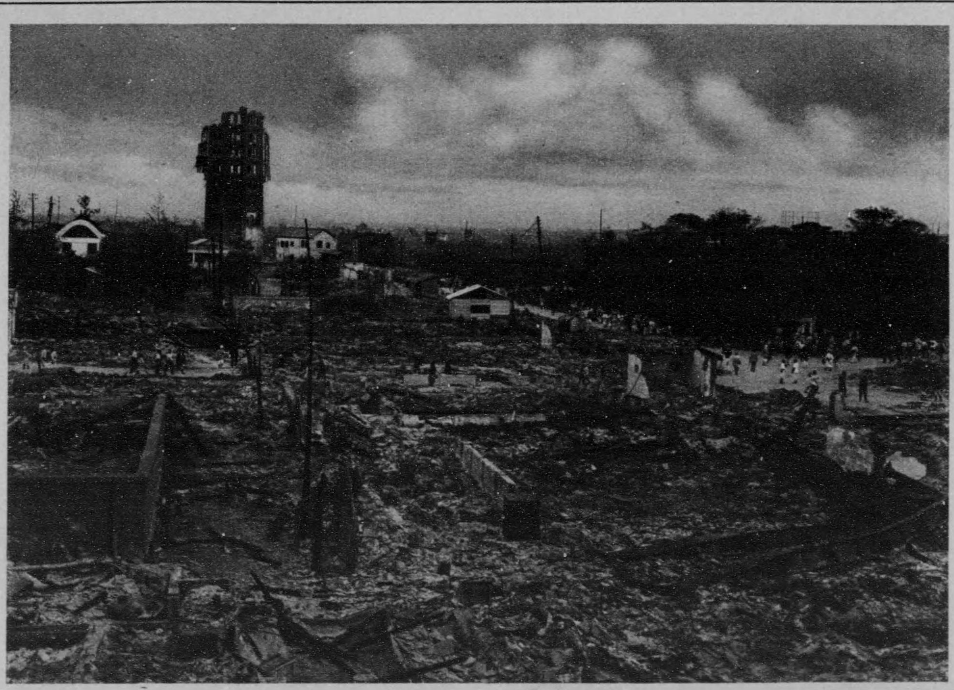
Damages at Asakusa, the remains of theatres and the 12 storied tower which was broken down from nine stairs.
