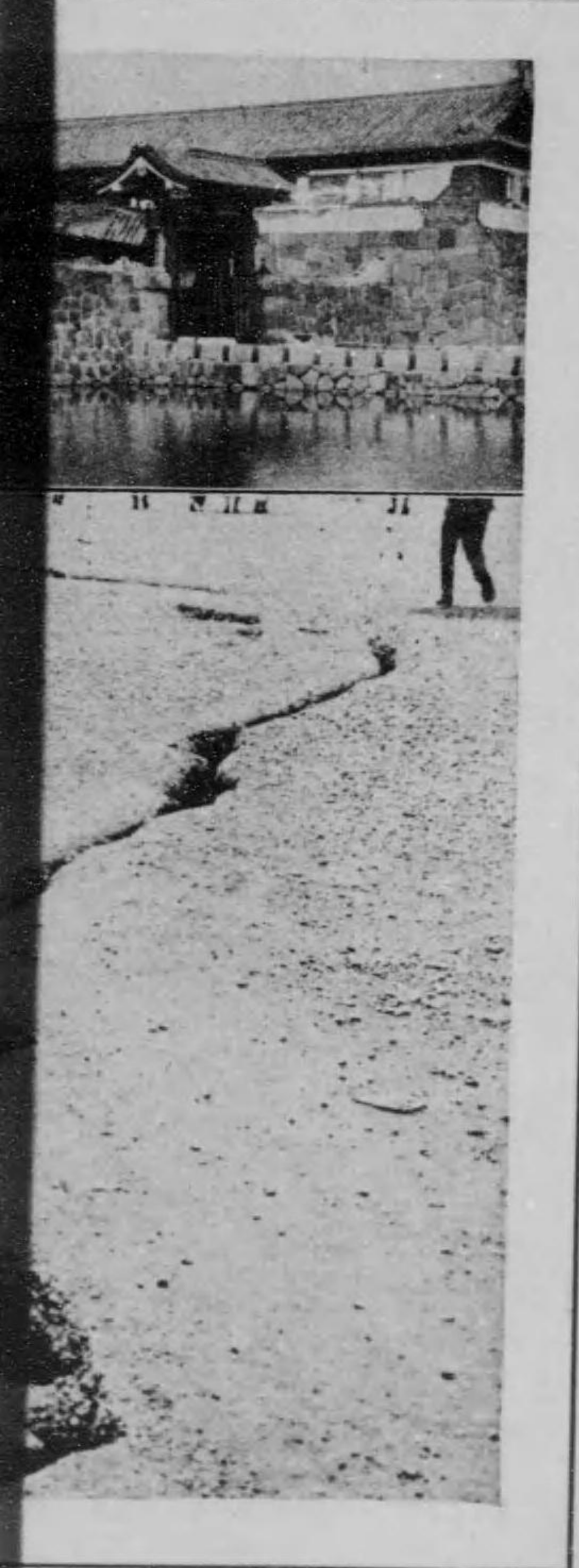
Damage of Ote
