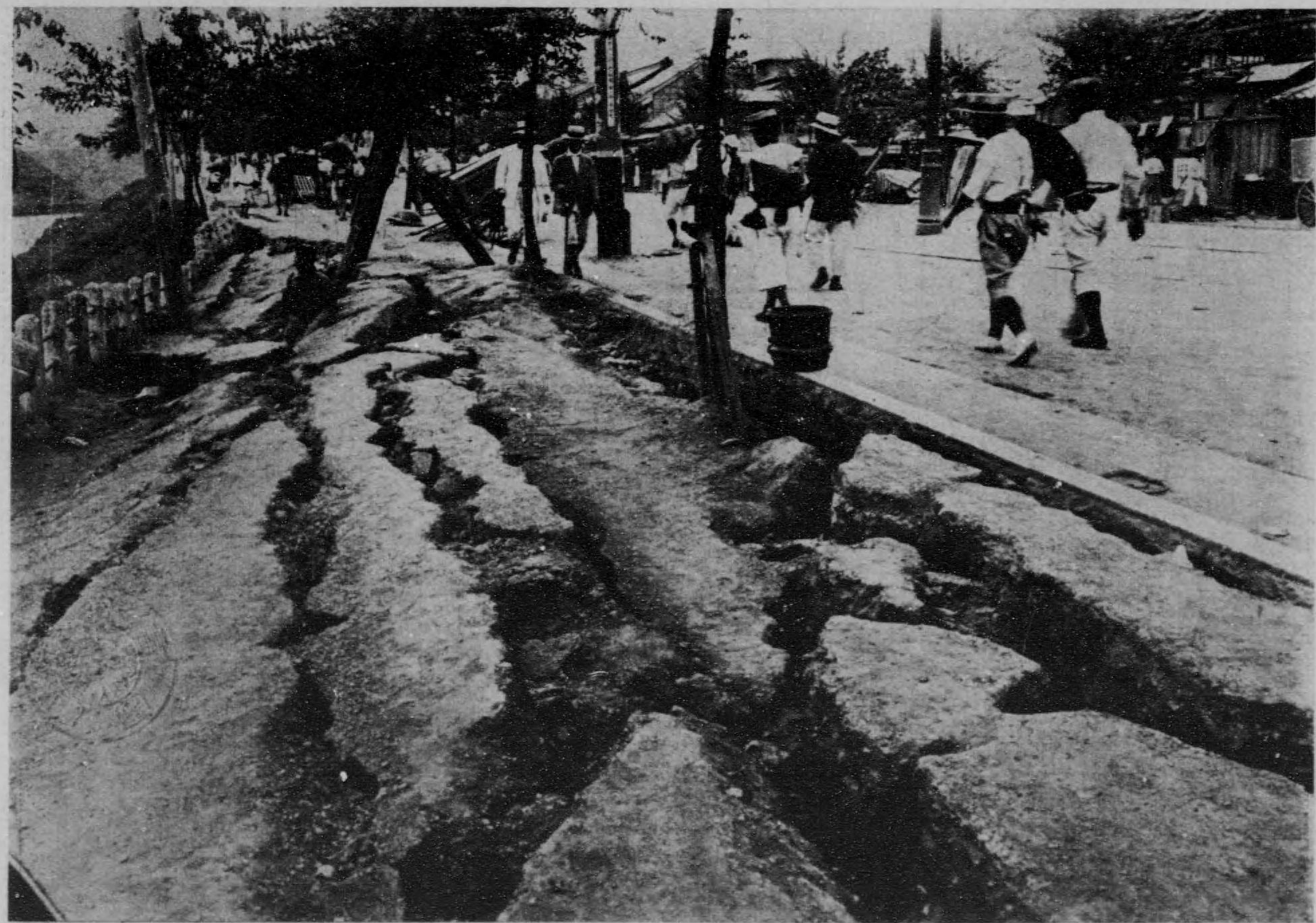
Fissures on the road at Ichigayamitsuke. Note the depth of it comparing with a man.
