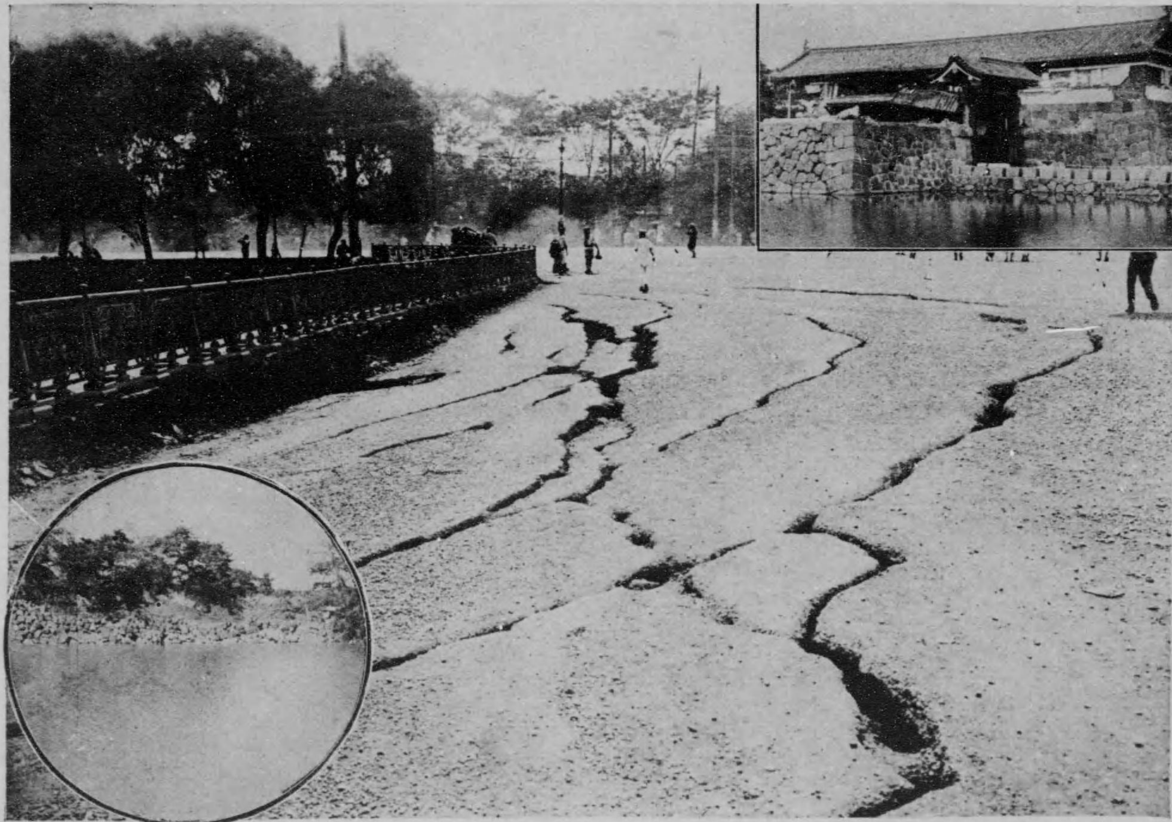
Damages around the Imperial Palace; Upper ; Fissure in front of Sakurada gate. Middle ; Damage of Ote gate. Lower ; Stone wall facing the Palace crumbled.
