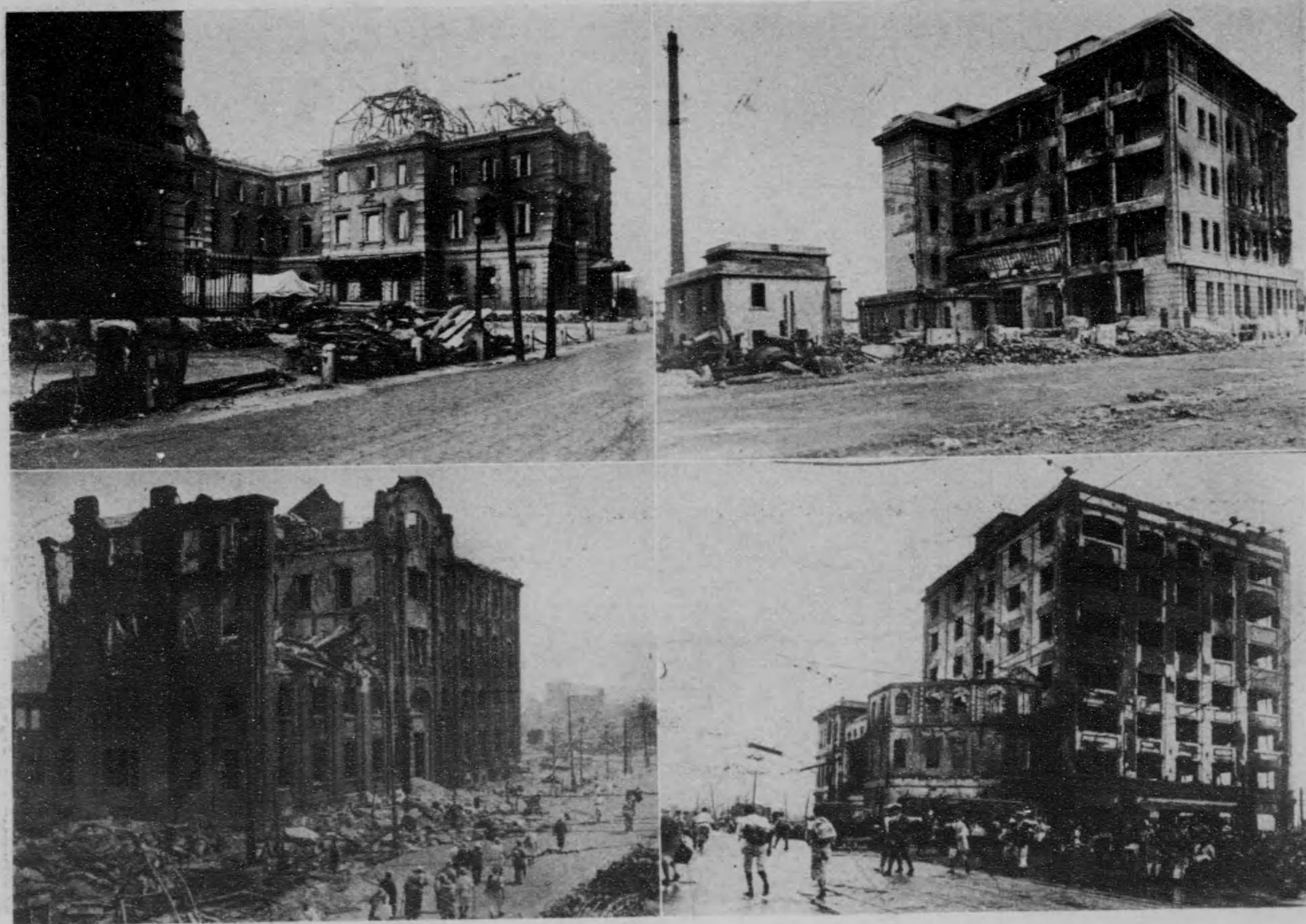
Damages of four big buildings. Upper right: branch of the Bank of Korea. Kojimachi. Lower right: Hoshi pharmaceutical Company at Kyobashi junction. Upper left, Mitsui Bank. Lower left: Takata Shekai, one of the noted Trading company.
