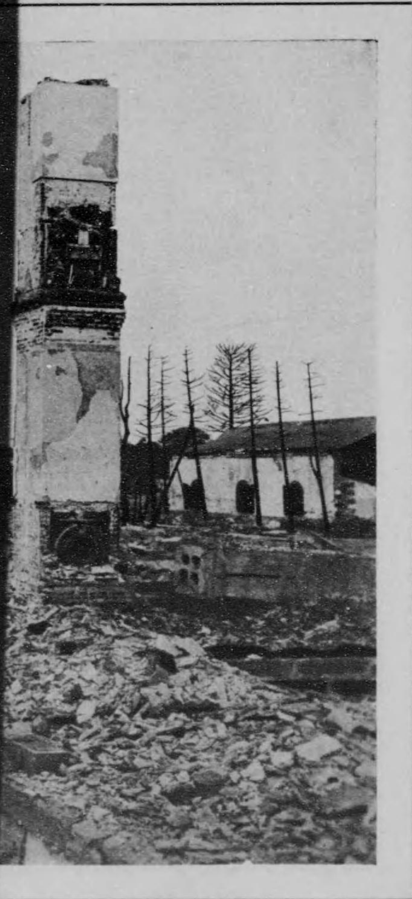
here was a innumerable damage
