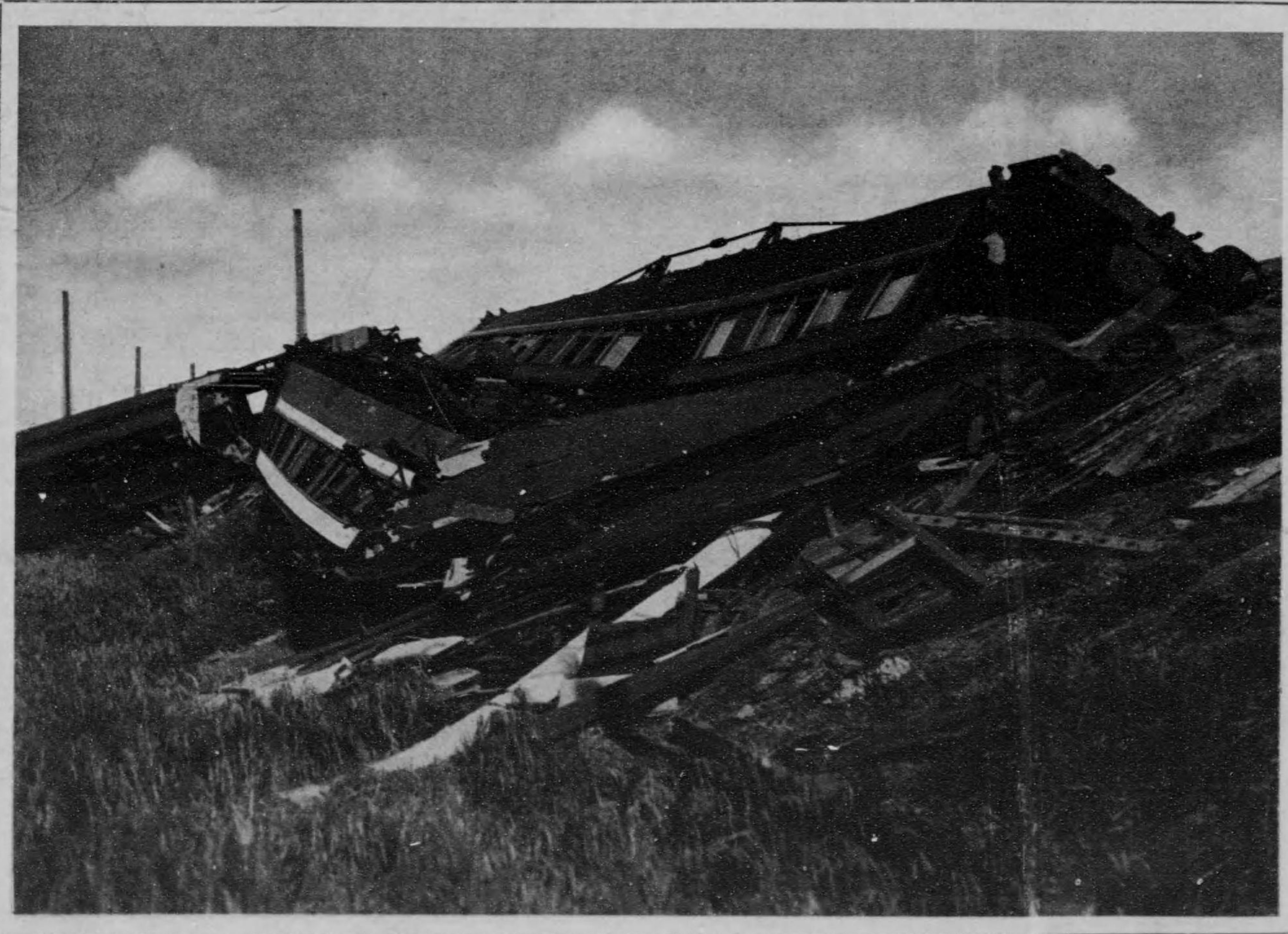
Overturnd train on the Tokaido line. Twenty-four trains were met with a similar fate.
