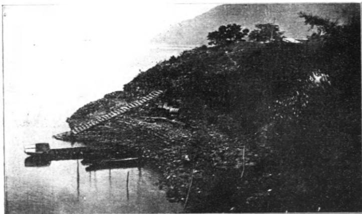
The picture shows a part of an old dyke projecting far into the river thus causing eddies etc. injurious to the dyke. An example of how a dyke should not be constructed.
