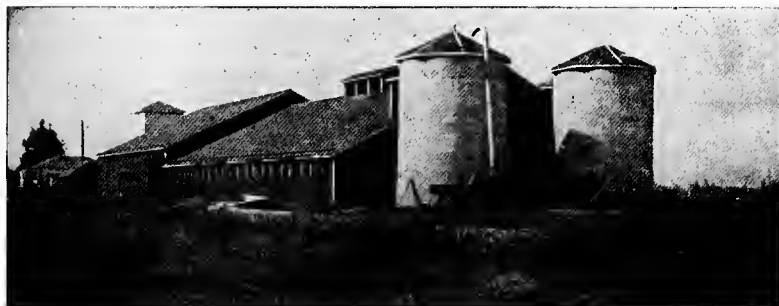
FIG. 29.—A California dairy barn, with concrete silos, accommodating four rows of cows, with a driveway in the middle.
