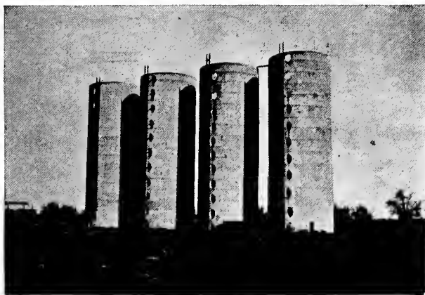
FIG. 31.—Battery of four cement silos on a California cattle ranch. Dimensions 20 feet in diameter, and 46 feet high, capacity about 350 tons each. ( Pacific Rural Press )
