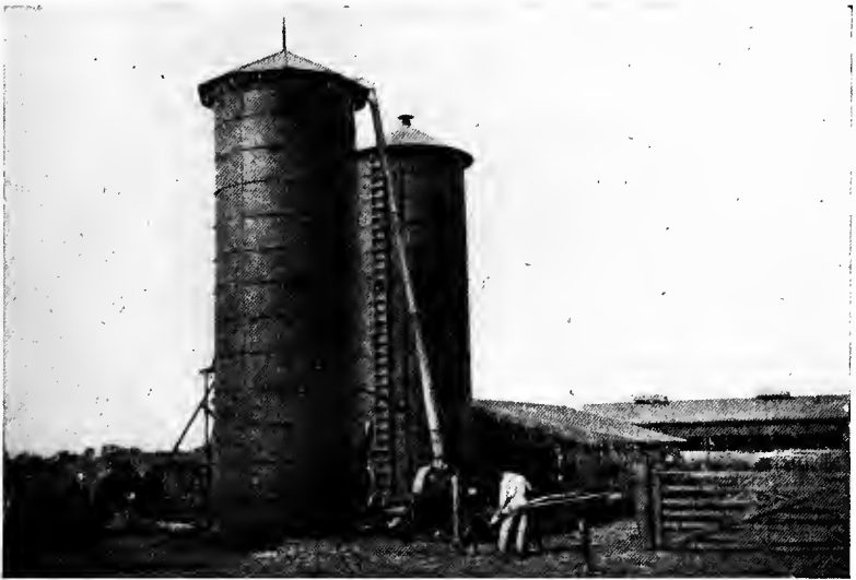
FIG. 27.—Stave silos. Dimensions, 12 feet in diameter, 36 feet high, capacity 84 tons.
