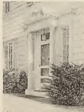
A Very Effective Door Entrance Planting
