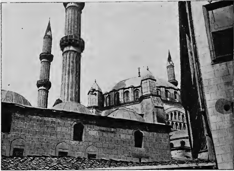
FIG. 15.—MOSQUE OF SULTAN SELIM A CUPOLA OF THE DOME RENT BY AN EXPLOSIVE SHELL
