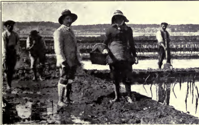
FIG. 20. Arcachon, France. Oyster parks with low clay walls. Water is retained in those at the right at the low tide, that at the left being emptied for repairs.
