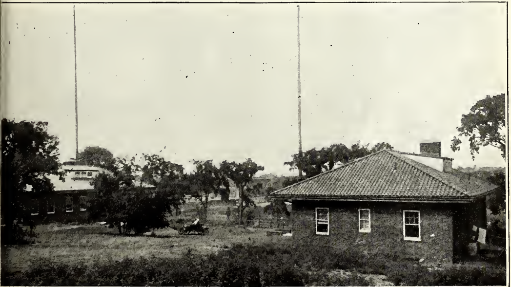
THE STATION OF THE TRANSATLANTIC WIRELESS TELEPHONE, NEW BRUNSWICK, NEW JERSEY
