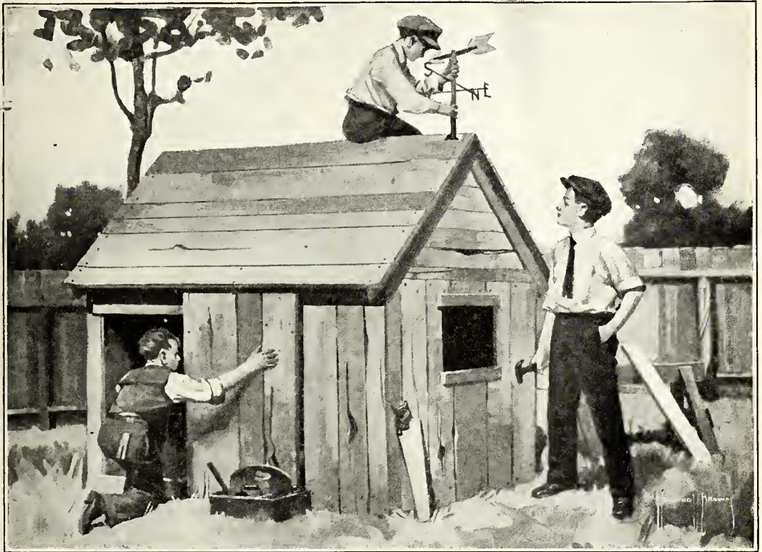
HARD AT WORK ON THE "BARN," OR FIRST BUILDING, IN PACKING-BOX VILLAGE
