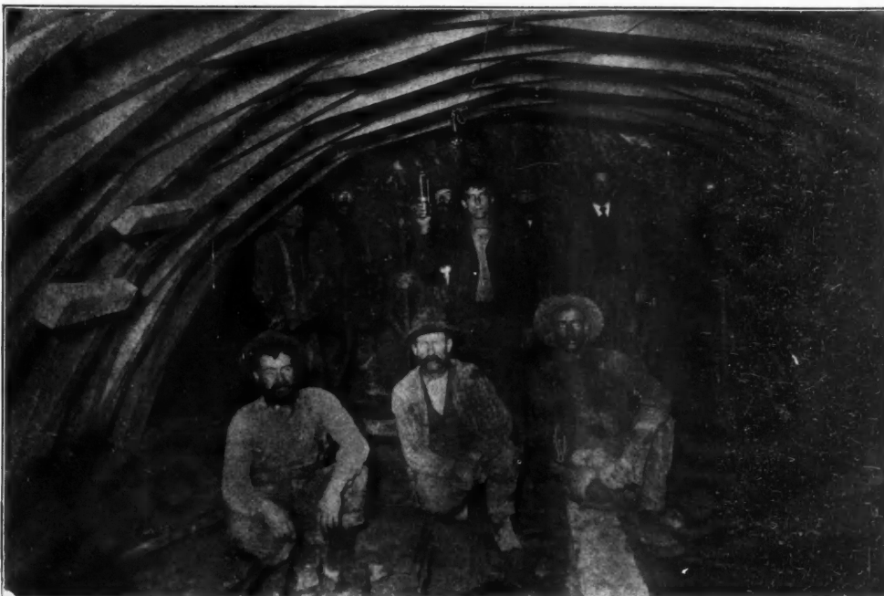
DRILLING IN ASPEN TUNNEL.
