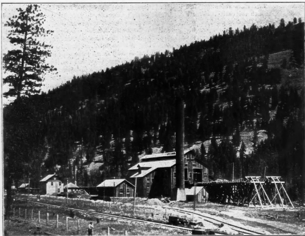
MONTREAL AND BOSTON COPPER CO.'S SMELTER NEAR BOUNDARY FALLS, B. C.
