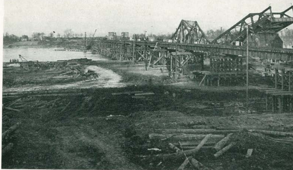
U. S. Army Railroad Bridge over the Rhine at Wesel, Germany
