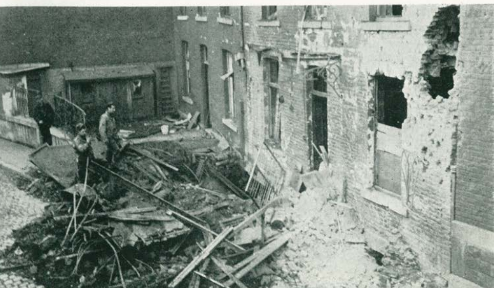
Damage from 100-pound Aerial bomb, 708th Headquarters, Liege, Belgium
