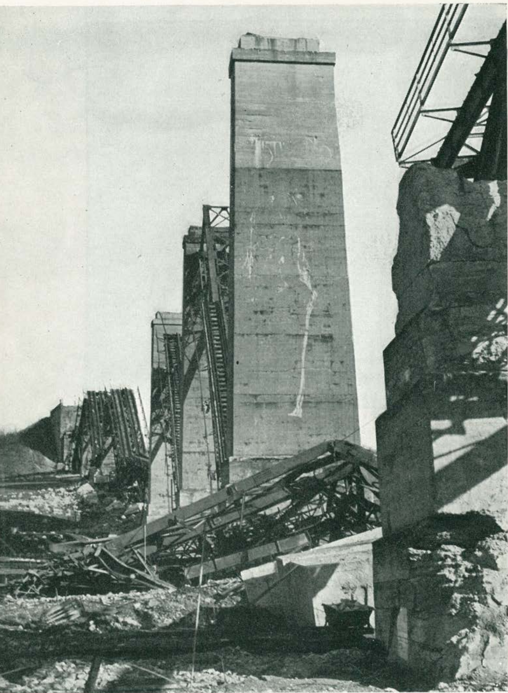
Destroyed Railroad Bridge, Montzen, Belgium
