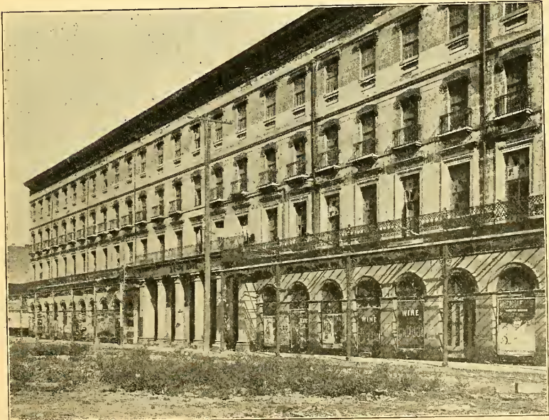
Old Hotel Royal, recently demolished —See Page 37.
