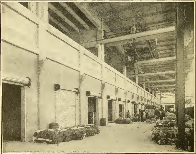
Interior View of Cotton Warehouse.
