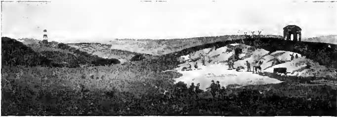
Fig. 7. View from Wentworth House, before it was improved, and while the improvements were going forward.
