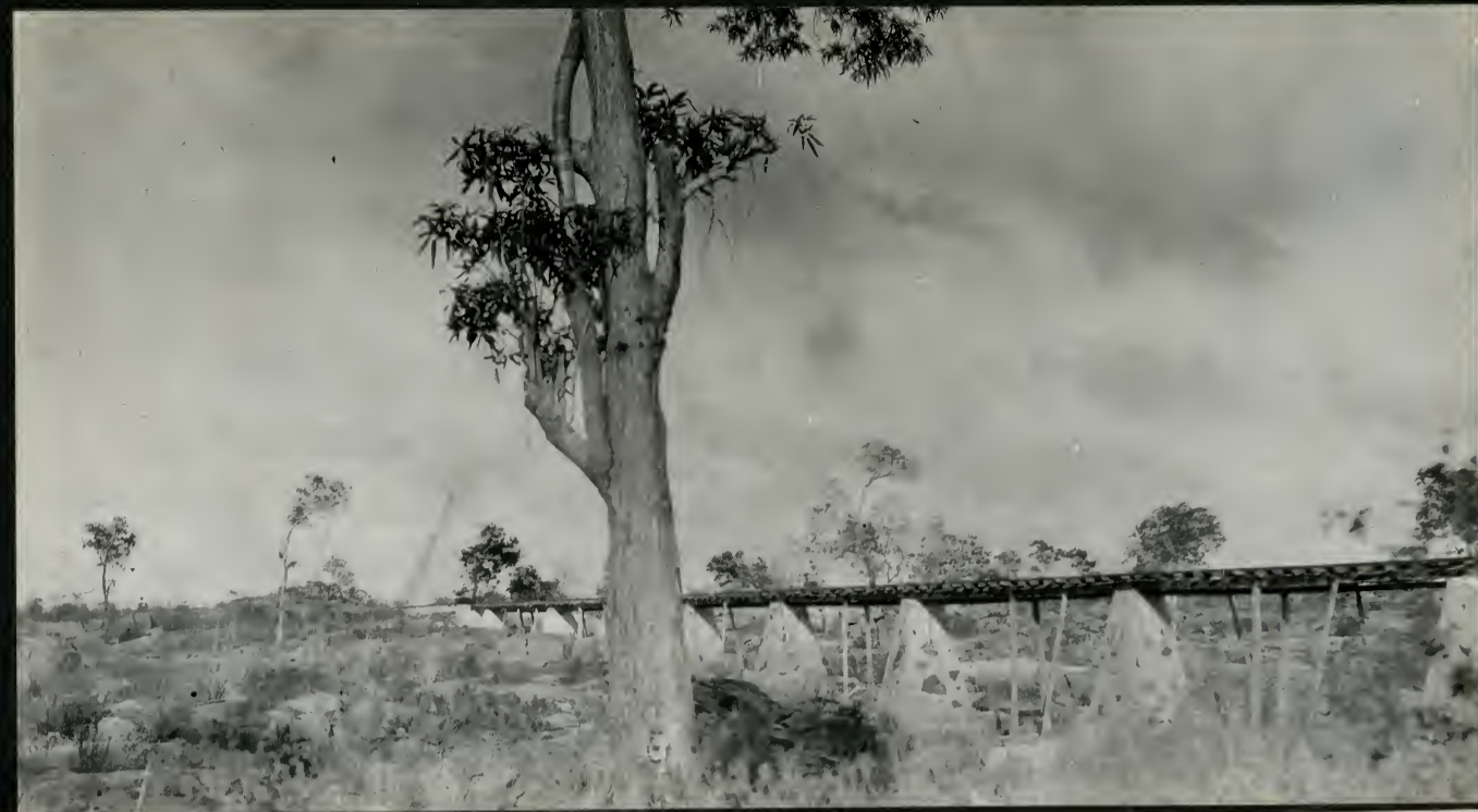
1781. Region of Paulo Affonso falls, Alagoas showing trestle approach to falls.
