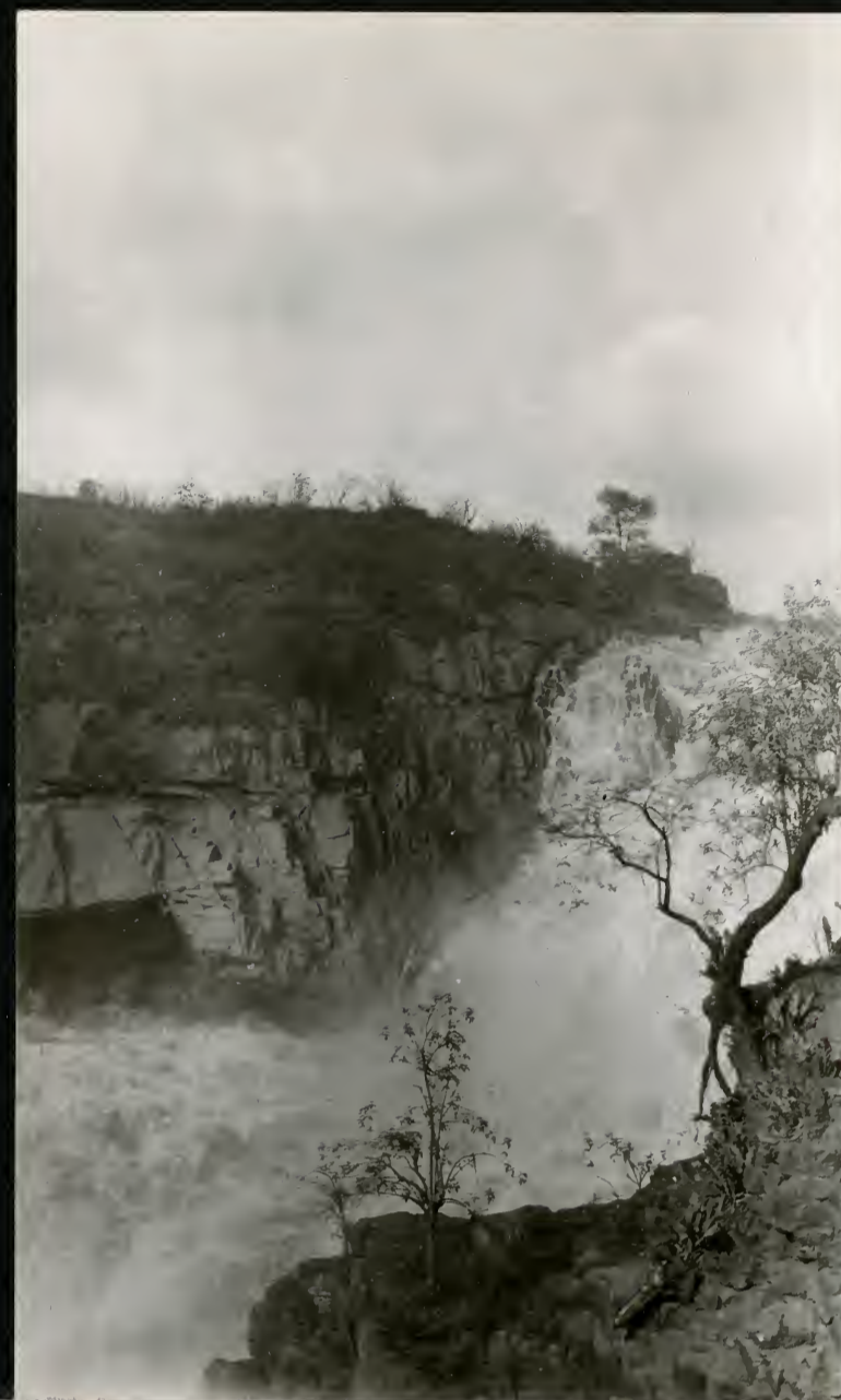
1806. Paulo Affonso falls from turbine station.
