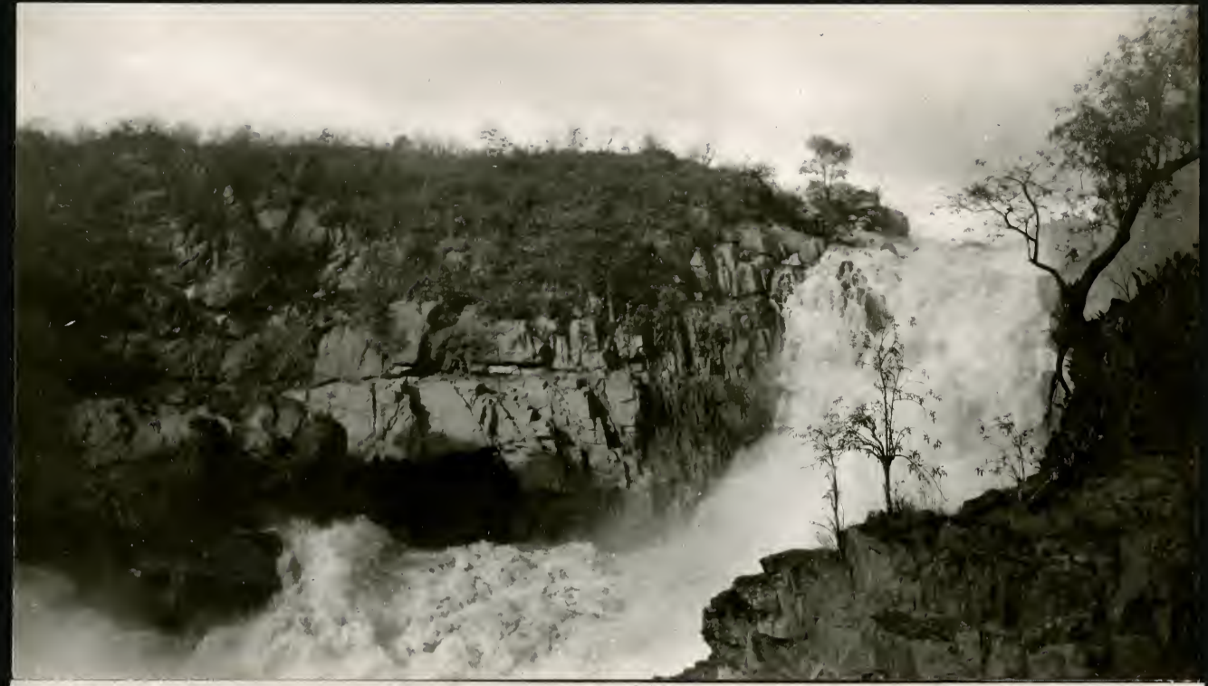
1794. Paulo Affonso falls from turbine station.
