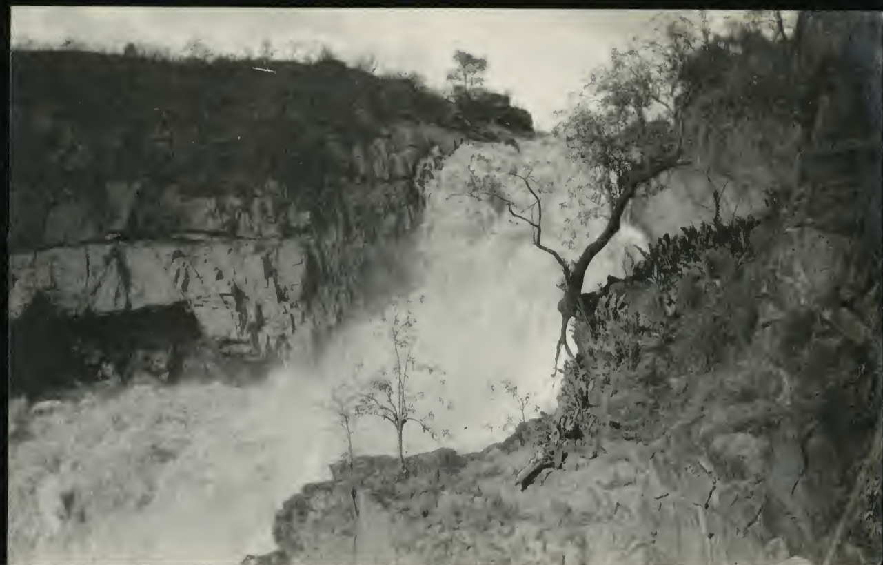
1801. Paulo Affonso falls from turbine station.
