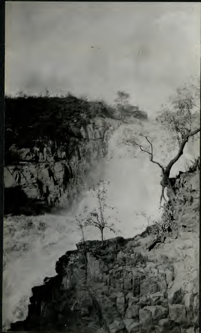
1802. Paulo Affonso falls from turbine station.
