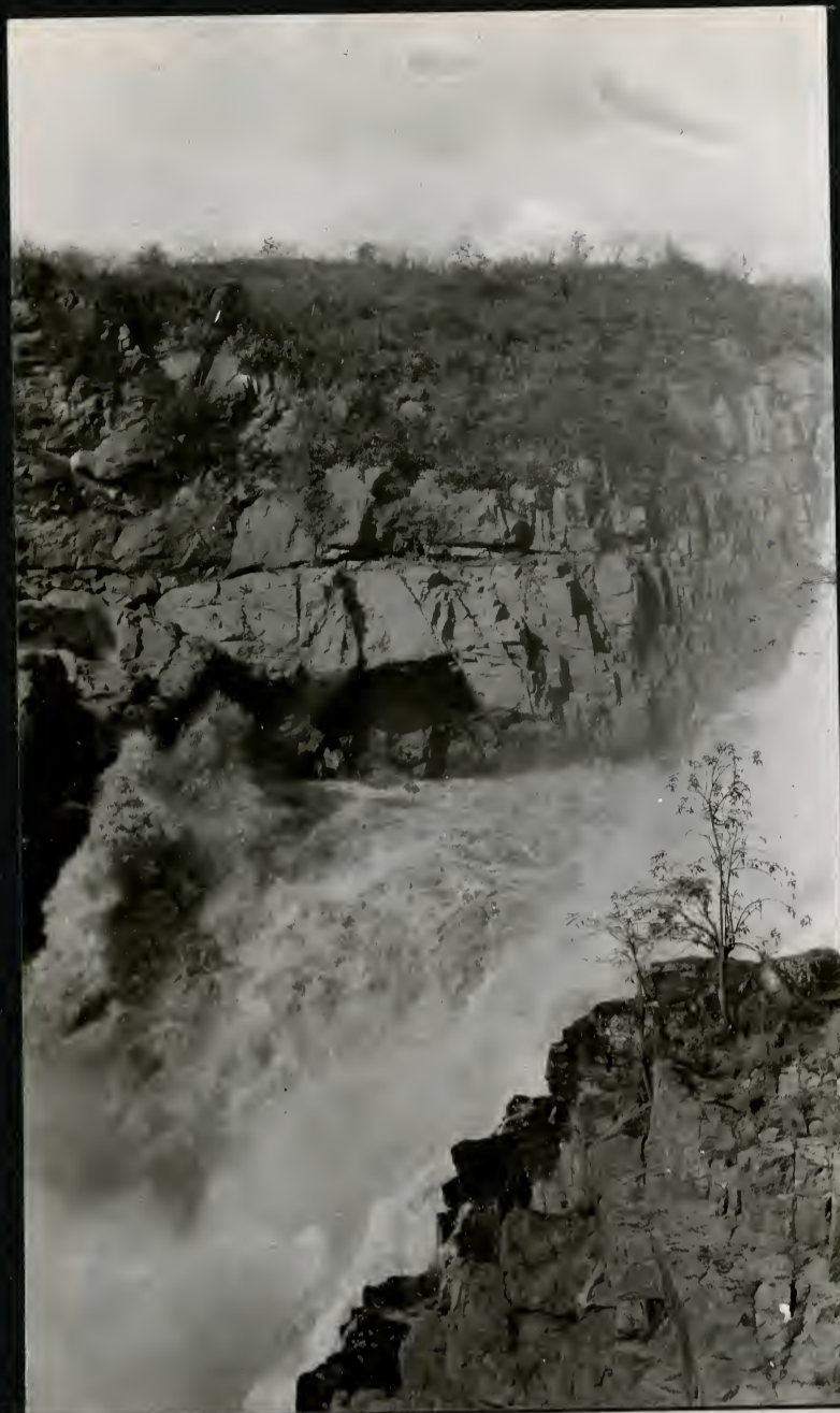
1804. Paulo Affonso falls from turbine station.
