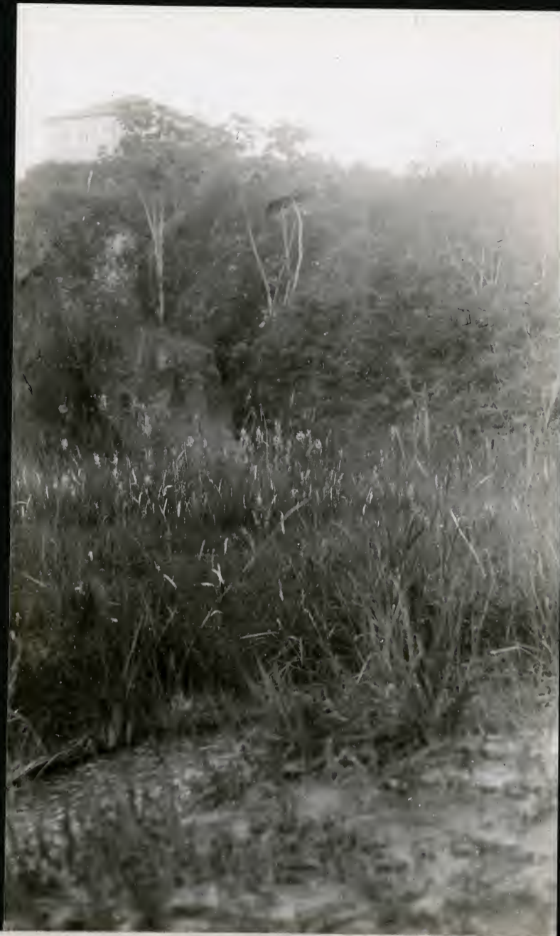
1869. Lavras, showing erosion in red clay hills.
