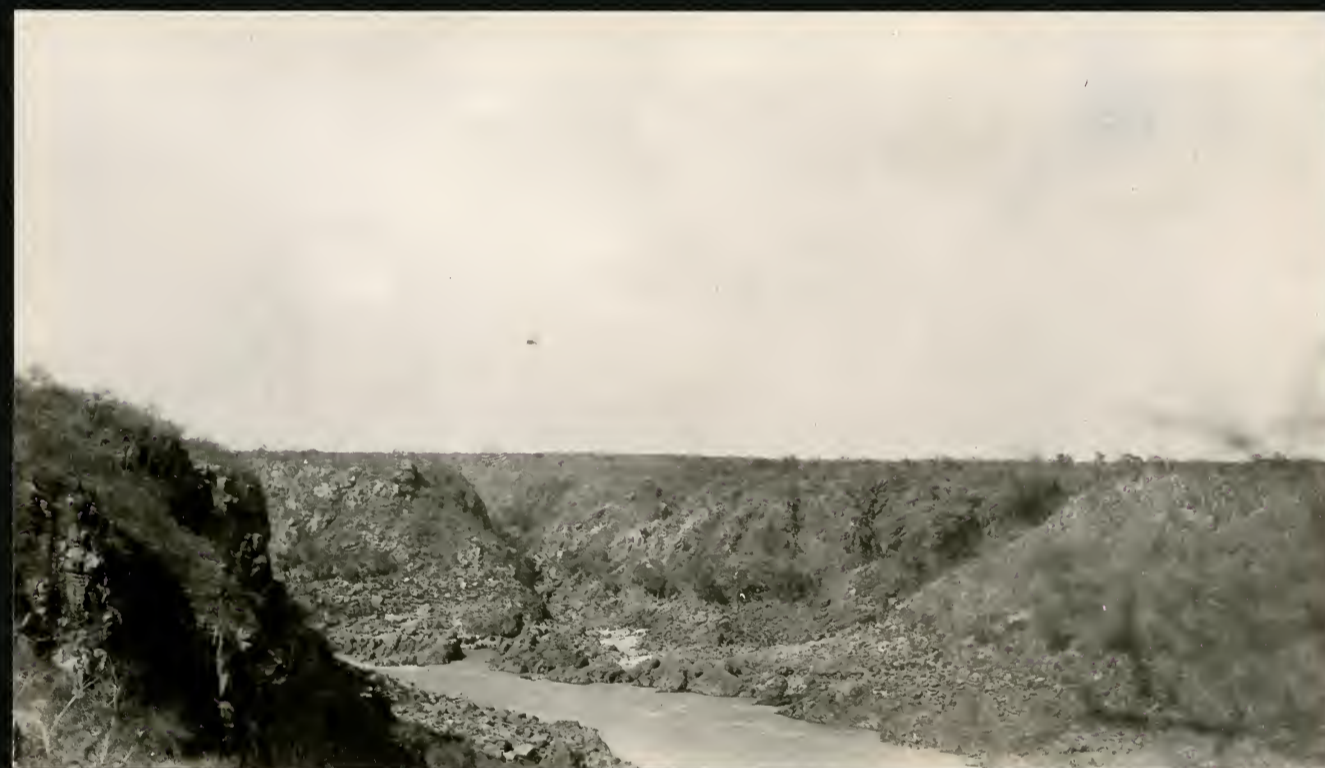
1827. Stream separating power station from mainland.
