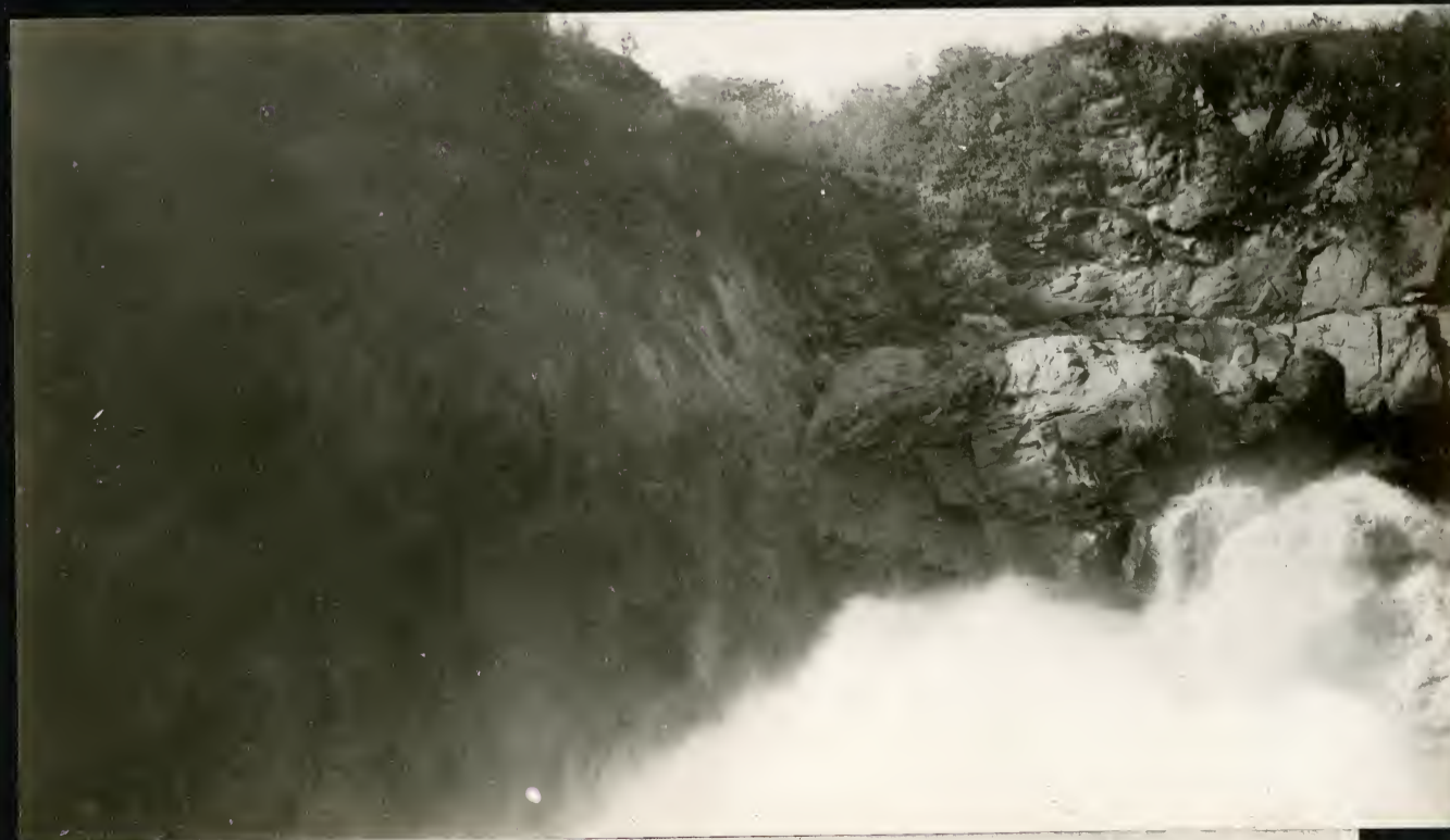
1797. Paulo Affonso falls from turbine station.
