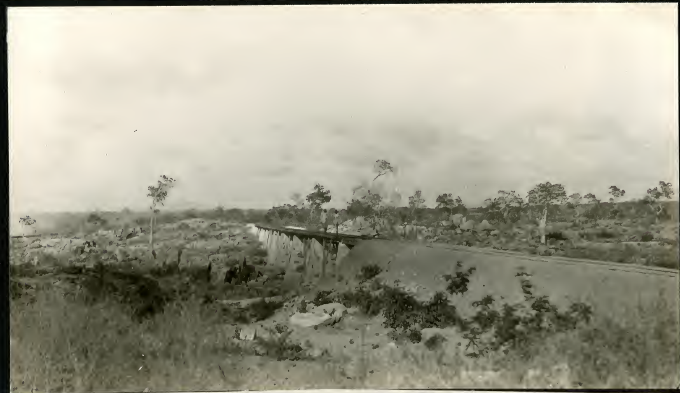
1780. Region of Paulo Affonso falls, Alagoas showing trestle approach to falls.
