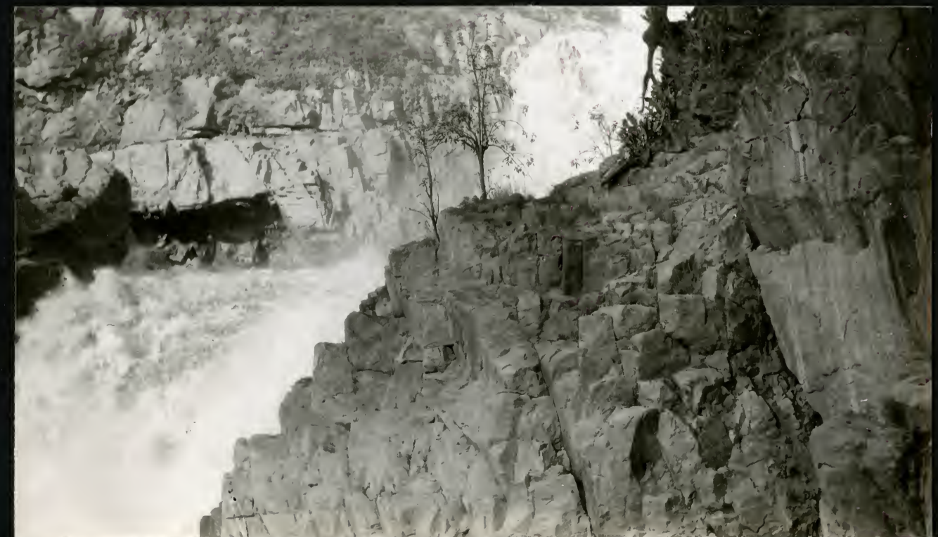
1798. Paulo Affonso falls from turbine station.
