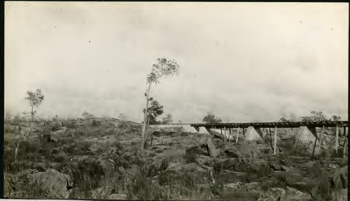
1782. Region of Paulo Affonso falls, Alagoas showing trestle approach to falls.
