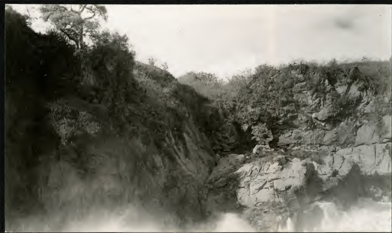
1803. Paulo Affonso falls from turbine station.
