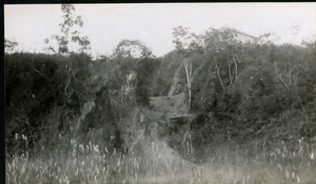
1868. Lavras, showing erosion in red clay hills.
