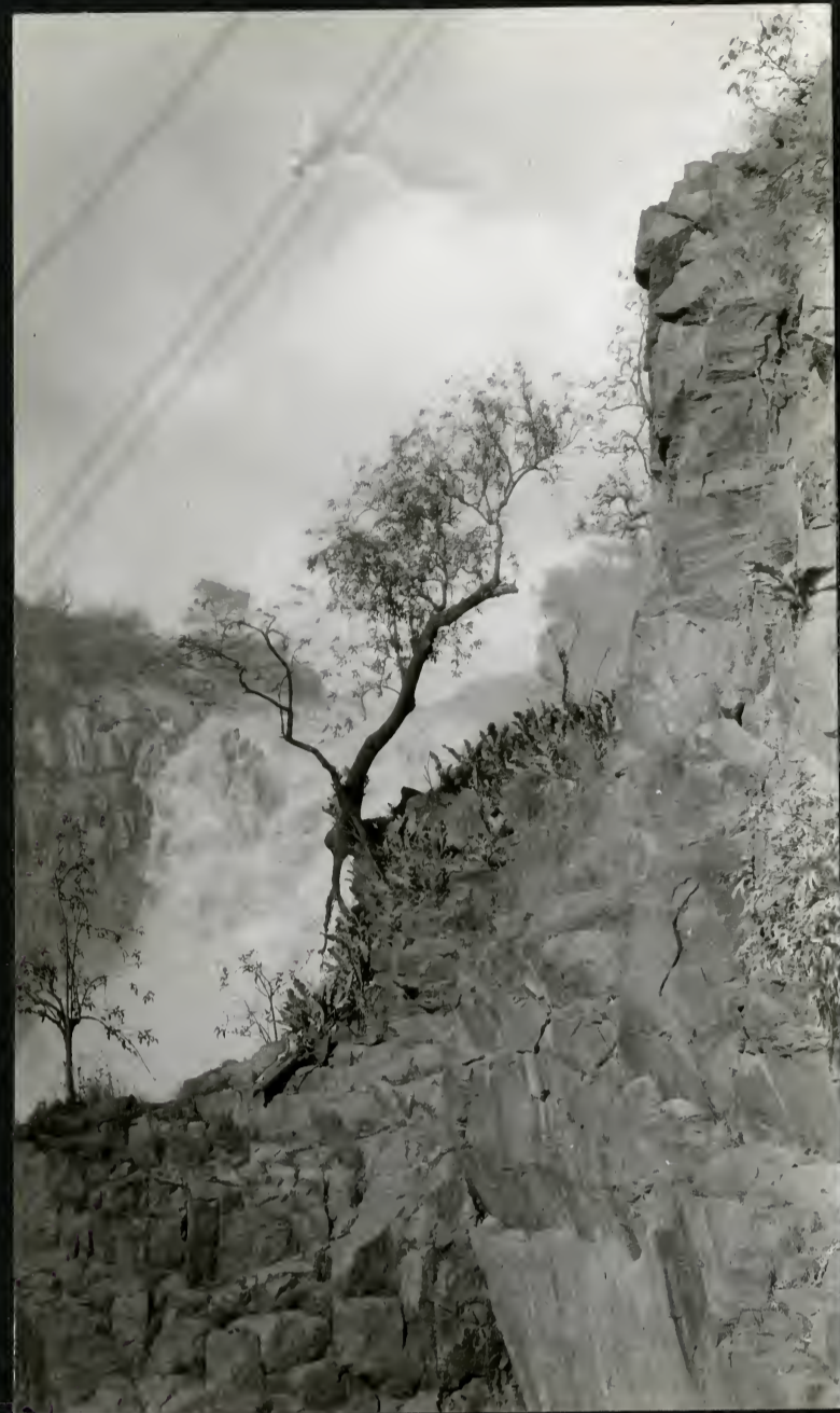
1800. Paulo Affonso falls from turbine station.
