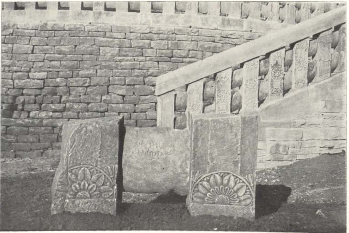
b. STUPA 3: DETAIL VIEW OF GROUND AND STAIRWAY BALUSTRADES.
