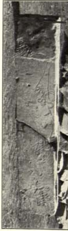
d. OPEN RAILING PILLAR.
