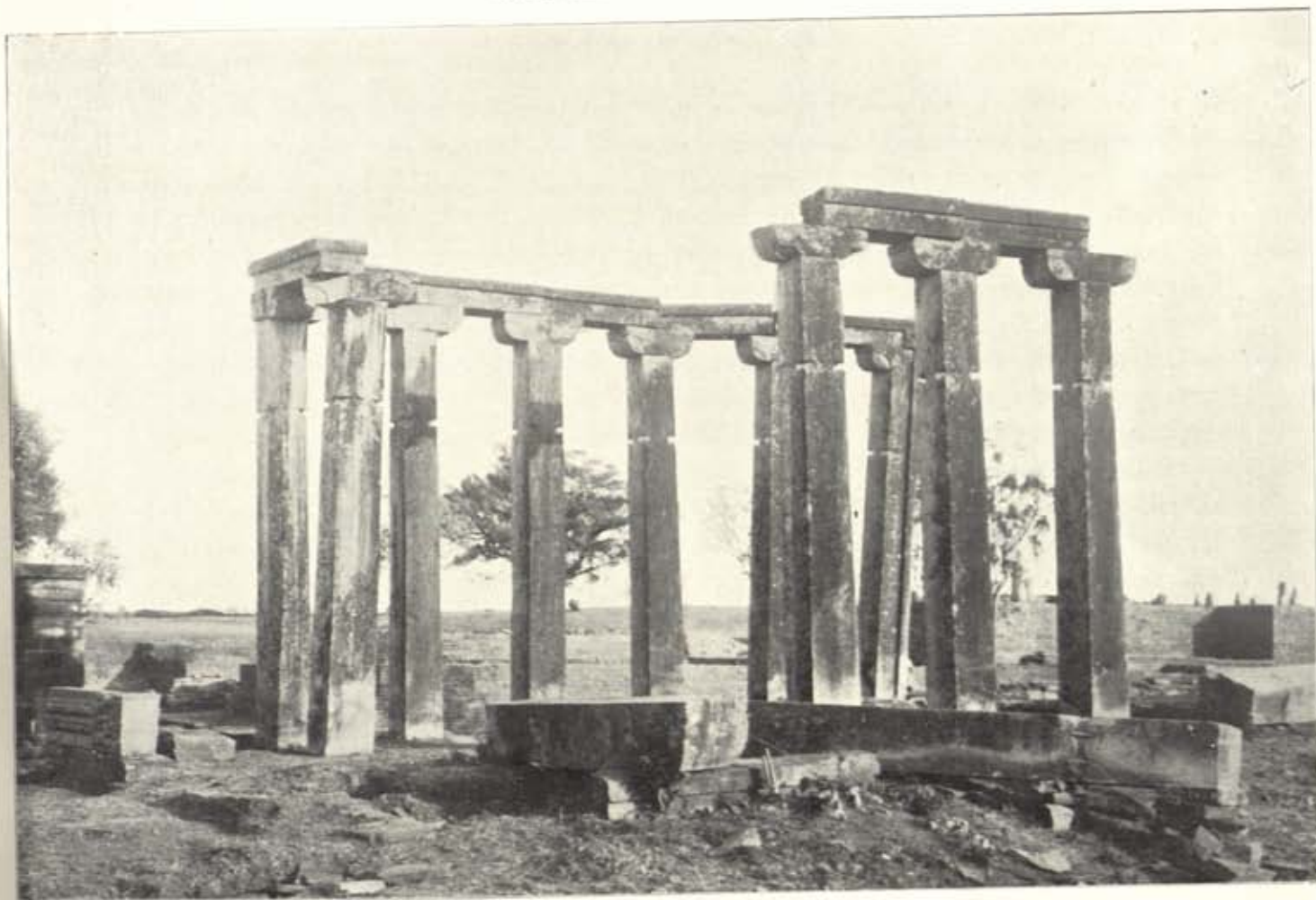
a. TEMPLE 18, FROM NORTH-WEST BEFORE EXCAVATION.
