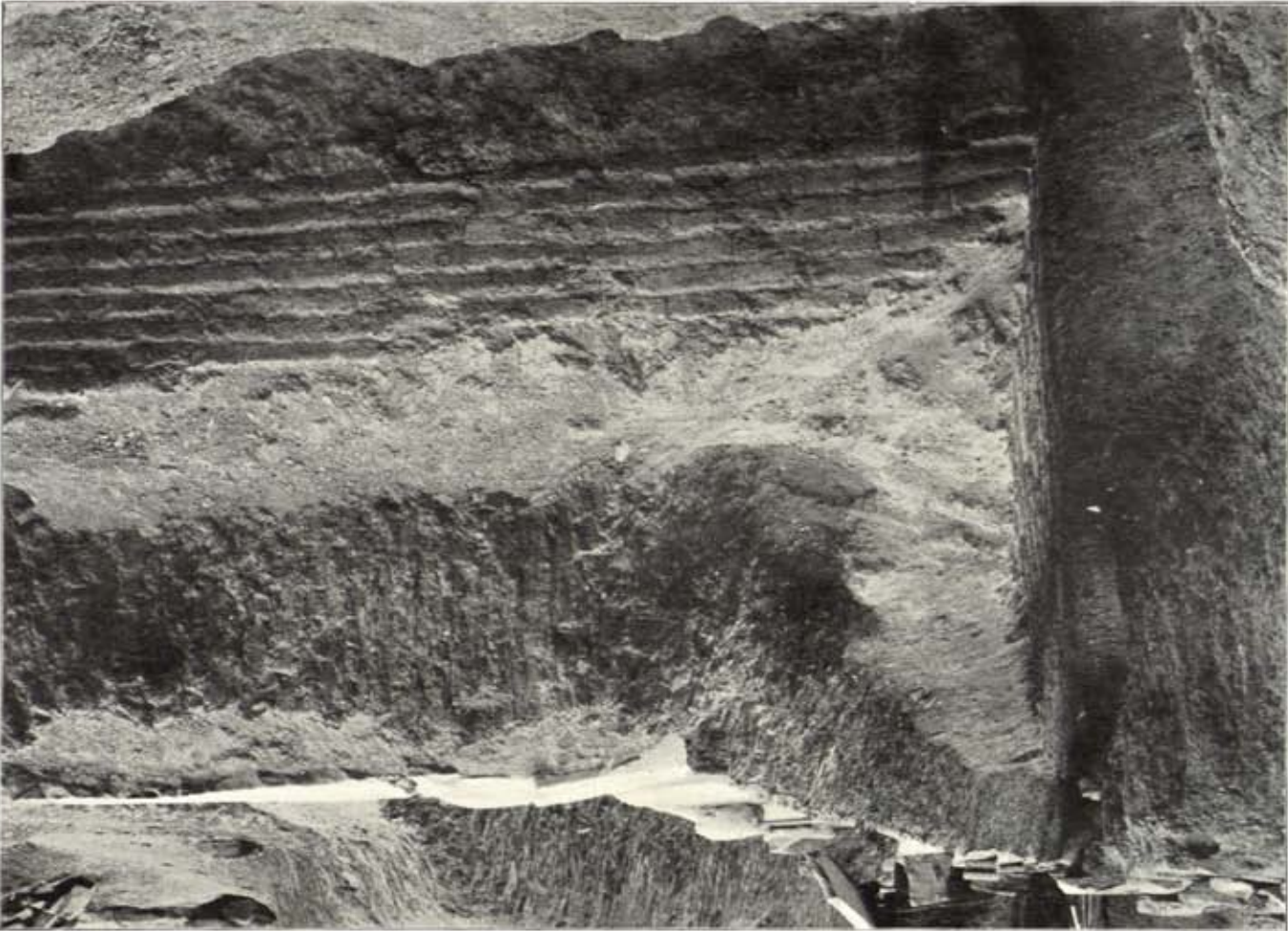
a. VIEW OF BRICK WALL FROM N.-W.
