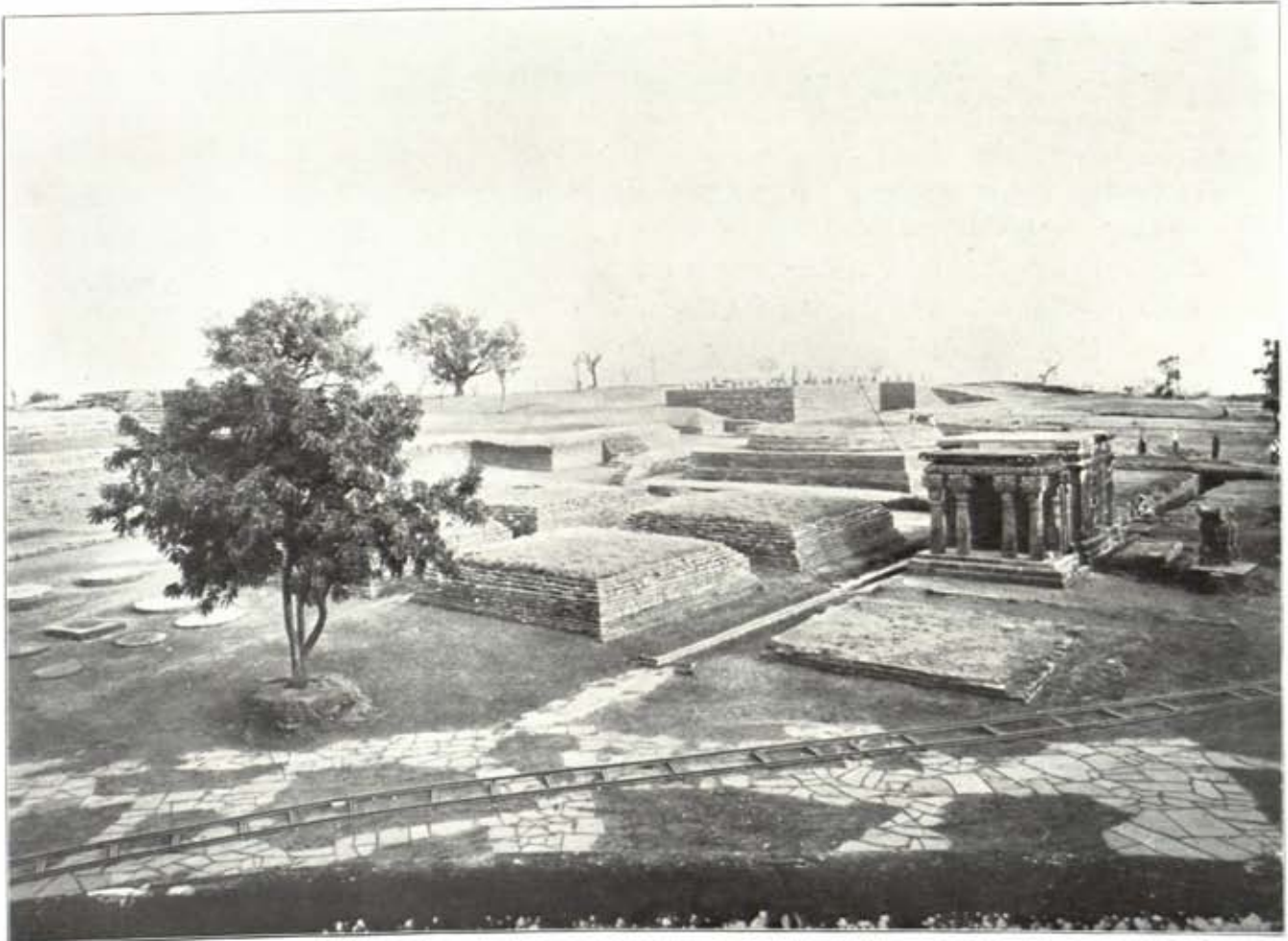
b. TEMPLE 17 AND STUPAS 6, 11, 12, 13 AND 14, FROM NORTH-WEST.
