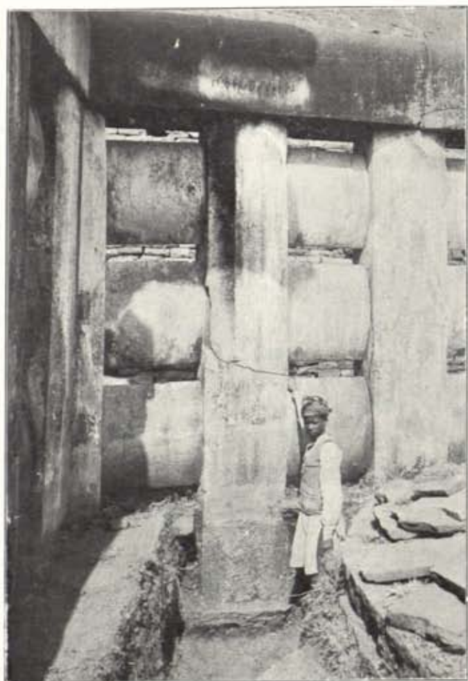
c. STUPA 1: BASE AND FOUNDATIONS OF GROUND BALUSTRADE.
