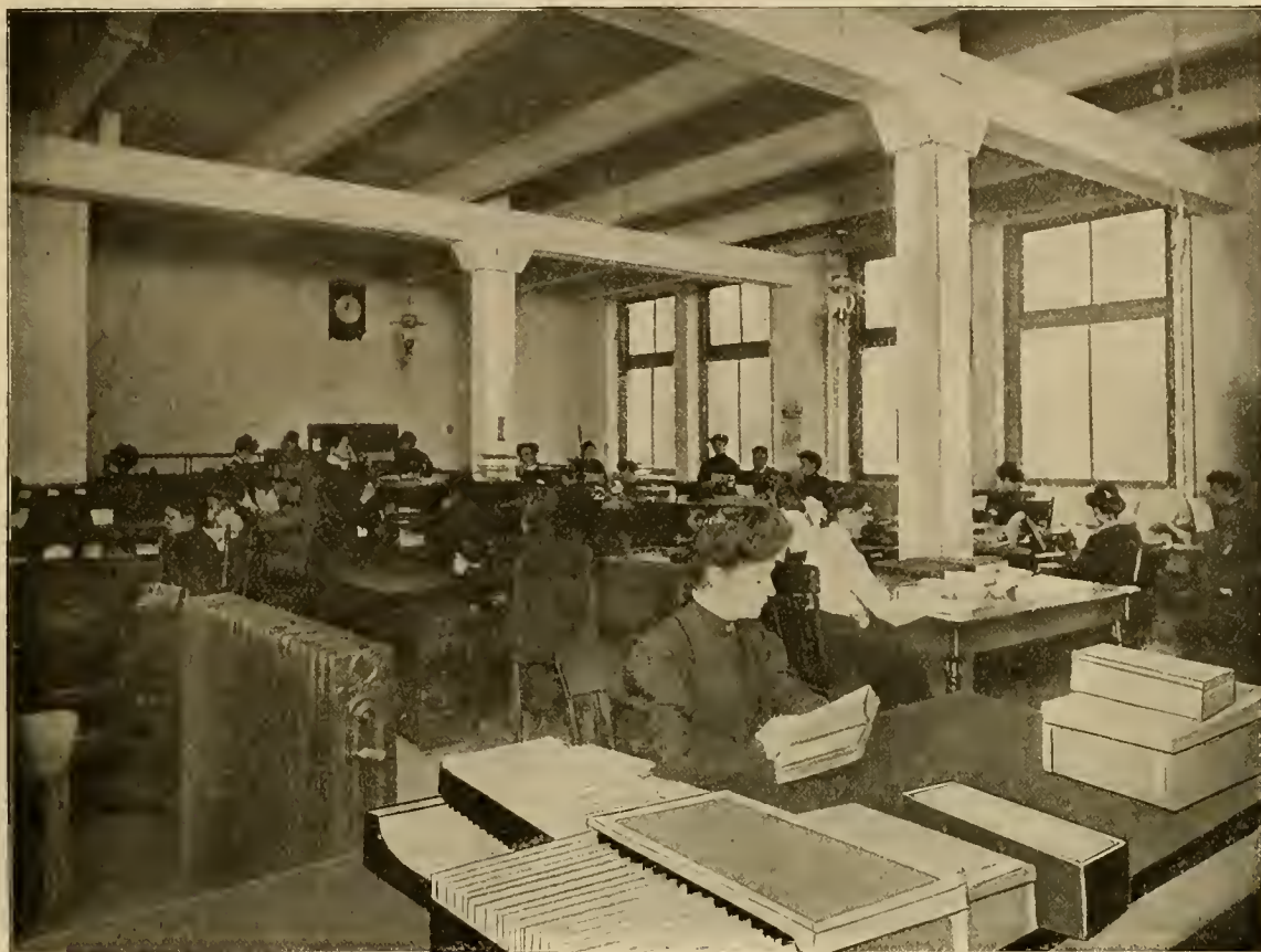
View of Main Office, showing Accounting and Mailing Departments.
