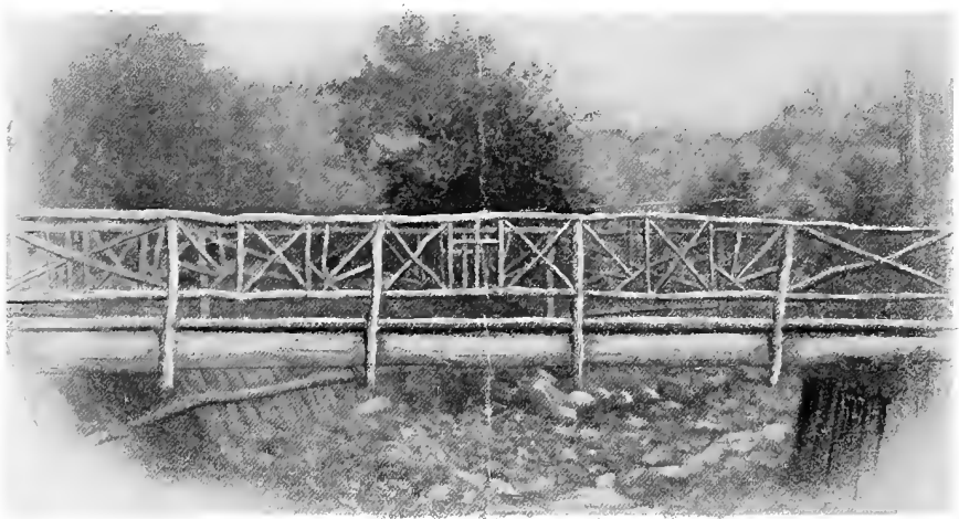
BRIDGE IN RAVINE.
