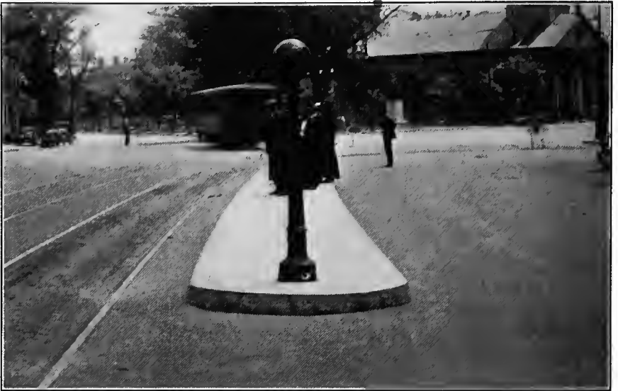
FIG. 35A.—Safety platform at Newark.
