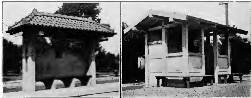
FIG. 96.—Small concrete waiting stations on the lines of the Pacific Electric Railway, Los Angeles, Cal.
