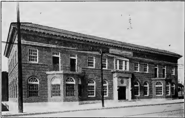
FIG. 118.—Operating depot, Cleveland Railway.
