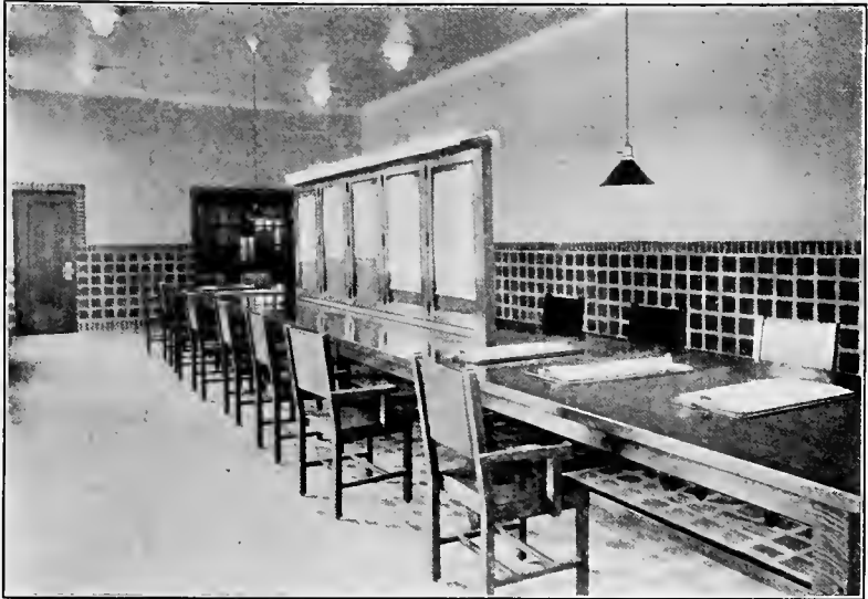
FIG. 119.—Schedule room with metal furniture in Carmen's Depot, Cleveland.
