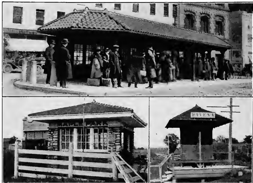
FIG. 95.—Upper view shows waiting station at Hartford, Conn., built by city. Lower views show inclosed and “X” plan stations on Kansas City, Clay County & St. Joseph Railway.
