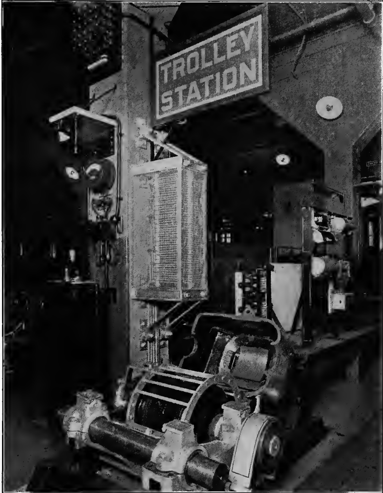
FIG. 116.—Model for showing operation of electrical equipment, Brooklyn Instruction Room.
